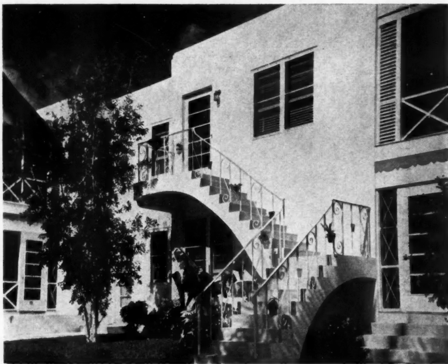
THE office wing can be seen at the far left of this view of the Mooney and Nelson apartments at Fort Lauderdale, Fla. The flower pots attached to the wrought iron railing further add to the ornamental character of the concrete stairs to the second floor apartment.
