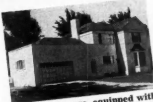
Attached garage, equipped with Ro-Way "Two-Car" Overhead Type Door. Architect, Aldrich & Aldrich, Galesburg, Ill.
