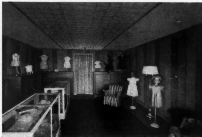
TOTS AND TEENS SHOP, Dallas, Texas, illustrates one of the almost unlimited decorative wall and ceiling effects easily achieved with time-saving Temlok De Luxe. Ceiling is of white panels for superior light-reflection; walls are of 10" wide planks in three colors—all erected with Armstrong's No. 514 Adhesive. Architect: F. J. Woerner, Dallas. General Contractor: W. H. King Construction Co.
