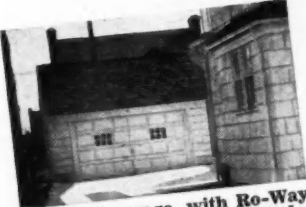
Detached garage, with Ro-Way Overhead Type Door. Toledo, Ohio, residence of Ray Shaffner. Architect, Harold Spooner.
