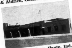
Bus Station, Terre Haute, Ind., using 12 Ro-Way Doors. Miller & Yeager, Terre Haute, Ind., Architect.
