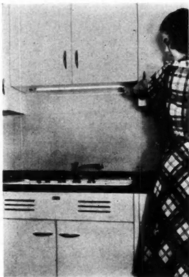
FLUORESCENT light built into underside of kitchen wall cabinet.
