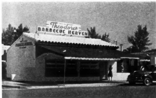
BARBECUE STAND on Alton Road is done in lively, contrasting colors of cream and red.
