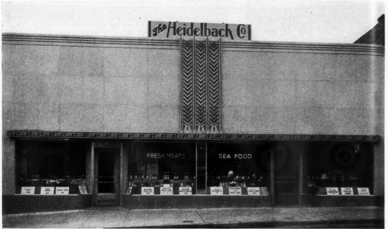
ARCHITECTURAL CONCRETE SLABS in attractive colors feature the front of this meat store in Baltimore, Md., designed by J. R. Kennedy.
