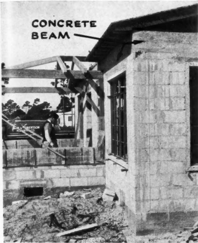
SUBSTANTIAL CONCRETE MASONRY, with 12" "hurricane proof" beam at top of wall, to which rafter plate is bolted.
