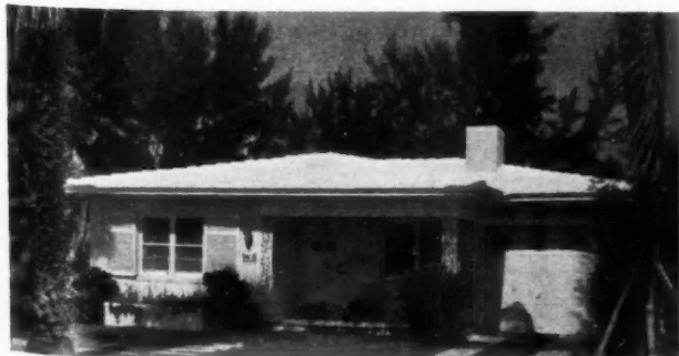
White tile roof, pastel colored walls in Miami house.
