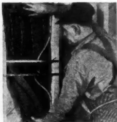
KIMSUL Flexibility Solves Problems KIMSUL comes compressed, is expanded when installed. Can be placed behind electrical outlets and pipes.
