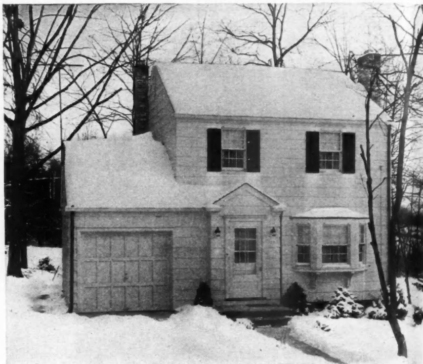
SNOW DIDN'T MELT. Insulation kept the heat inside this typical 5-room Concord Colony house, built by B. V. Zamore.
