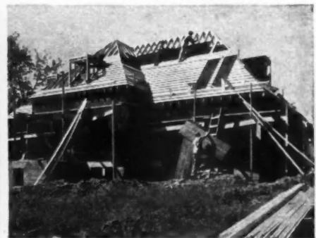
Use Fir-TEX Firkote sheathing on all side walls and roof areas. It takes the place of ordinary sheathing and building paper and provides an unbroken area of insulation. It has greater bracing strength than wood sheathing.
