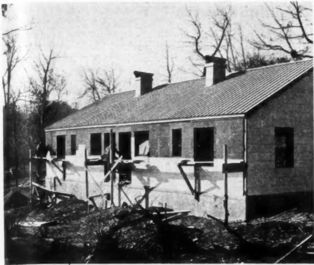
CLOSEUP of two-family Quantico home, showing asbestos cement shingles being applied to insulating board over steel frame.
