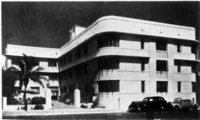
BARBIZON apartment hotel, designed by John and Coulton Skinner; built by O'Neill and Orr.
