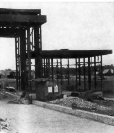
CONSTRUCTION view of framework; note canopy.
