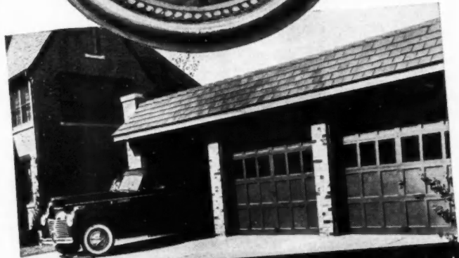
Attractive three-car garage equipped with Ro-Way Overhead Type Garage Doors. Architects, Aldrich & Aldrich, Galesburg, Ill. Contractor, John Dahlberg, Galesburg, Ill.
