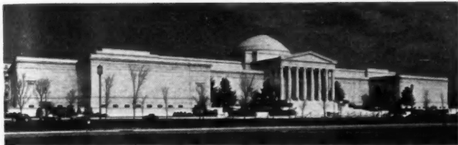
NATIONAL Gallery of Art, gift of the late Andrew W. Mellon. Architect: John Russell Pope (1874-1937); associates, Otto R. Eggers and Daniel Paul Higgins. View shows the Mall front. It stretches for three blocks, is slightly longer than the Capitol and its wings.
