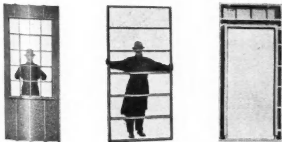
GABLE PANELS are of light steel. At left is wall section with steel window welded in place. In center is interior partition panel, and at right is shown typical door panel with steel frame.
