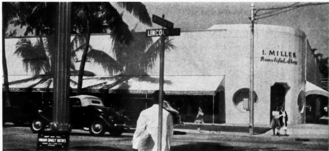
FAMED LINCOLN ROAD in Miami Beach has the most beautifully designed group of shops and stores of any street in the world. Above is the I. Miller store, with typical canopy treatment.
