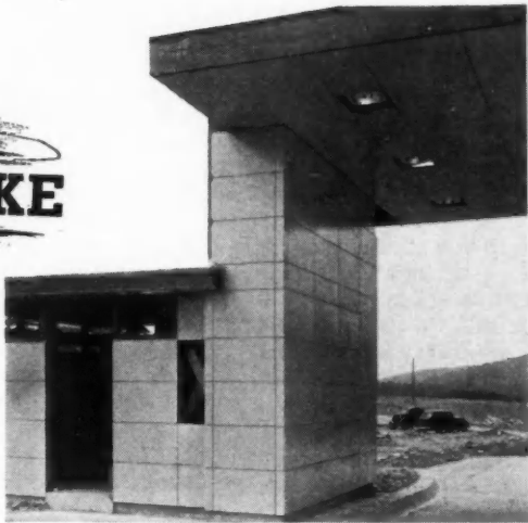
RIGHT: Panels almost cover the frame of this turnpike ticket booth.
