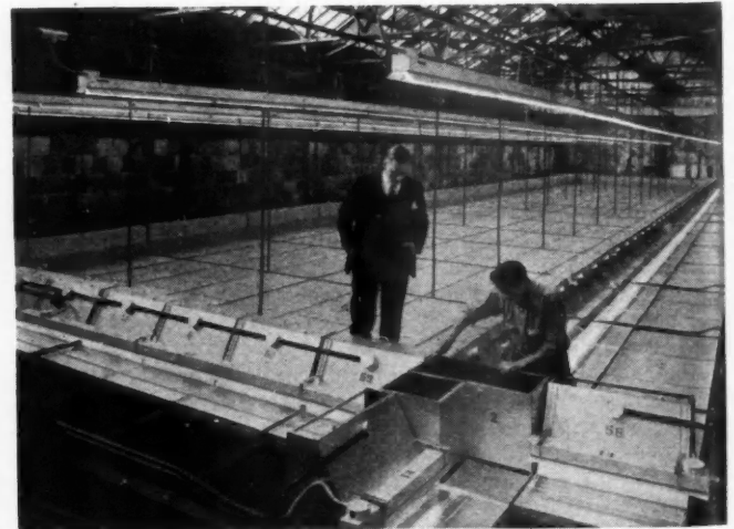
OVERHEAD view of improved lighting being installed in Carnegie gallery.
