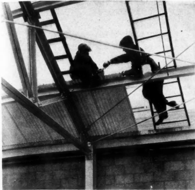
WORKMEN fastening sheets to beam with rustproof bolts.
