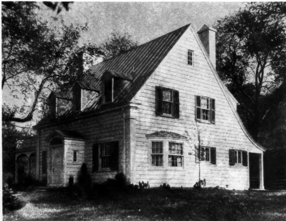
A TERNE roof with standing seams adds to the sweeping effect of the design on this residence of medium size.
