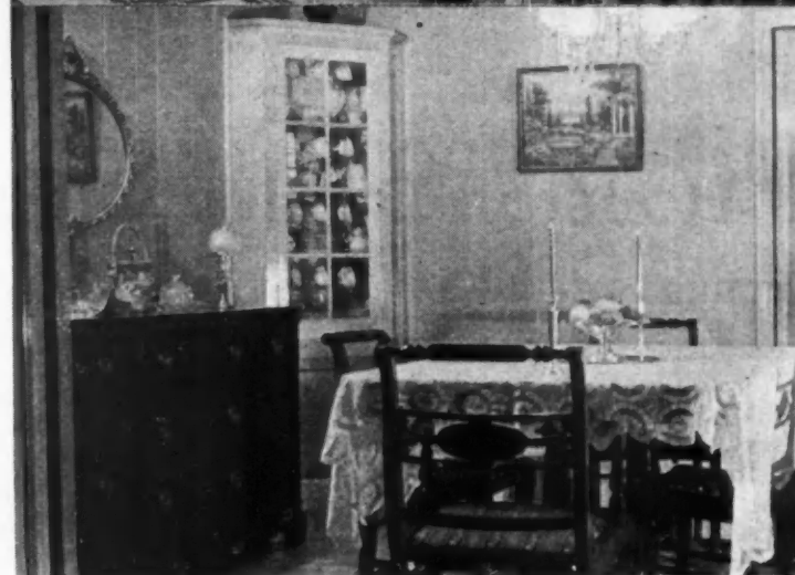
THE dining room, like other rooms of the house, is finished with dry-wall type of construction; in this case, as illustrated at the right, Nu-Wood decorative plank applied vertically was the material selected for the walls.
