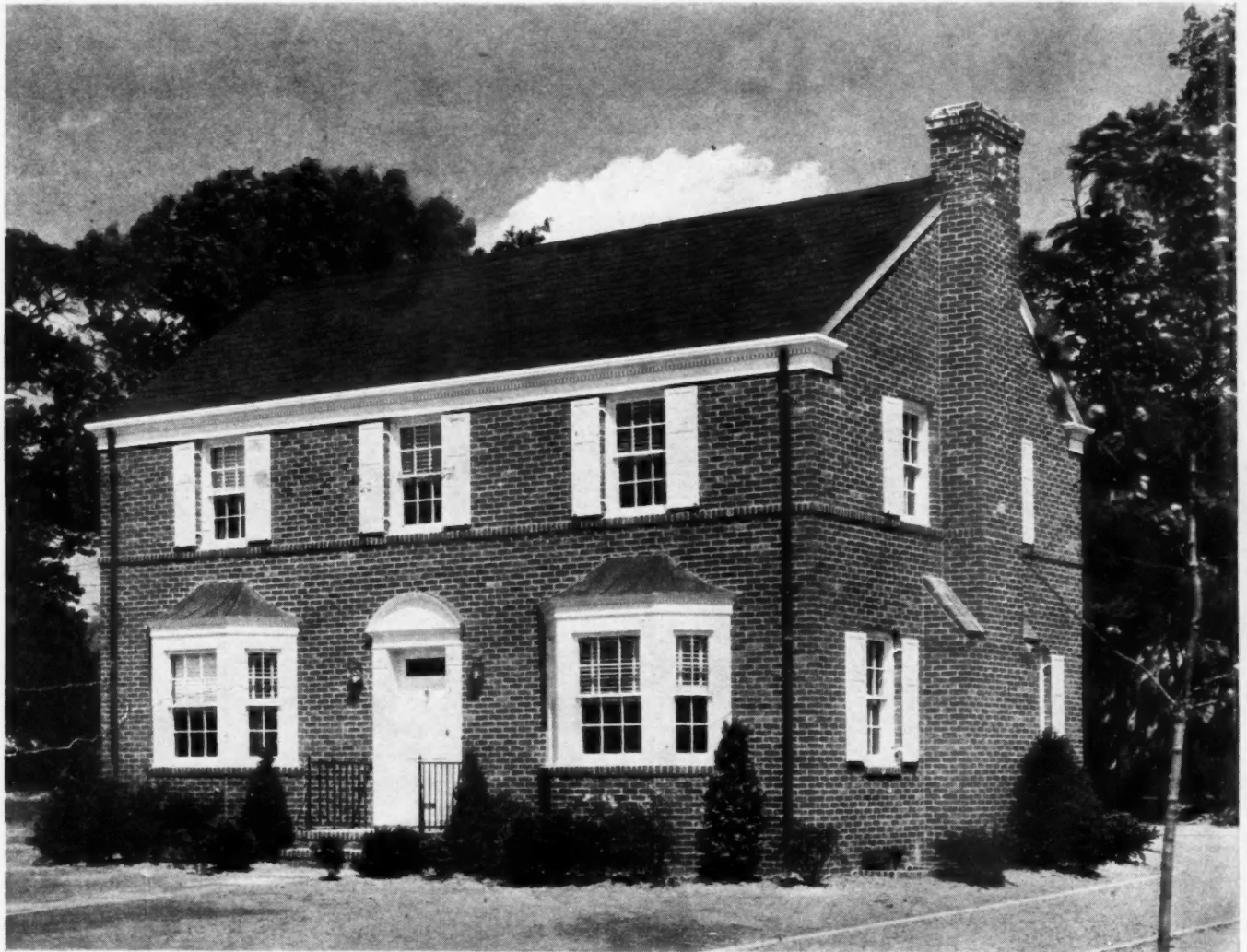
BUILT-UP CORNICE, bay windows with standing-seam copper roofs, and a wrought-iron entrance railing contribute to appeal of this Loft Estates home designed by Walter D. Spelman.
