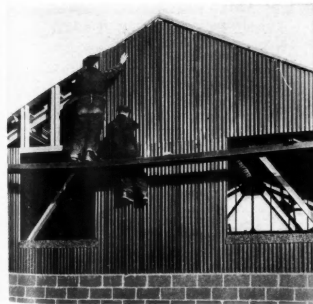
APPLYING side sheets with interlocking edge; note enameled sill.
