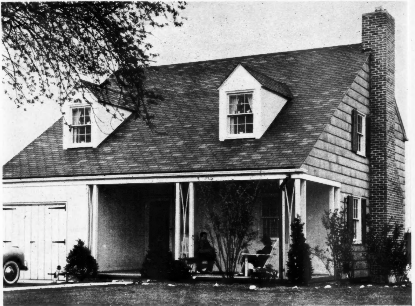
THERE'S FRIENDLY APPEAL in the pleasant front porch and the red cedar shingle exterior. Photos by Hiland Dale Holt.
