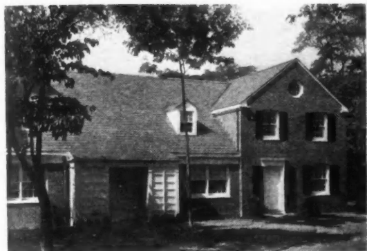
EXTERIOR VIEW of apartments Nos. 20 and 21. Plot plan shows placement of River Glen duplex units. Nos. 2, 3, 6, 7, 12, 16 and 19 are 3 1/2-room units. Nos. 11, 17 and 18 are 4 1/2-room units. Nos. 1, 4, 5, 8, 9, 14 and 21 are same as 4 1/2-room plan above except being corner units, windows are at side; no fireplace.
