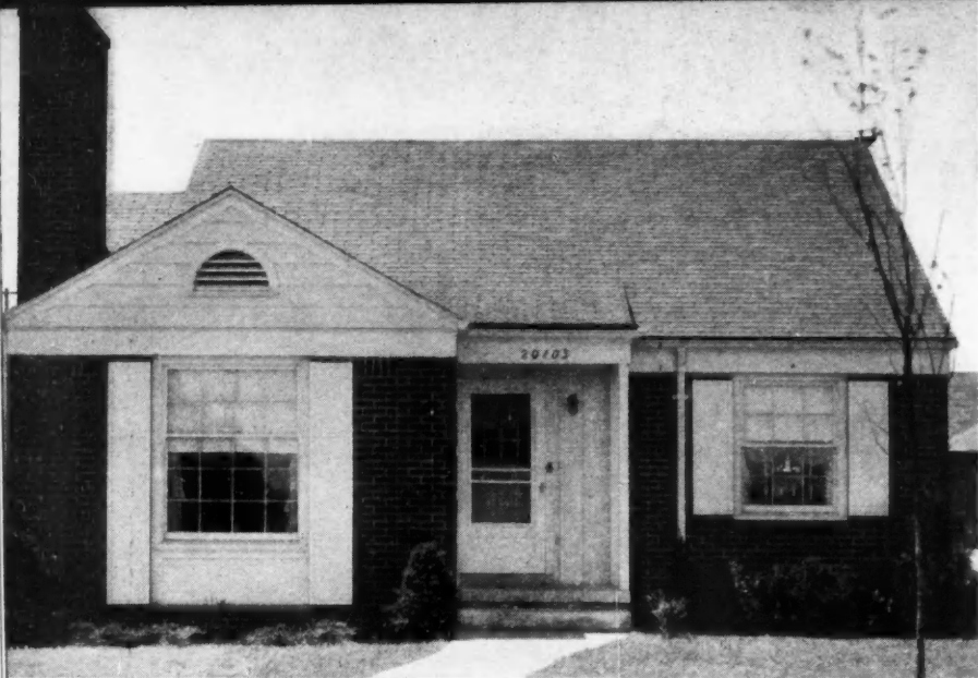
BUILT by Milo F. Gonser, this compact five-room design has through hall circulation, vanity in tiled bath, Celotex insulation, corner cabinets in octagonal dining room, Curtis millwork, Niagara gas conditioner, and Sonneborn floor finish.
