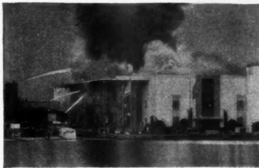
EXT-DFFPA PROVES FIRE RESISTANCE The California State Building on Treasure Island was a veritable furnace on Aug. 26. But the exterior walls, built of 7/16" outdoor plywood covered with fire resistant paint, remained standing in spite of terrific heat inside and water pressure outside. Mr. C. E. Seage, Assistant Executive Officer of the Exposition, wrote "The performance of the plywood was most gratifying. In many instances the fire on the inside burned away heavy studding leaving the plywood to withstand vertical loads. The conclusions are that had not the plywood with the aid of the paint resisted the fire in the manner it did, it is possible the spread of the fire would have been much greater."
