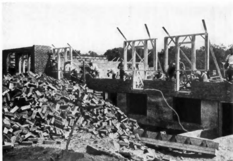
STREAMLINED ORGANIZATION of workers gets job done quickly.
