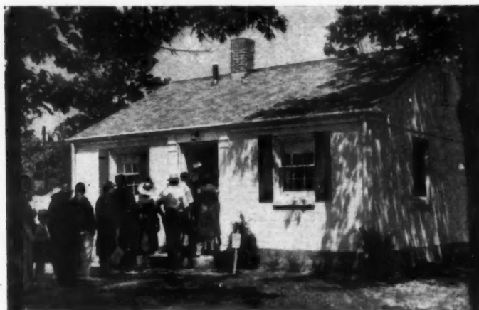
This attractive small concrete house is one of forty built in industrial Chicopee, Mass., by H. D. Fiedler and Associates. Prices, with lot, ranged from $2,800 to $3,500.
