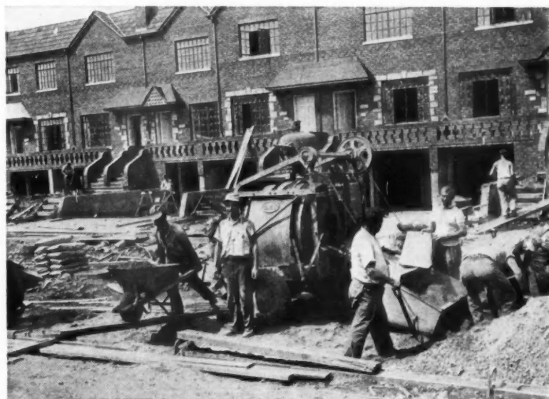
CONCRETE WORKERS rush Trump houses to early completion.
