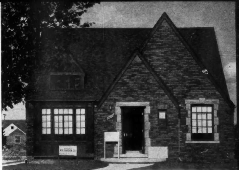
W. R. GORDON & Co., Detroit designers and builders, erected this home in the 1940 Builders Association project and featured unfinished second floor with gas-fired conditioning unit large enough to heat it when completed. Besides this flexibility, it has Rezo doors, Standard fixtures, Savutime hot water control, breakfast bay, Air-O-Cel in side walls and rock wool in ceiling, tile kitchen.
