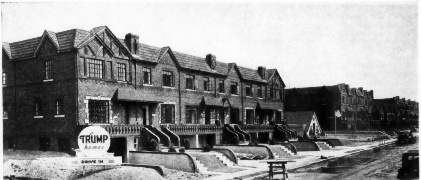
ROW of Trump homes in Flatbush, Brooklyn, where Trump built and sold 125 houses in three months last summer in $6,000-$7,000 class. Floor plan is shown on page 26.
