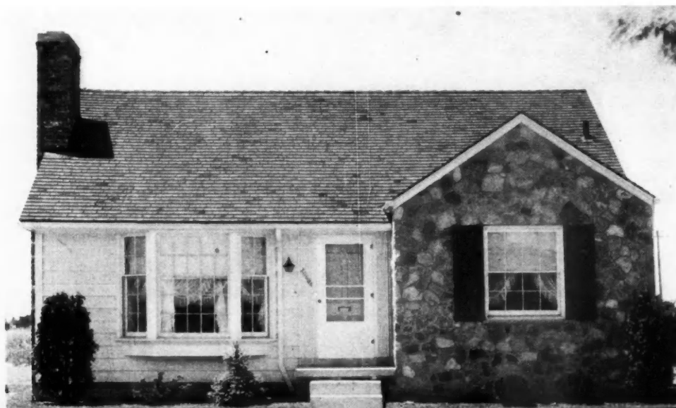
THIS trim little four-room design by Builder A. L. Doenges has five-room efficiency, with eating space either in the kitchen corner or living bay. As one of the houses in the Builders Association of Metropolitan Detroit demonstration project, its charm had wide appeal. It featured automatic gas heat, recreation room, built-in wardrobes and tile bath.
