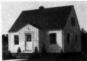
CLEVELAND —One of 16 houses in which George M. Colcher, Cleveland builder, has used Fenestra Package Windows. 27 more planned. Colcher says, "They are money-savers and sales-winners."
