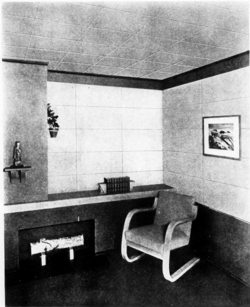
THE ATTRACTIVE finish of this insulation board, combined with invisible nailing of the wall and ceiling panels, results in a number of new decorative possibilities for this economical surfacing material.
