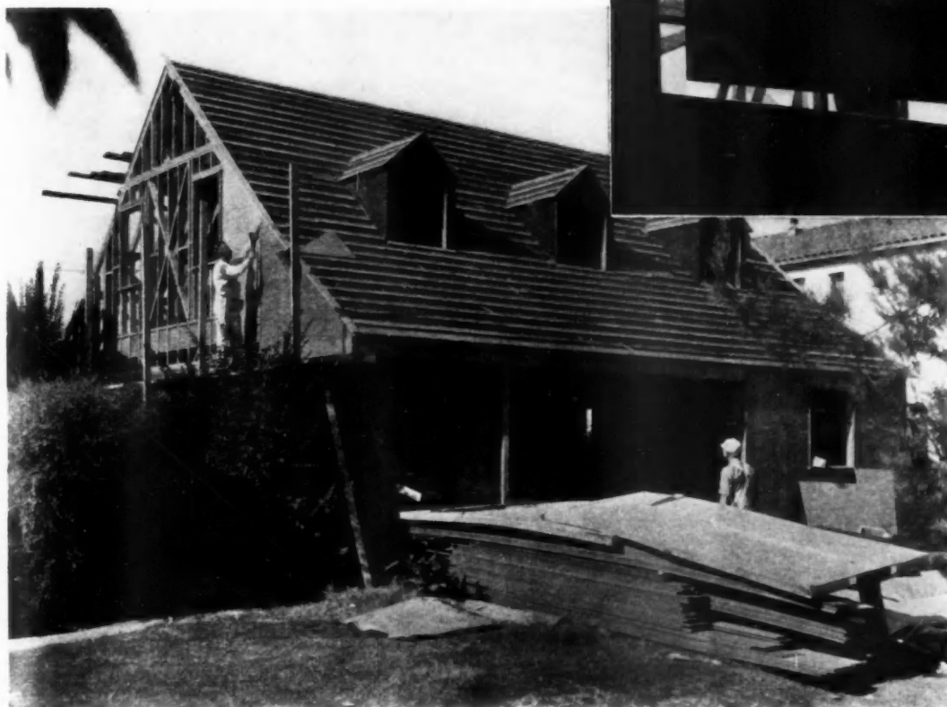
HORIZONTAL sheathing units 2' x 8' make shiplap joints on long edges.
