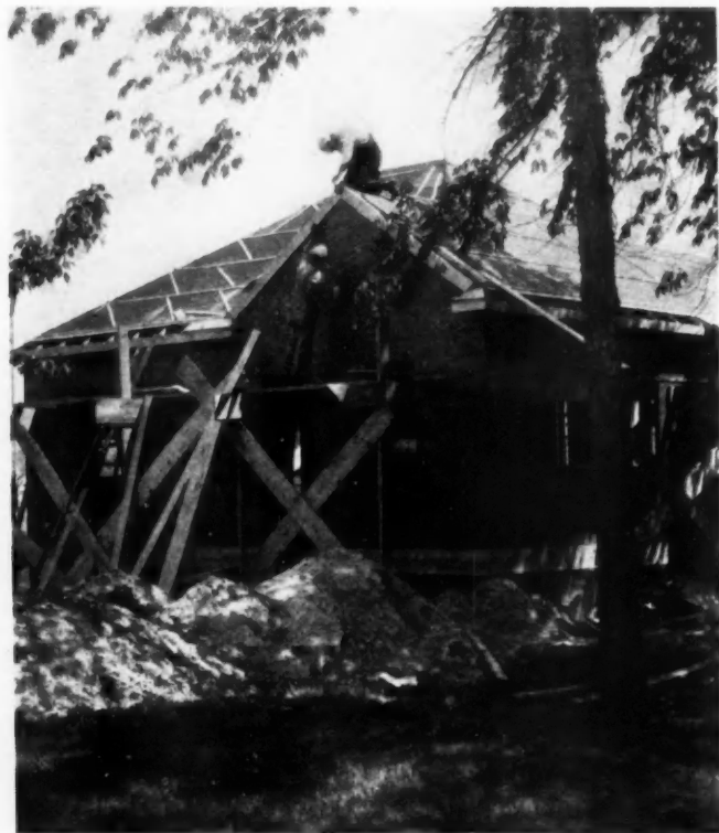
INSULATION board is popular for sheathing homes, assuring both stiffness and warmth.
