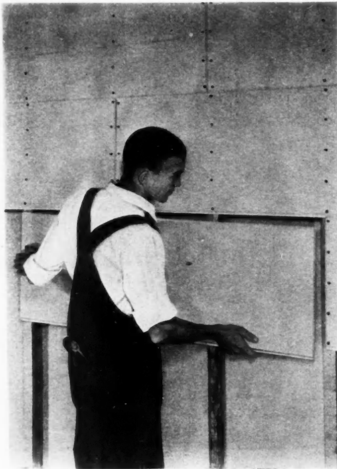
PLASTERING lath of insulation board goes on fast and is economical of plaster.
