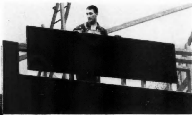
HORIZONTAL sheathing units 2' x 8' make shiplap joints on long edges.
