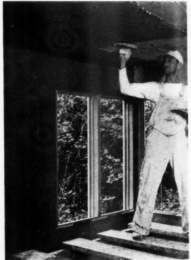
PLASTERING lath of insulation board goes on fast and is economical of plaster.
