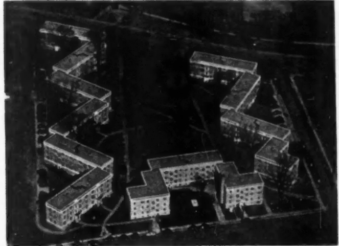
AERIAL VIEW of Cameron Court apartments, showing how 147 units are grouped about court.
