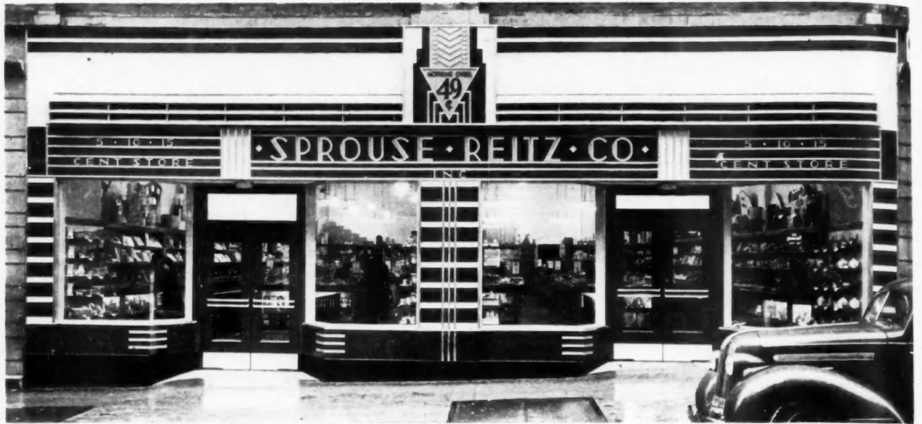
THE WELL LIGHTED INTERIOR is the window display of this Portland, Ore., store. Front is Micarta and Carrara glass, aluminum trimmed.
