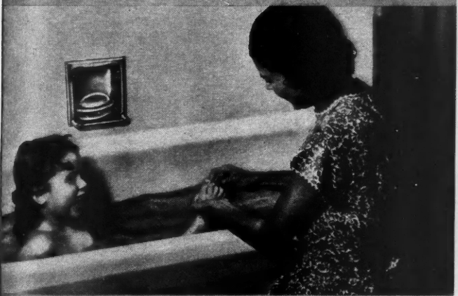
WATER-HEATING . . . Instant hot water any time at the turn of a faucet. Improved insulation cuts down fuel consumption.
