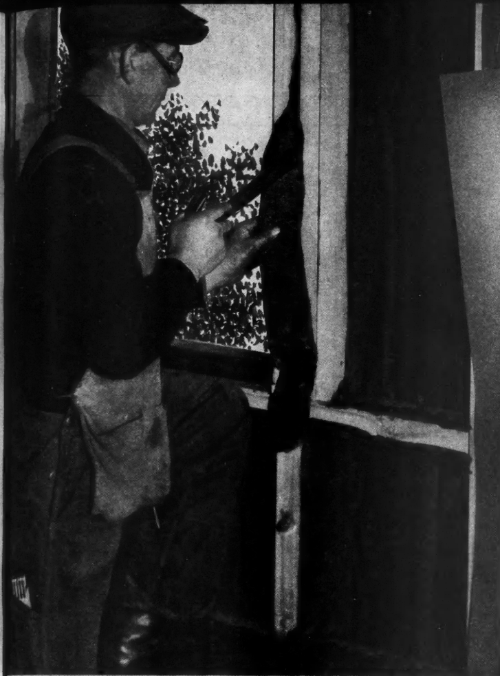
As these pictures show, Kimsul is an all-purpose insulation material. It can be installed with equal ease in standard and odd sized wall openings. Short ends are valuable as caulking around window and door frames. For attic floors, simply lay expanded blankets between joists and fasten them down at the ends. It also makes possible an efficient and practical method of insulating sloping roofs.
