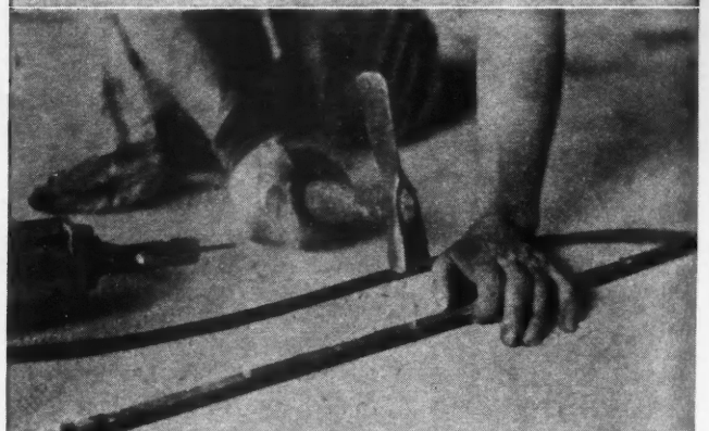
MARTIN-CONROY'S method of attaching steel stud to concrete floor and ceiling in Ten Eyck Homes.
