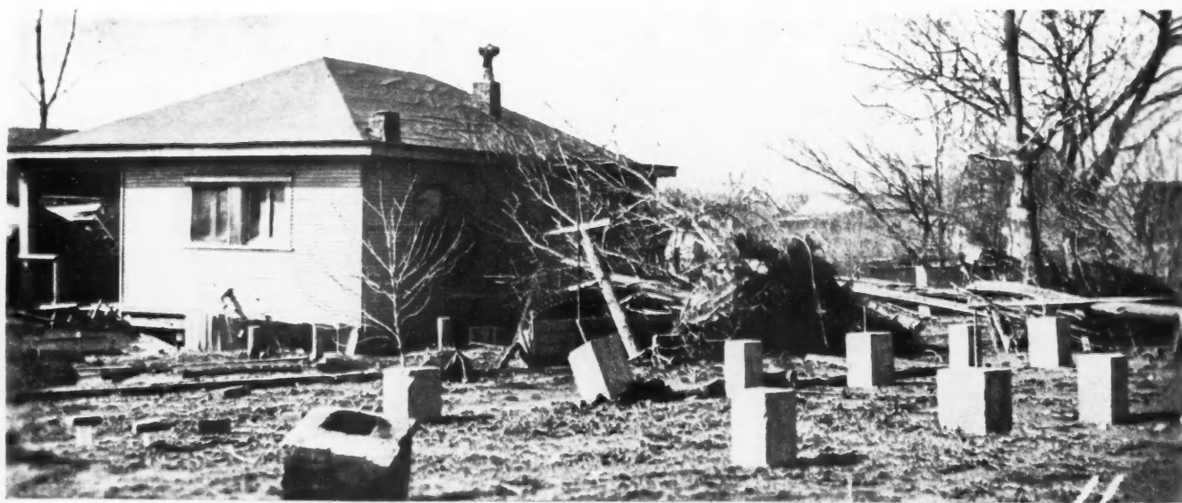
THE BUOYANT effect of submersion caused this house to rise off its concrete piers and float away. The straight anchor rods imbedded in the piers without washers and nuts proved insufficient anchorage.
