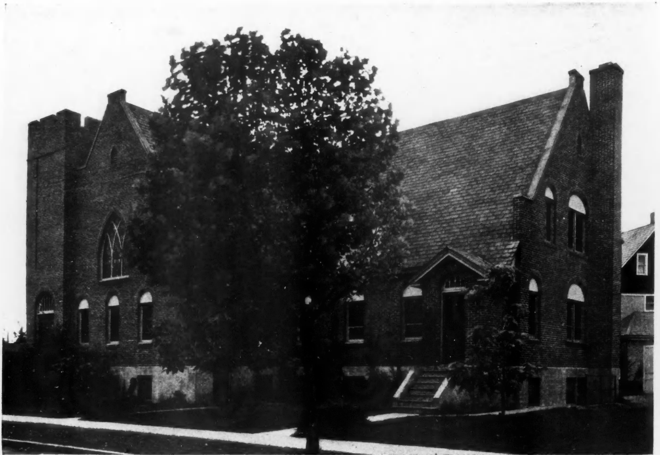
AFTER —Here is the Glens Falls Church after the exterior had been covered with 2" split brick laid over Steeltex. The ladies of the church were so pleased with the transformation that they told practically everybody in town about it, which was fine advertising.
