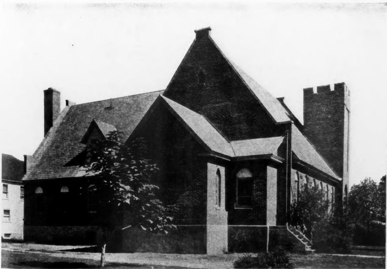
AFTER —Rear view of the church after modernizing, showing how beautifully the new brick surface improved its looks. A slight addition was made to the choir loft projection but very few other structural changes were required. Cost was under $3,000.
