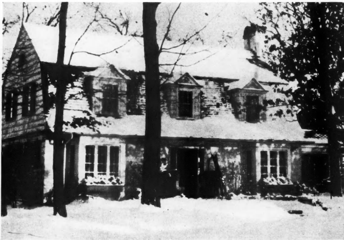
RESIDENCE of Professor G. L. Larson, Madison, Wis., on which novel insulation calculations described in this article were made.
