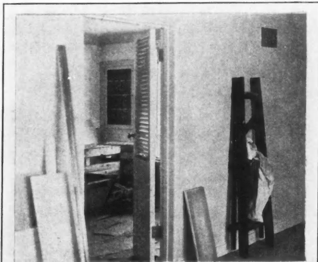
FIG. 2 DOOR LEADING FROM LIVING ROOM TO DINING ROOM. MANY OF THE DOORS ARE OF THIS HANDSOME LOUVRE TYPE. DELIVERY GRILLE AT UPPER RIGHT.
