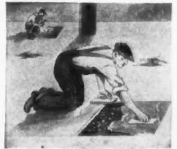
WORKMAN installing Rockflux floor.
