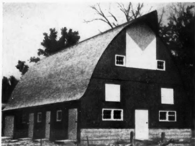
GOTHIC roof barn near Jewell, Ia., designed by the Author whose shop fabricated curved rafters were furnished through the O. I. Kleaveland Lumber Co. Below, frame work before enclosure.
