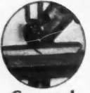
Compound Miter Sawing
