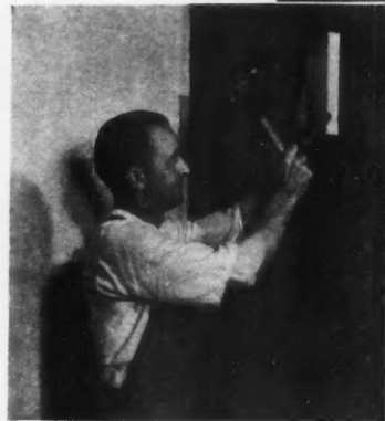
LEFT: Adhesive is applied to both lap joints as well as back and bonded by pressure of hammer blows.
