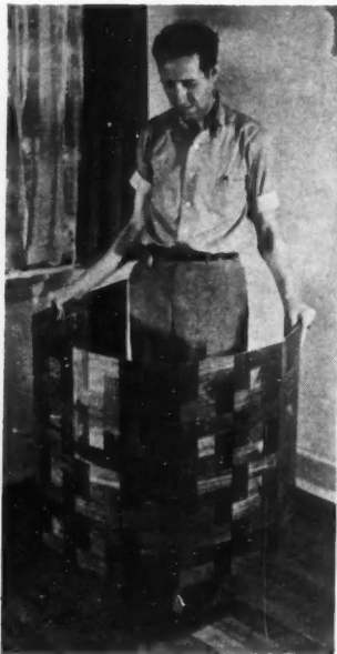
LEFT: Workman holding Parkay floor section shows flexibility of material. Right: Finished floor quickly laid in mastic is ready for use.
