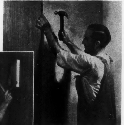
LEFT: Adhesive is applied to both lap joints as well as back and bonded by pressure of hammer blows.
