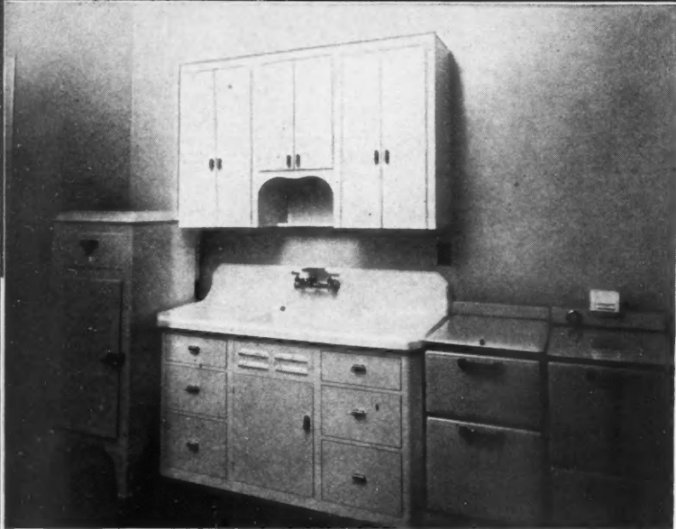
ABOVE: Top view shows typical kitchen which before remodeling was large and badly outmoded. The completely modernized kitchens have steel cabinets over the sinks and built into the canvased walls, latest mechanical equipment and linoleum covered floors.
