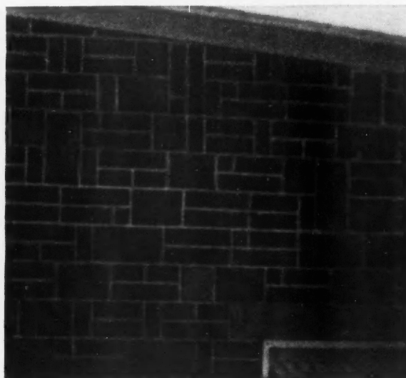
WALL of random ashlar concrete blocks after pointing.
