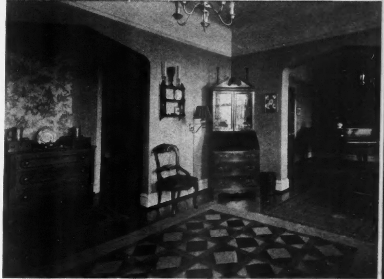
ABOVE: The somber old living rooms have given way to light, open areas. Long, dark hallways were eliminated to add size to other rooms; seven and nine room units were divided into two apartments; closet space was increased where storage was inadequate.
