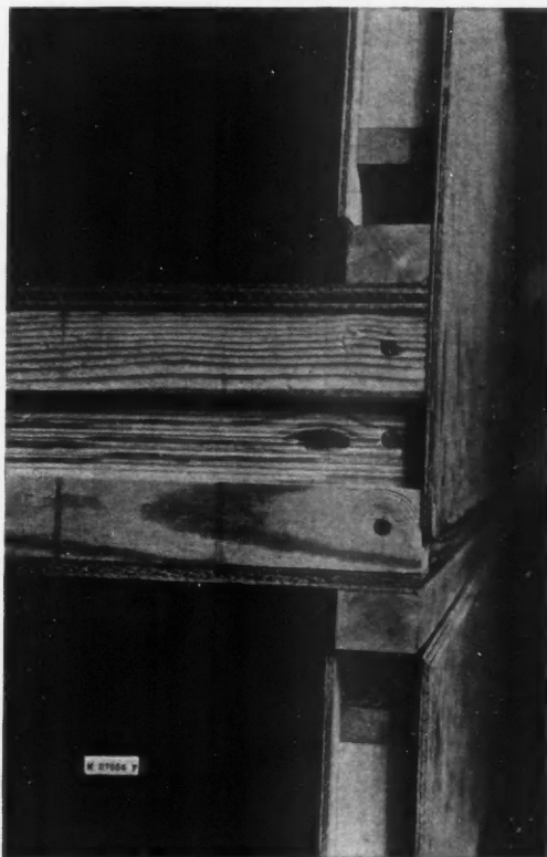
FIG. 10—Portions of first story wall panel, floor panel and second story wall panel which are slightly separated to show how parts fit together.
