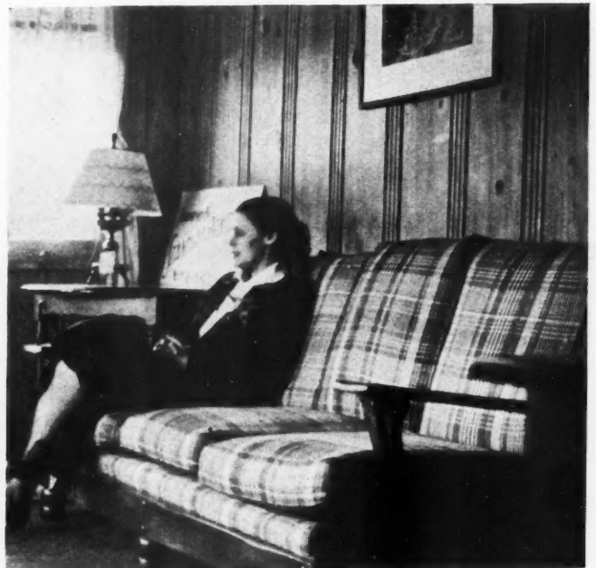
INTERIOR of "Stud-bat" cottage showing smooth surface walls (like detail No. 10) produced by 12-inch vertical boards panel fitted into grooved 2x4 studs set flat. This feature is being patented by Klicka Lumber Co.
