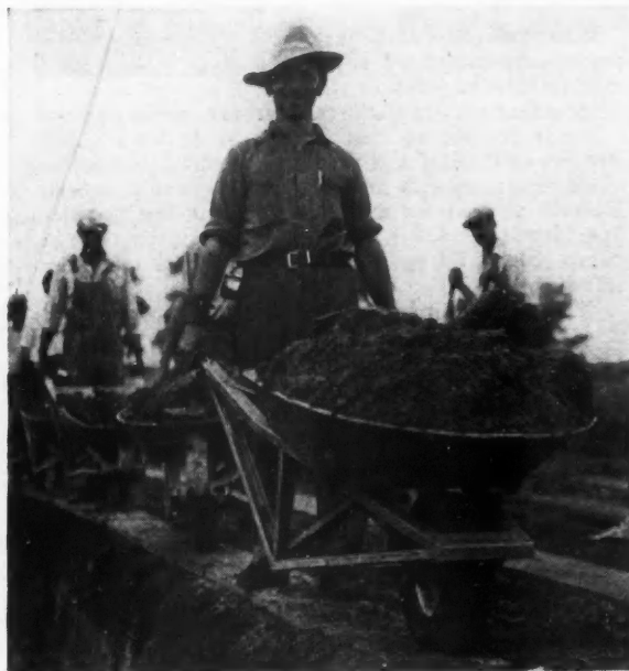
WORKMEN using light weight, pneumatic tired wheelbarrows.
