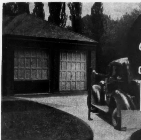
Key operated switch located conveniently on the driveway post enables operator to open and close door without leaving the car.
