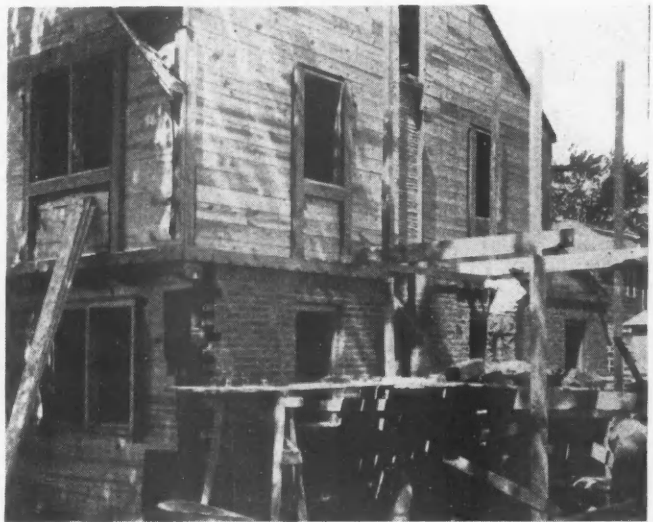
HALF TIMBER WORK , water table, windows are copper flashed; face brick skilfully laid over waterproof paper, the work carefully done.
