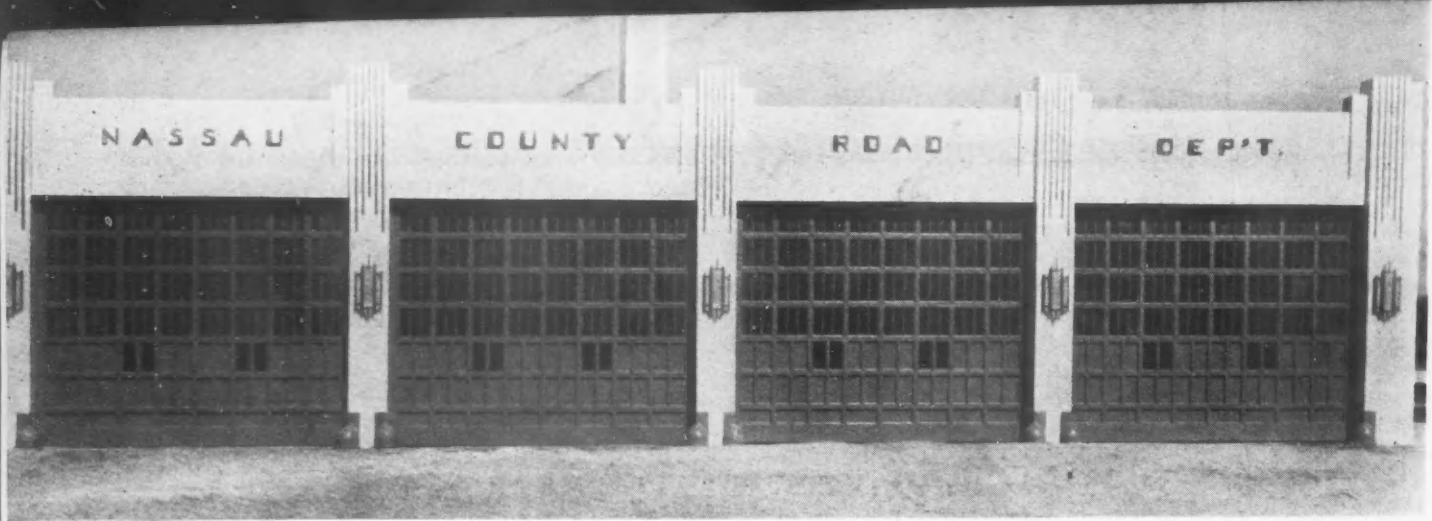
ABOVE: The County Garage on Baldwin Road, South Hempstead, N.Y., has large steel Float-Over doors using the equipment of Cornell Iron Works, Inc. Below: Key operated switch seen at left controls the Rol-Top Kinnear doors from the drivers' seat.
