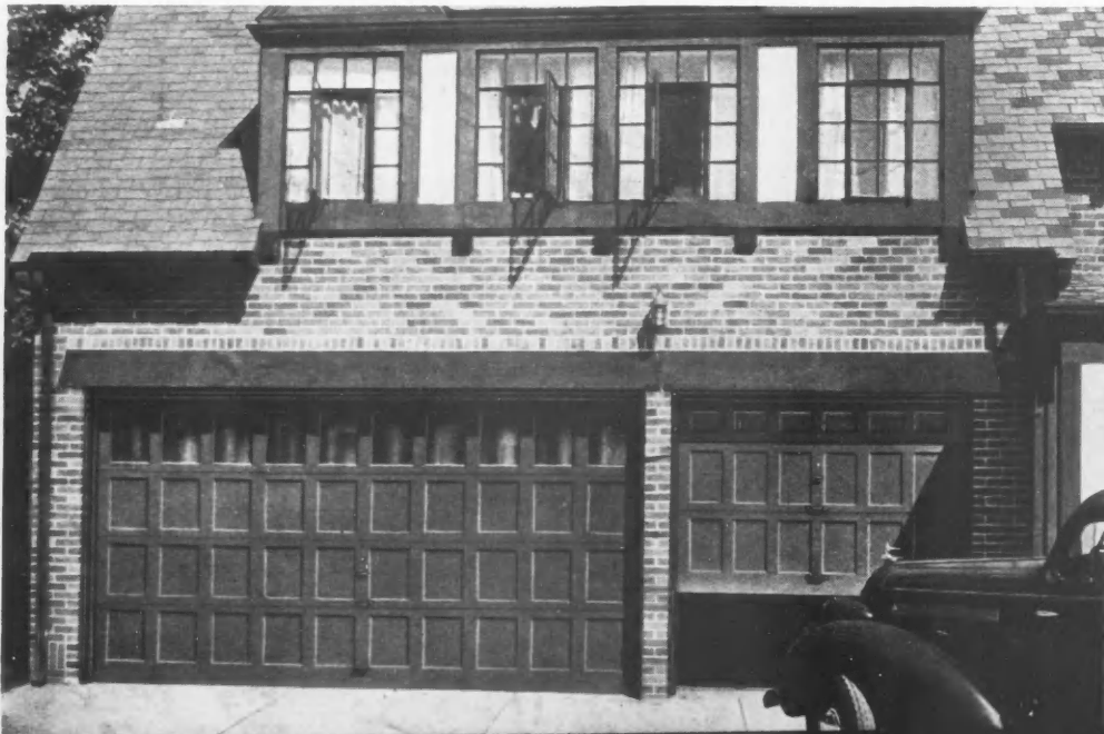
LEFT: Originally designed for a three-car garage, lack of space for three separate doors was overcome by using one double and a small door with Overhead Door Corp. equipment. Owner, Wellington Burt; architect, L. J. Sarvis; contractor, D. L. Murray; location of job, Battle Creek, Michigan.
