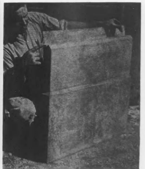
LEFT: Drawings show cornice treatment of poured concrete and details of veneering (the standard soldier course as shown in drawing was replaced by a precast base on this particular job). BELOW: Brick veneer hung on steel strip fasteners ready for mortar; Contractor Mullins points to nailing strip in foundation slab.
