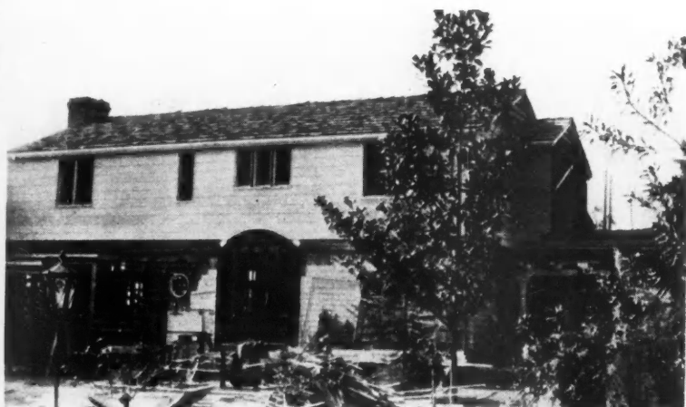
ABOVE: Front view of the house during alterations showing additions and new roof line after the dormers were removed. BELOW is the same view when completed; the garage is seen at the right.
