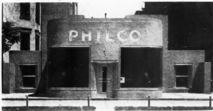
ABOVE: The Philco Bungalow before remodeling; set back from the sidewalk, it had little attention value from the street. LEFT: New unit with large and attractive display windows. BELOW: Plan and sectional drawings of modern addition.
