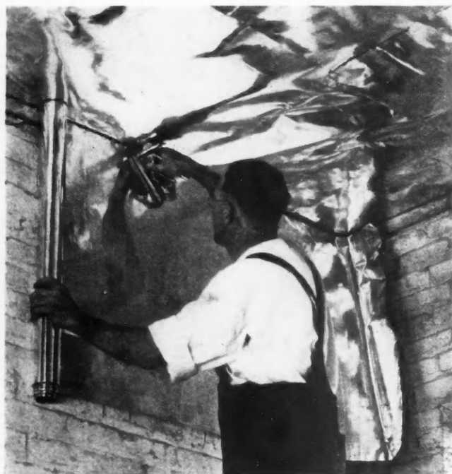
Applying insulation with new tacker
