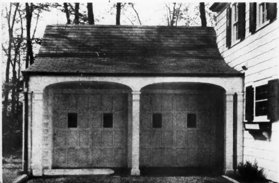
TO LEFT: Covered approach from house to these garage doors is appreciated in rainy weather, besides giving architectural character to this motor wing. Cornell Float-Over doors were used by the builder, Masten & Wicht, of Oceanside, L.I.
