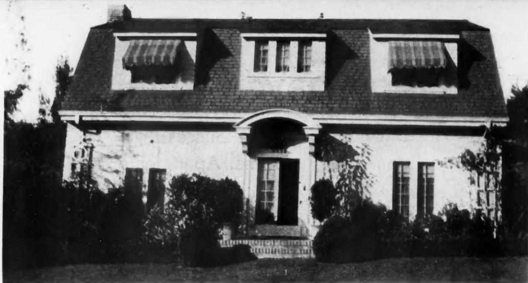
THE DUTCH COLONIAL at Altadena, Calif., as it appeared before remodeling; too small and unattractive to the owners although location and surroundings were satisfactory.
