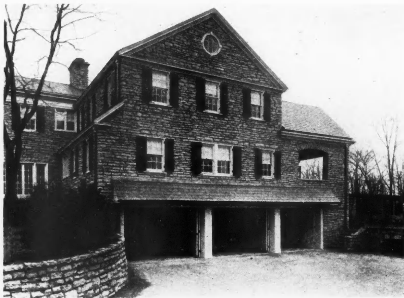
ABOVE: Three-section motor room in basement of large Louisville home; C. A. Zeigler of Philadelphia, Architect; Palmer Graham of Louisville, Contractor; Richards-Wilcox Slidetite garage door hardware used.
