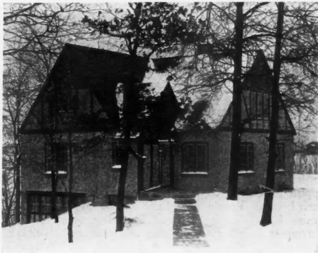
THE STUCCO HOME above is substantial and attractive, and typical of the types of homes that will be built when FHA financing becomes available. It has a large living room, 5 bedrooms, and cost $10,000 in Kalamazoo, Mich.
