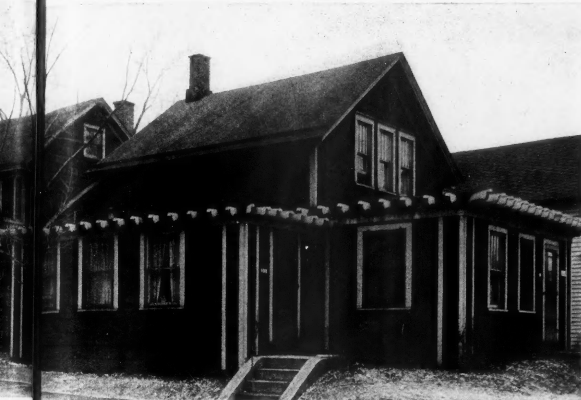
FROM a $20 a month cottage, this property was developed into the row of apartments pictured at left, now fully rented and earning 14% on the investment. Shutts and Morrison, Erie, Pa., are the architects.
