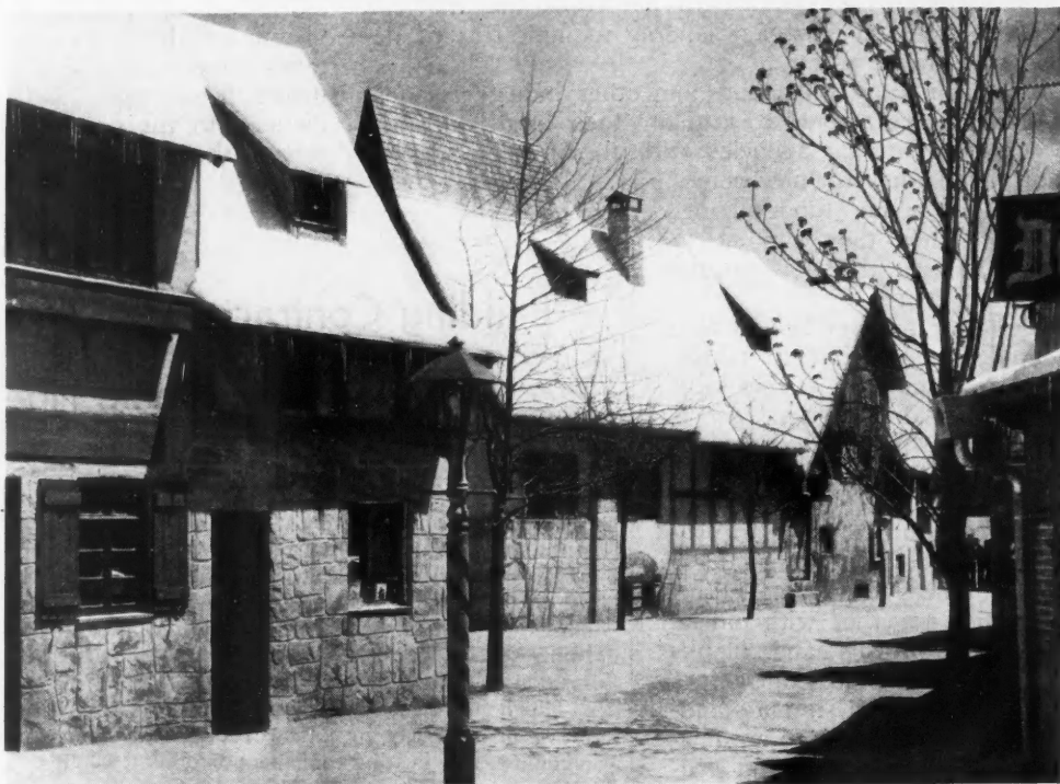
THE SWISS VILLAGE at Chicago's 1934 World's Fair shown above features the Swiss mountain chalet. The reproduction of mountains is most realistic. Daniel H. Burnham, Architect; Kaiser-Dussett, Builders.
