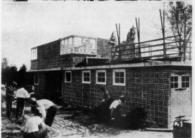
Three steps in the procedure of casting brick panels and assembling them into a building as developed by Architect Henry K. Holsman.
