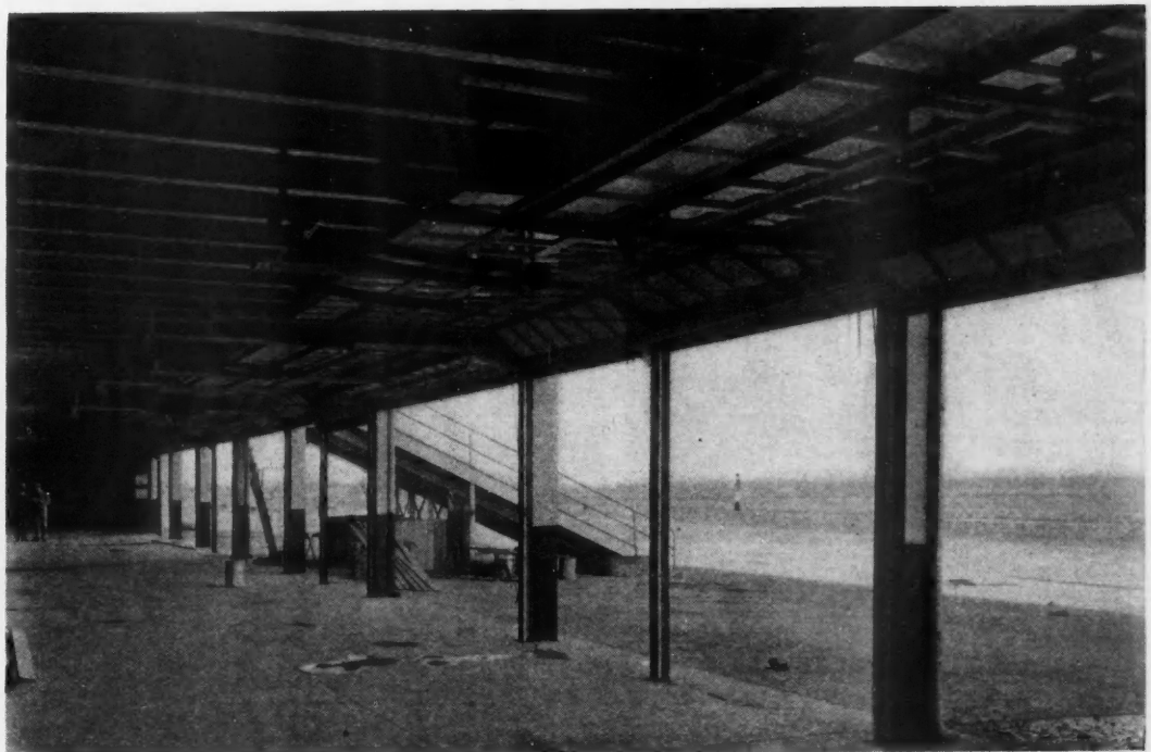
COURT OF THE WORLD in the Ford Exposition Building showing the chromium metal columns built from plywood faced with thin sheets of chromium plated copper.
