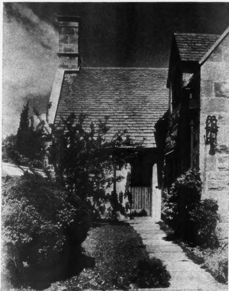
THIS COTTAGE, designed by Roger H. Bullard, New York architect, was awarded the Gold Medal in the Better Homes in America Small House Architectural Competition. Limestone walls, slate roof, stock design casements are used.
