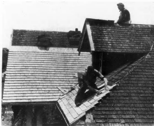
New shingles over old roofs are proving entirely satisfactory
