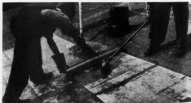
COPPER ASPHALT ROOFING —a new product consisting of thin, flexible layer of copper with heavy asphalt saturated fabric back. Comes in rolls, is durable, strong, easy to apply.
