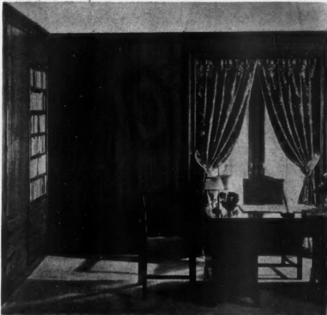
WOOD SURFACED GYPSUM BOARD —light weight gypsum board panels used in library. Wood-like surface resembles mahogany, and provides inexpensive paneled effect.
