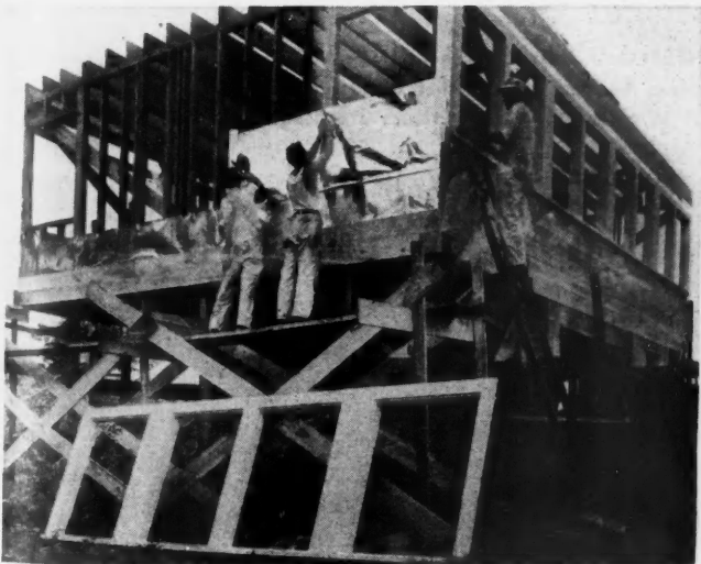
ALUMINUM FOIL SHEATHING PAPER —new insulating building paper comes in rolls, is quickly applied as shown above.
