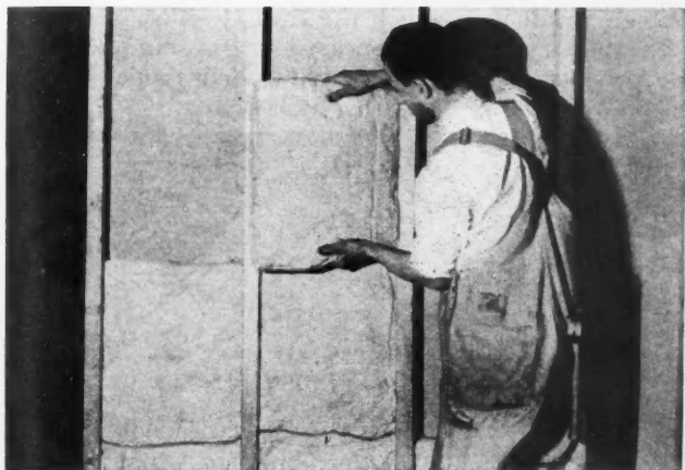
MINERAL WOOL BAT —this is one of the insulation advances of the year. Bats are easily and quickly tucked into place.
