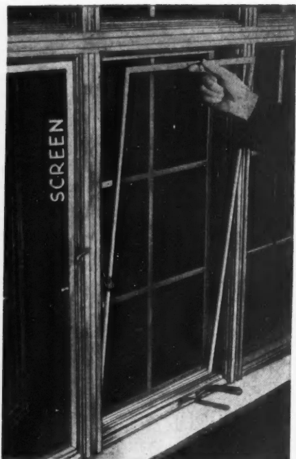
WINDOW UNIT —new type window comes complete with screen units and removable double glazing. Double glass is important for houses having air conditioning equipment.
