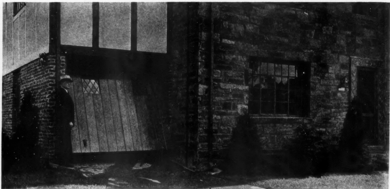
A swing-up type door of rigid construction that harmonizes well architecturally with house.
