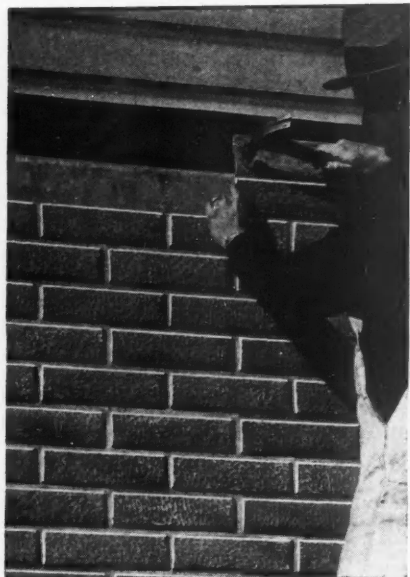
BRICK-TYPE SIDING —asbestos cement product comes in strips 6" x 30", looks like real brick, is quick to apply over old exterior, comes in natural textured brick colors.
