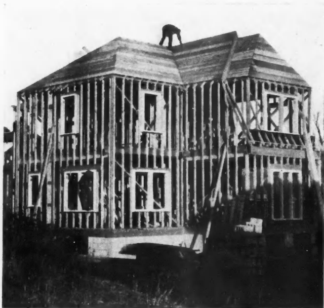
GUIDE-LINE LUMBER —house under construction with new square-end framing lumber. Every piece is accurately squared and every inch marked with guide lines for better work.
