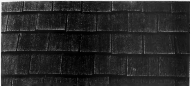
Asbestos Cement Shingle Looks Like Mellowed Wood.
