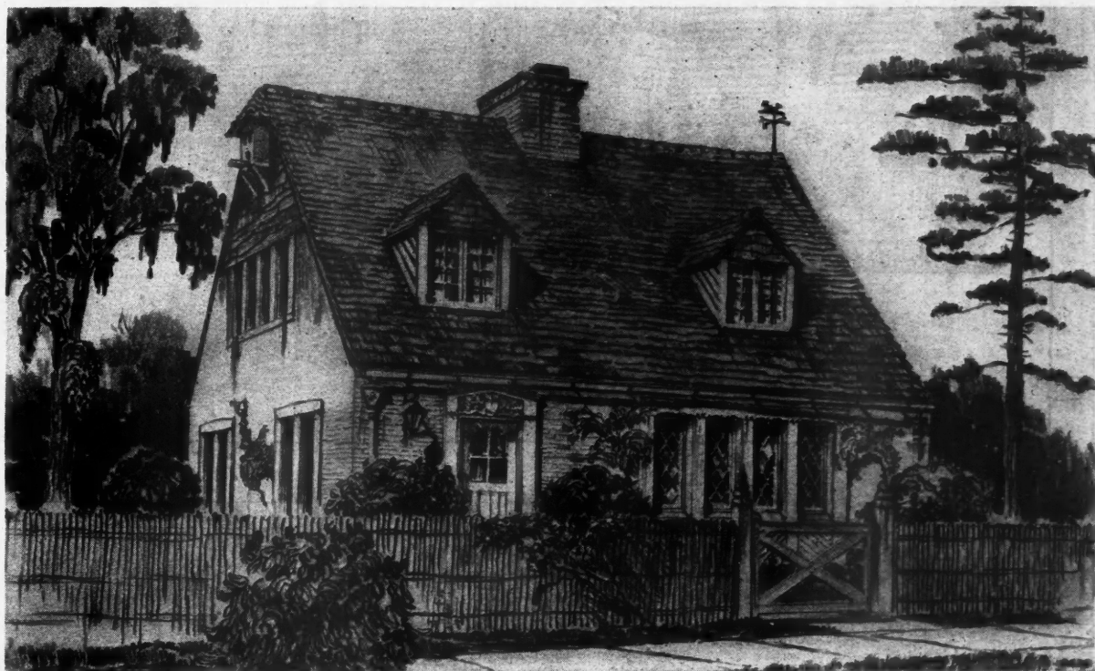
A correctly designed home of English tradition that will always be in good taste
