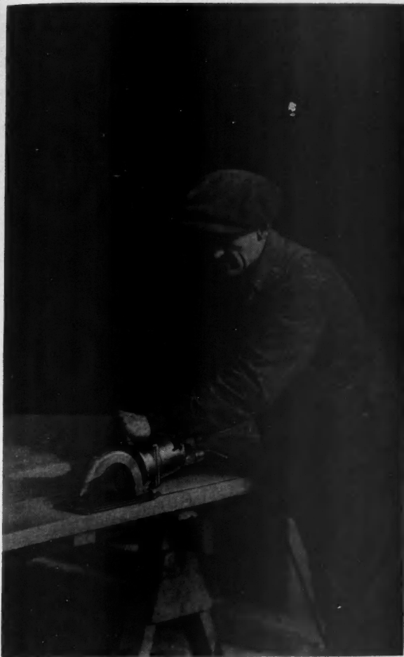
Above: Electric saw with abrasive disc used in routing, cleaning and tuck-pointing the marble joints on the steps and terraces of Field Museum, Chicago.
