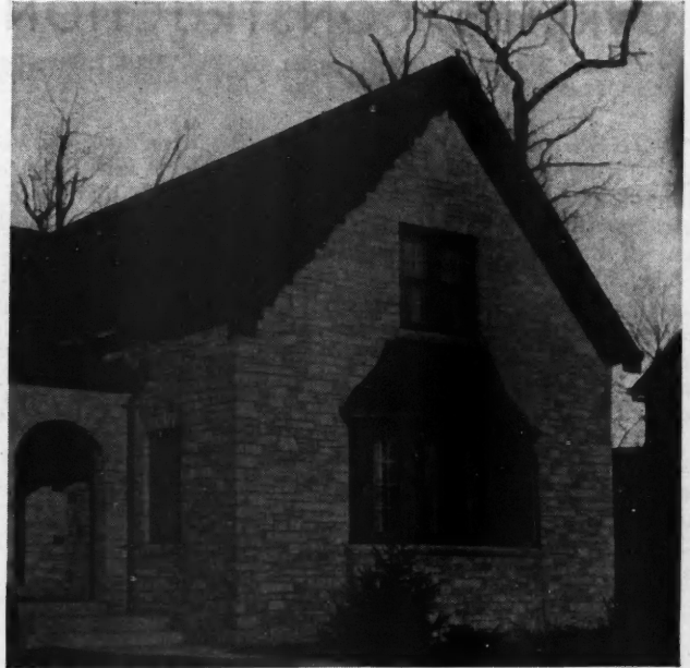
The exterior of this good looking house is of granite block veneer of natural granite four inches thick.
