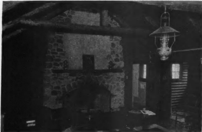
Massive stone fireplace in cottage built by Homeland Co., New York. At right—log cabin of permanent construction that fits surroundings well. Chimney is of second-hand common brick.
