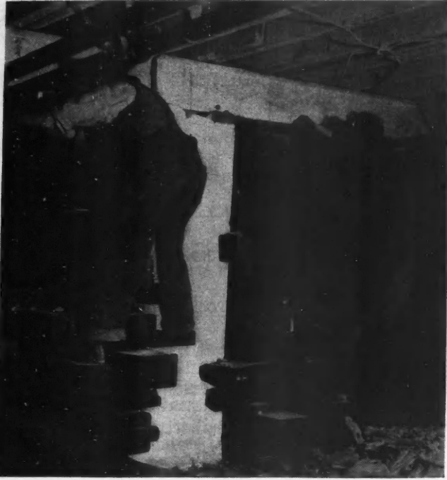
Basement setup of equipment showing how structure was lowered without damage.
