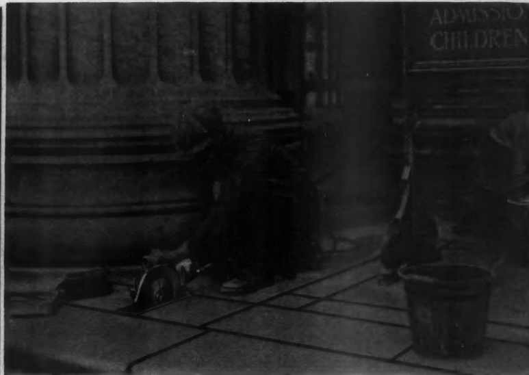
Above: Electric saw with abrasive disc used in routing, cleaning and tuck-pointing the marble joints on the steps and terraces of Field Museum, Chicago.
