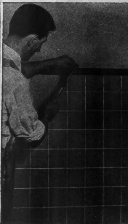
Cap and base—either of wood or asbestos—are nailed in place. As easily applied as the sheets.
