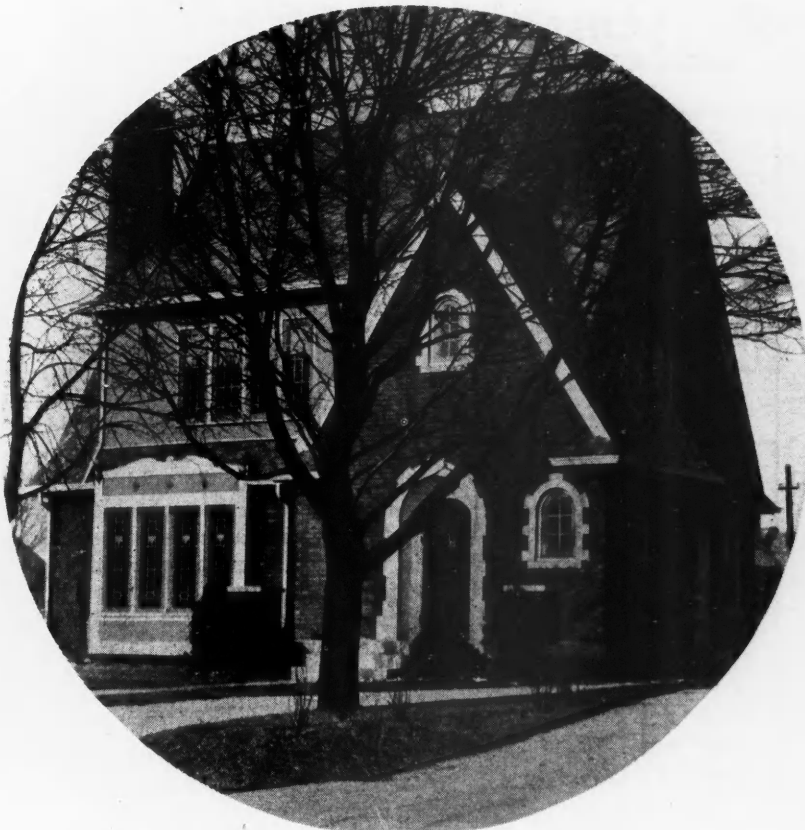
One of the abuses of the design on the opposite page, which depreciates the value of the original house. Changes in seemingly unimportant details have stolen away much of its charm.
