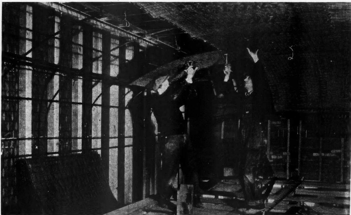
The Third Floor Living Rooms of the Leeb-Tyroler Apartments Have High Vaulted Ceilings. Photo shows simple method of attaching metal fabric plaster base to attachment bars to provide curved surface.
