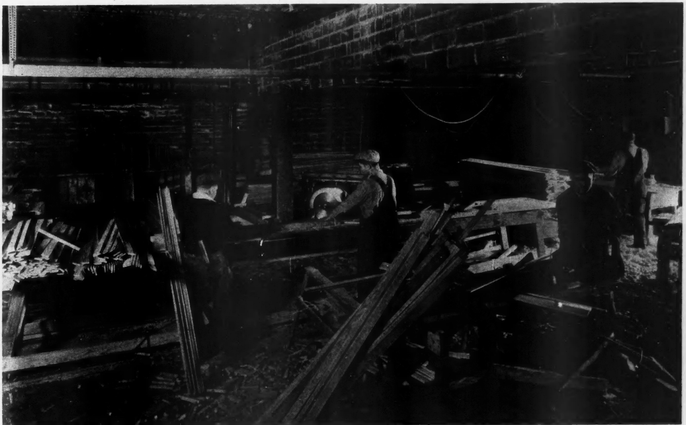
Portable Power Woodworking Shop Set Up in the Basement of the Leeb-Tyroler Apartments by the Carpenter-Contractor. Two men with power saw are mitering window stops and other wood trim on a production basis. Note racks and bins in background for storage of the different members.
