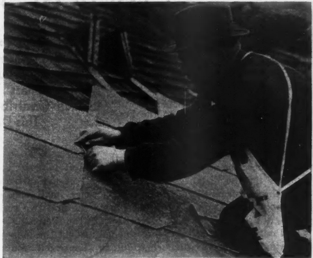
Fine Asbestos Shingle Roofs Have Been Made Inexpensive by an Anchoring Device Which Reduces the Cost of Application.
