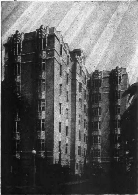
Moffett Apartments, Hollywood, Cal. Leland A. Bryant, Architect. Windows by Soule Steel Co. Glass by Thompson Glass & Paint Co.
