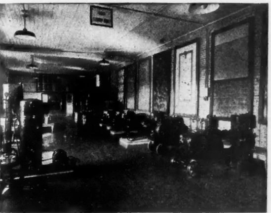
The photographs show parts of the various DeVilbiss schoolrooms in which students are trained free in the use of spray-painting and spray-finishing equipment.
