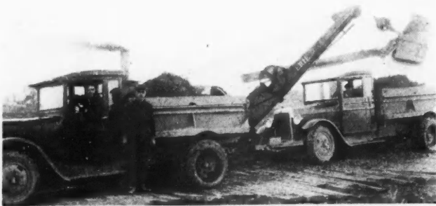
Three-ton Trucks with Special Dump Bodies Are Able to Get in Close for Hauling Out Excavated Materials.
