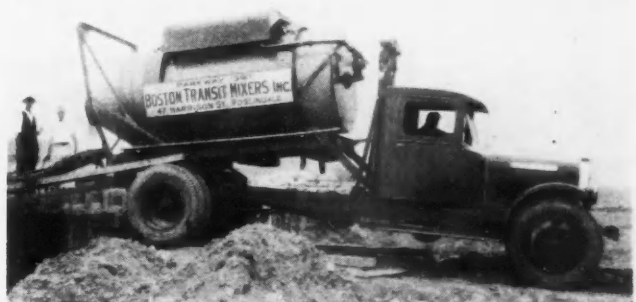
Six Balloon Tires Give Traction for This Special Mixer Truck Over Soft Going on the Building Site.
