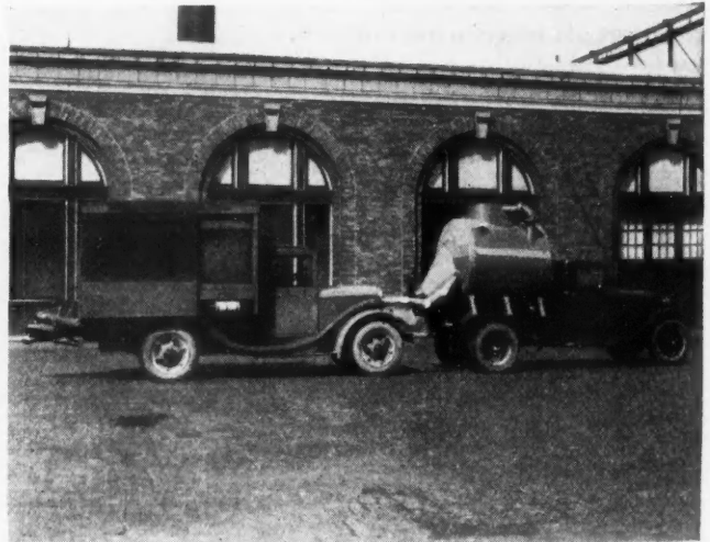
Removing Ashes by Suction, Without Noise or Dirt, at Low Cost.
