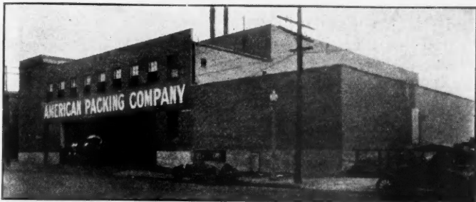
American Packing Company Building, St. Louis, Mo. Koerner Engineering Company—Engineers Herklotz & Herchert—Contractors
