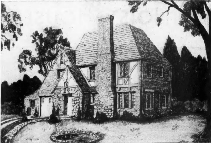
This Attractive English Type Home with Attached Garage was Built with Masonry Bearing Walls and Steel Joist Floors to Sell Complete with Improved Lot at $11,500.
