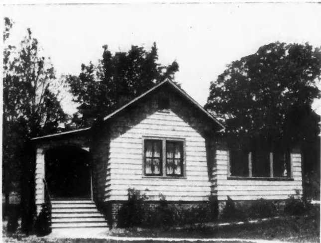
This Neat Little House Took on a New Value from Modernizing Suggested by the Builder
