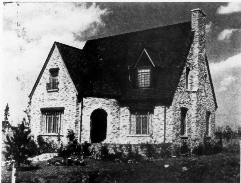
A Home in Jewel Park; Brick Construction, Six Rooms, Normandy Type, Size 31 Feet 6 Inches by 32 Feet 3 Inches; W. H. Floerke, Architect; for Floor Plans See Page 79.
