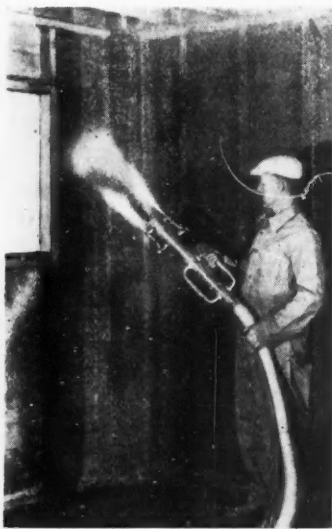
Applying Insulation with a Gun.
