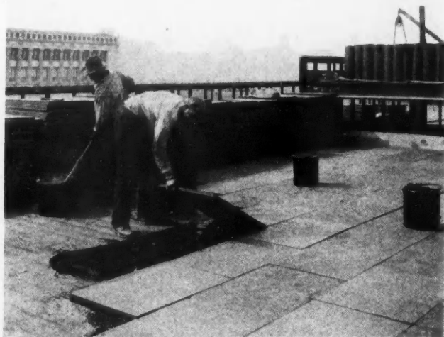
Applying Insulation to World's Fair Building
