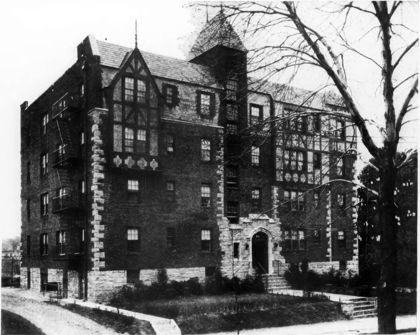
Apartment in Mt. Vernon, N. Y., Louis Levine, Architect Fitzgerald Building & Construction Company, Builders
