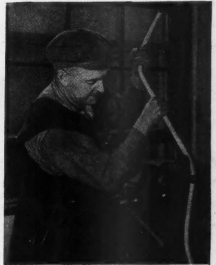
Workability and Elimination of Thread Cutting Make This Metallic, Electric Tubing Economical.
