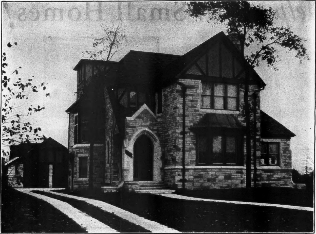
Residence, Detroit, Michigan. Charles Valentine, Jr., Architect. Lawrence B. Keim, Builder. Built of Sawed Indiana Limestone Random Ashlar, with cut-stone trim.
