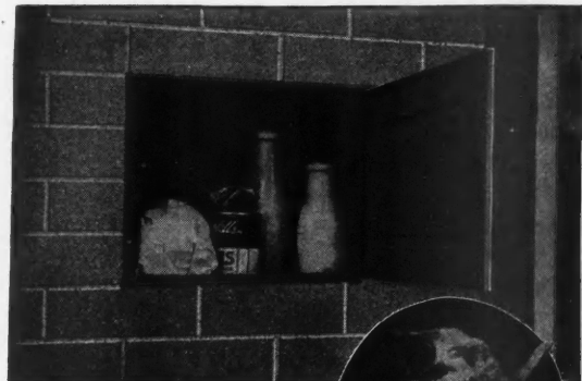
Protection of Deliveries and Convenience for the Housekeeper Are Provided by This Built-In Package Receiver.
