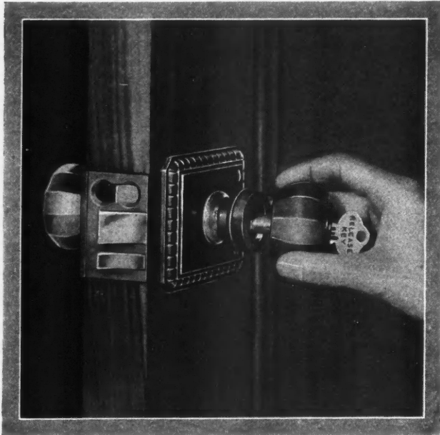
Flexibility of Keying Has Been Highly Perfected in These Locks by Means of Demountable Knobs and Exchangeable Cylinders.
