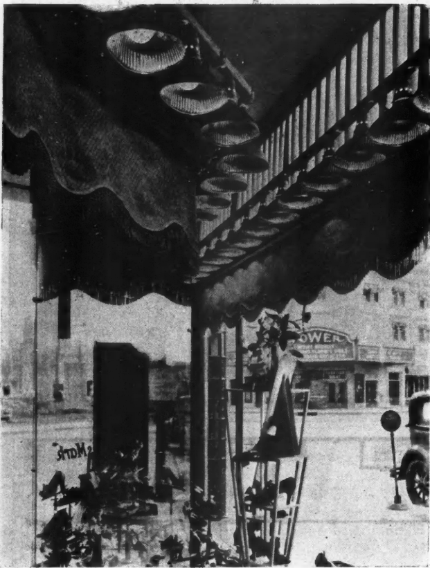
Show Window Lighting Equipment Used for the First Floor Shops in the McClatchey Building.
