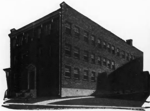
In this apartment house for F. W. Bengel, Laminex doors have proved very satisfactory, writes J. H. Angel
