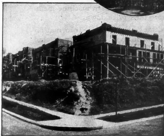
Steel reinforcing completely embedded in stucco will protect the exterior of these modern apartments at Oakmont, Penna. The owner and builder, John McSorley, prominent building developer of Pittsburgh, Penna., is using STEELTEX in direct-to-stud construction. In addition to insulating and sound-deadening, the double waterproofed backing of STEELTEX for Stucco shuts out dampness.
