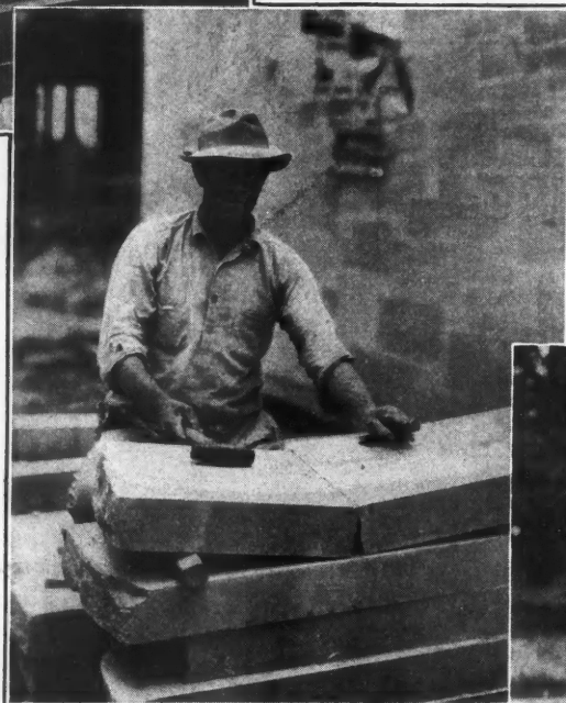
(Above) Preparing Indiana Limestone Random Ashlar with aid of coping tool. Note opening in wall showing construction. Here stone is being used as structural facing over hollow tile.
