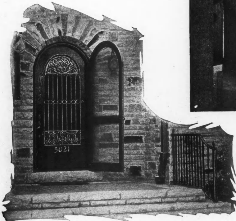
Ornamental Iron Is at Last Receiving Its Proper Recognition in This Country. An example of the excellence of American ornamental iron is seen in this wrought iron door grille and railing produced by the Badger Wire & Iron Works for the residence of Dr. Tainter, of Milwaukee, Wis. A. C. Sehrt Co., designers and builders.
