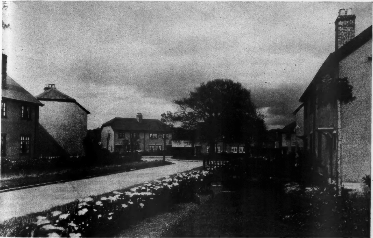
Burman Crescent, One of the Housing Projects in the Liverpool District Which Has Been Developed to Provide Suitable Homes for British Veterans of the Late War, in Accordance with Wartime Pledges. The houses in this group are all of concrete and every house must be provided with a modern bathroom.
