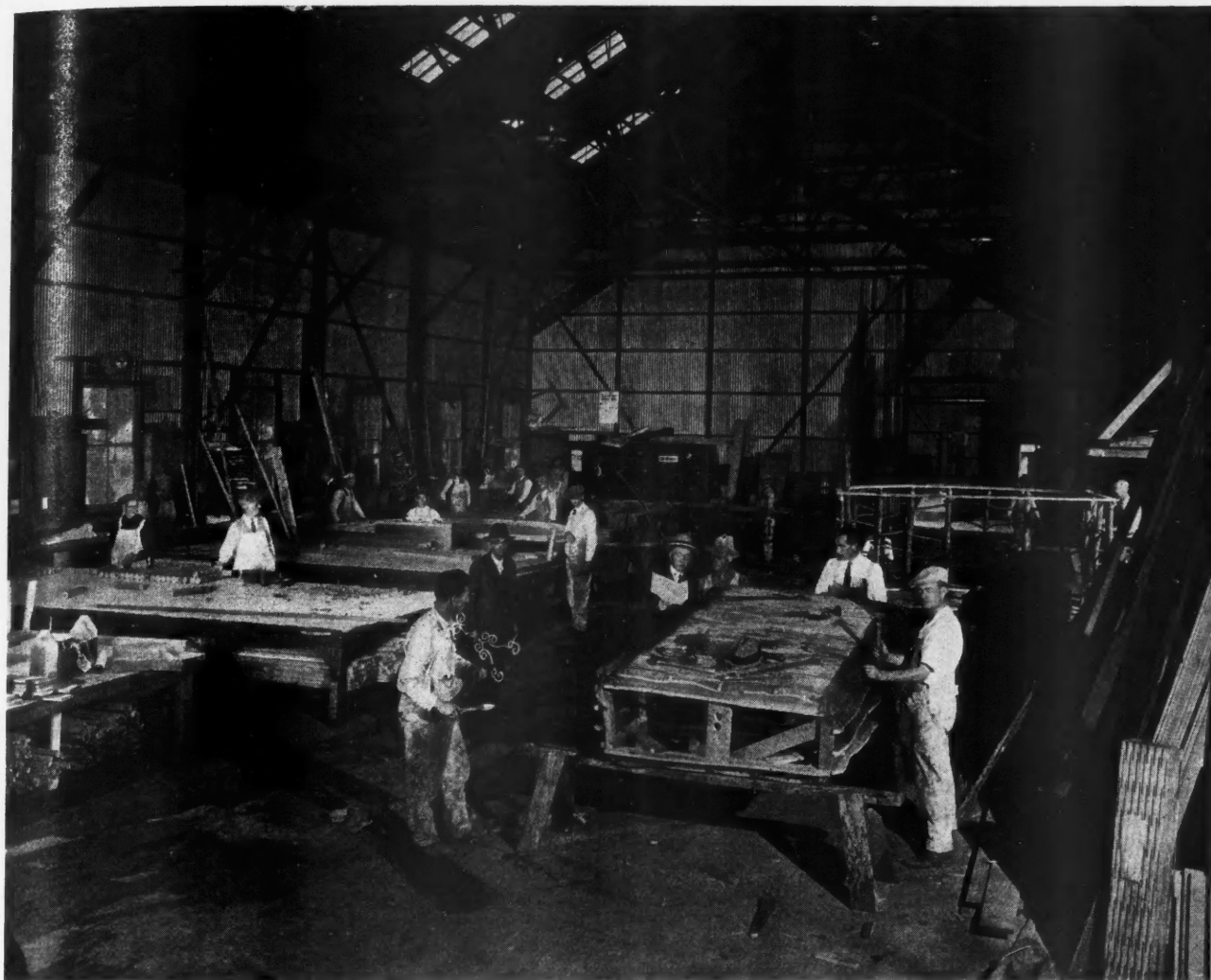
Largest Carpenter Shop in the West. Section of the tremendous construction department at Paramount Hollywood studio. Hundreds of expert workmen make everything called for by Famous Players-Lasky films, from a toy to a huge house, from a propeller blade to a wooden frigate cannon. It is one of the finest studio industrial plants in the world.
