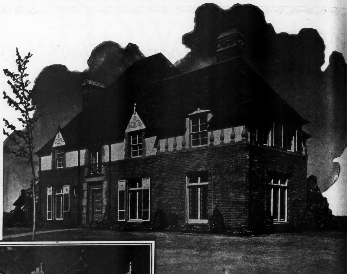
Masonite Insulating Lath was used as a plaster base in both of these fine homes
