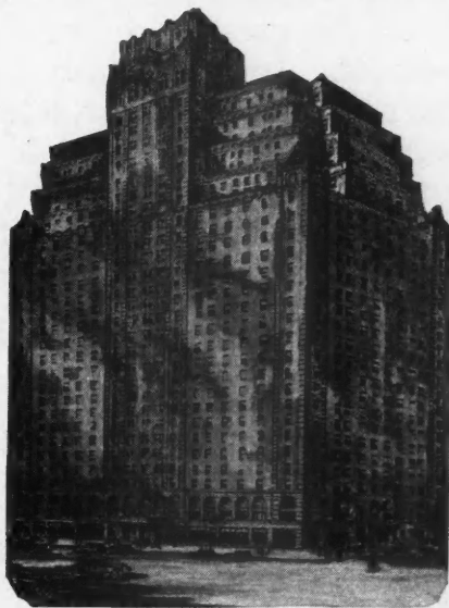
Lincoln Hotel, New York City. One of the newer buildings equipped throughout with the Brunswick White Seat
