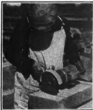
Portable electric saw replaces old mallet and chisel method of breaking stone. One man at ordinary wages now keeps six stone-masons busy!
