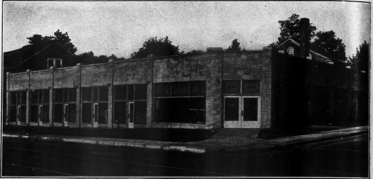
Carter Block, Indianapolis. E. H. Dalby, Designer and Contractor. An example of a moderate-priced store building built of Variegated Indiana Limestone Random Ashlar.
