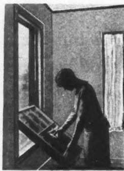
Two Views Showing How This New Type of Tilting Window Operates, Permitting Easy and Safe Washing from the Inside.
