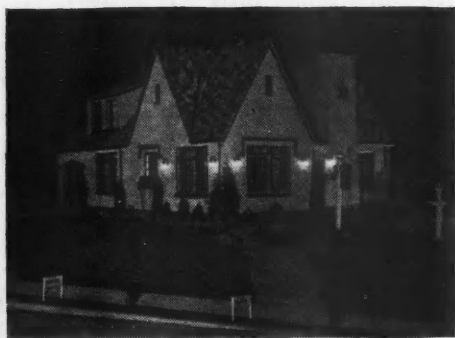
Eternit Heatherblends used on the Ideal Home at Asbury Gables, N. J.
