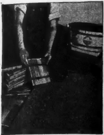
A complete unit of four flooring strips, splined together
