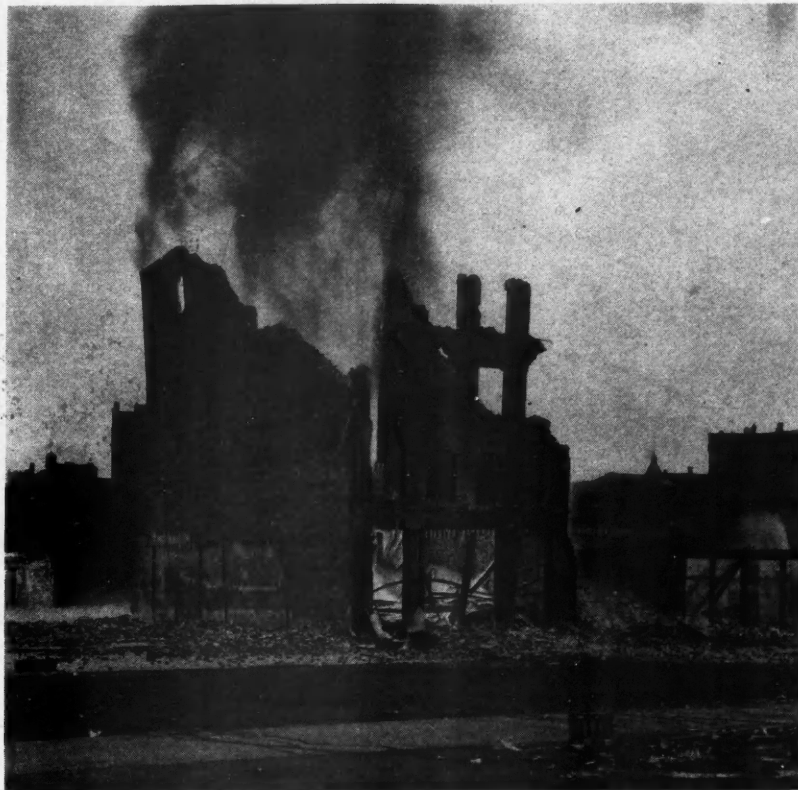
During the Actual Burning, the Steel Roof Remained Intact, an Effective Protection, Until the Entire Interior Was Burned Out, Practically Ending the Danger of Fire Brands, and Only Fell When the Brick Walls Collapsed.
