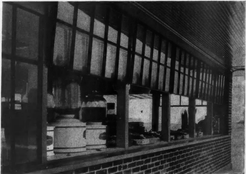
These Steel Windows Are Hinged to Be Raised Out of the Way as Shown. They are also equipped with glass which can be replaced with steel sheets during the closed season.
