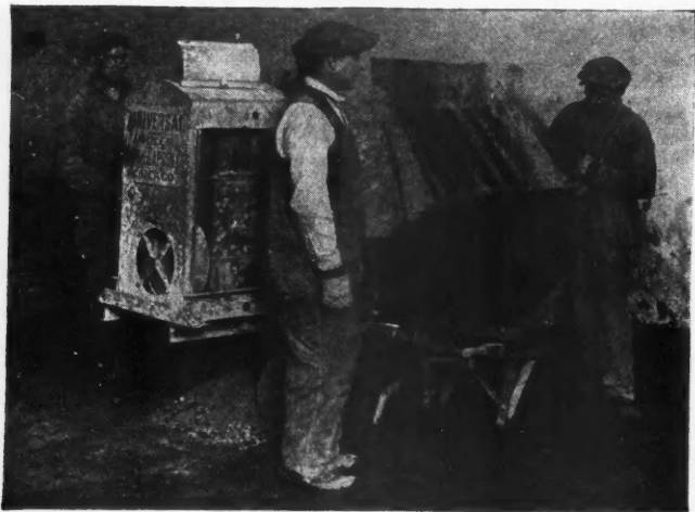
This Type of Plaster Mixer Has Been Used with Excellent Results for Mixing Concrete for Floors.
