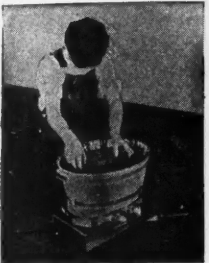
Dipping bottom side in Everbond, a plastic cement
