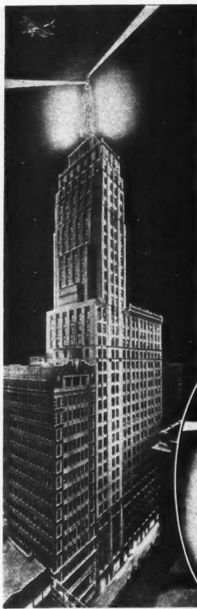
This Aerial Beacon, in Chicago, Is Visible for 100 Miles in Clear Weather to Planes at Certain Altitudes.
