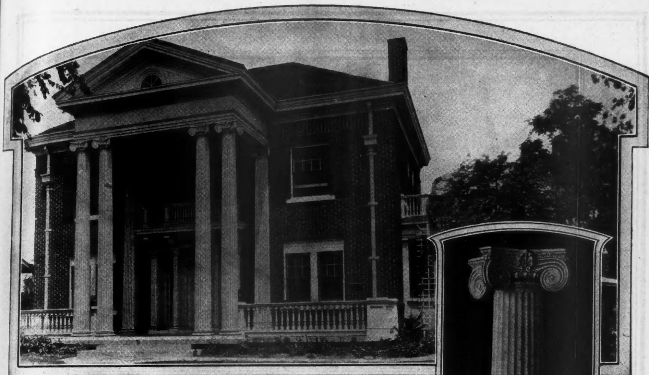
Residence of Doctor Berry, Okmulgee, Oklahoma. Architects, Smith, Rea, Lovitt & Senter. This photograph shows the application of large Union Metal Columns and Square Pilasters.
