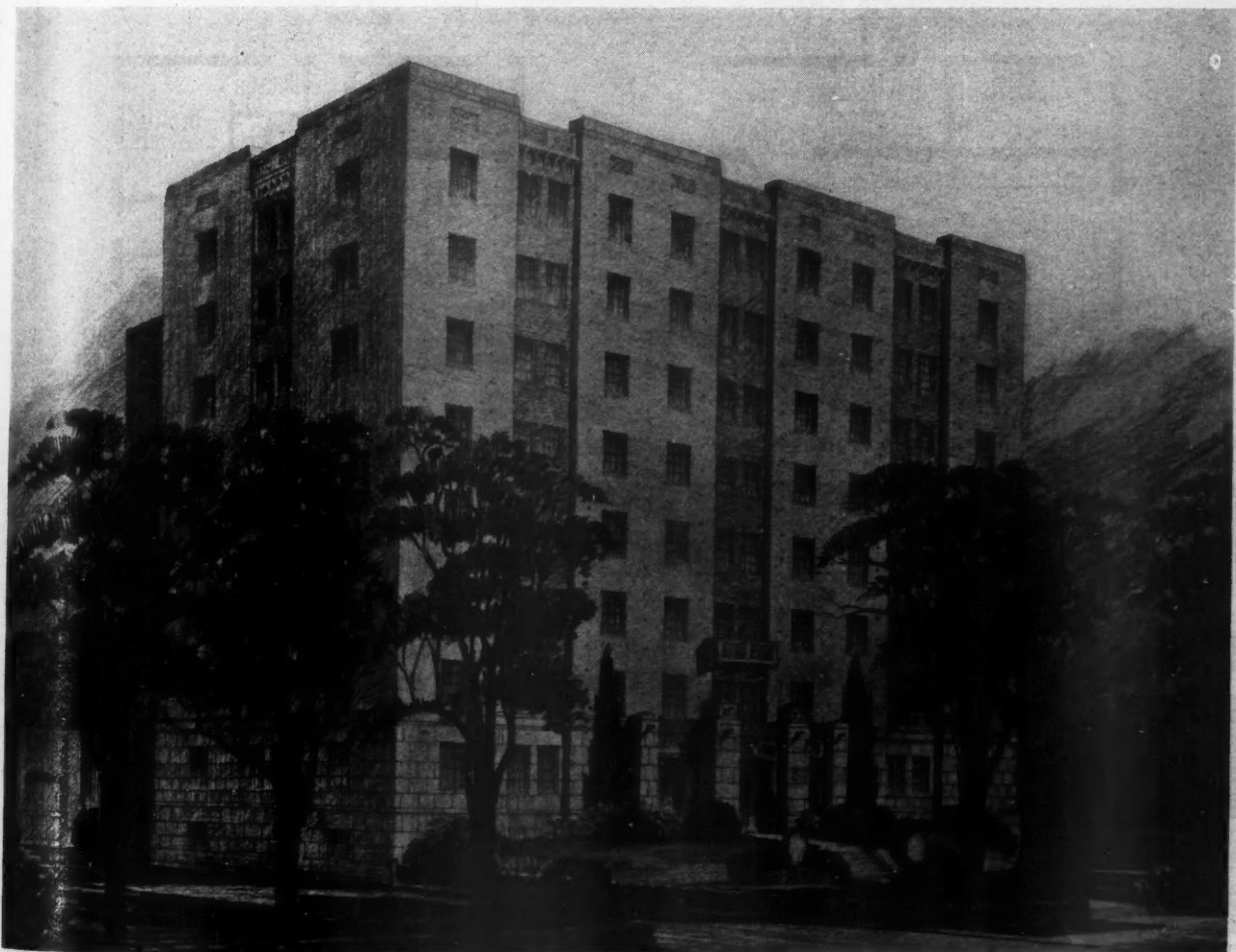
Ambassador Apartments, Pittsburgh; Marks & Kann, Architects.
