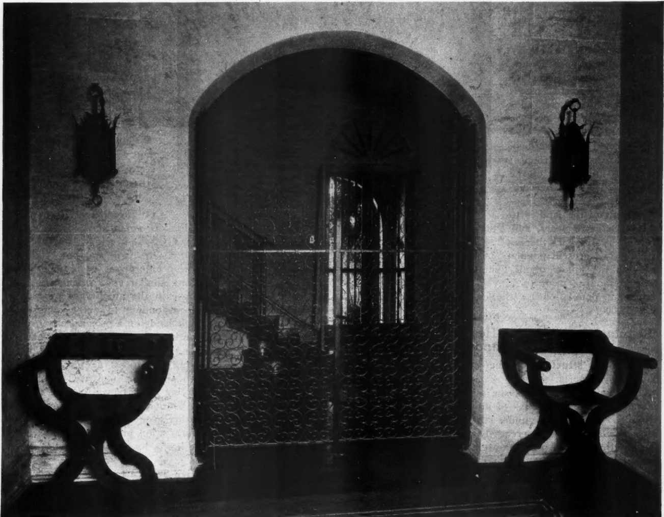
A Travertine Marble Interior Effect Which Has Here Been Developed in Plastic Paint Is Well Set Off by the Harmonizing Iron Grille Gate and Wrought Lantern at Either Side.
