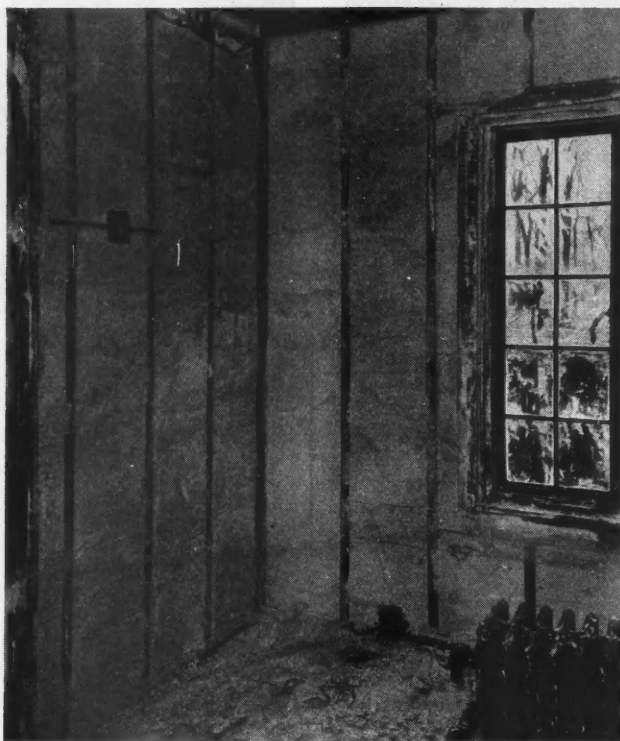
With This Bulk Insulation the Entire Space Between the Studs Is Filled with the Light, Porous, Gypsum Material.
