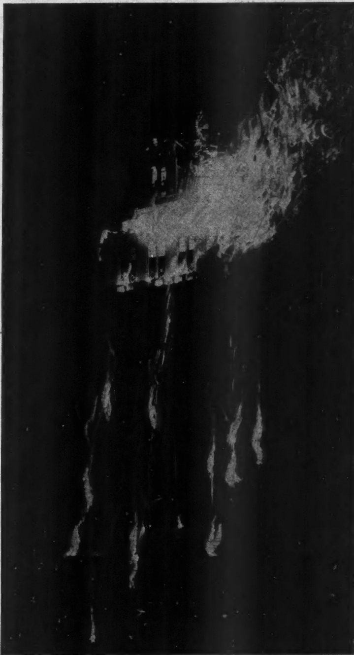
Thousands of New Yorkers Were Thrilled by the Spectacle of a Fire at the Top of This New 38-Story Skyscraper, at 5th Avenue and 59th Street, New York City.
