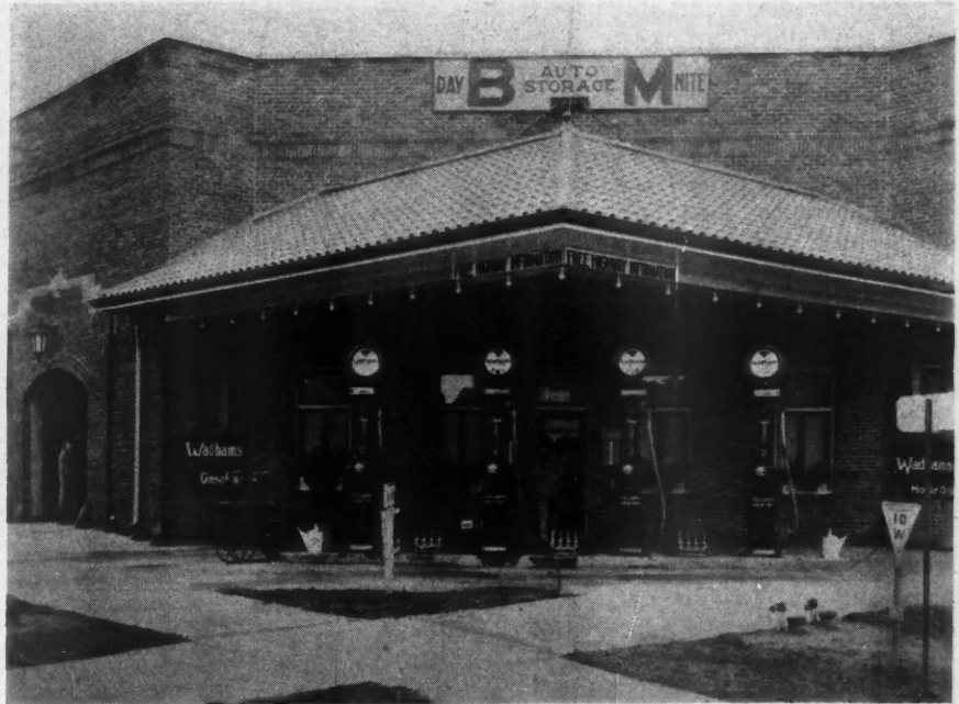
A Filling Station of the Type Which Provides a Canopy Over the Driveway Sheltering the Cars that Drive Up for Gas and Oil Service.
