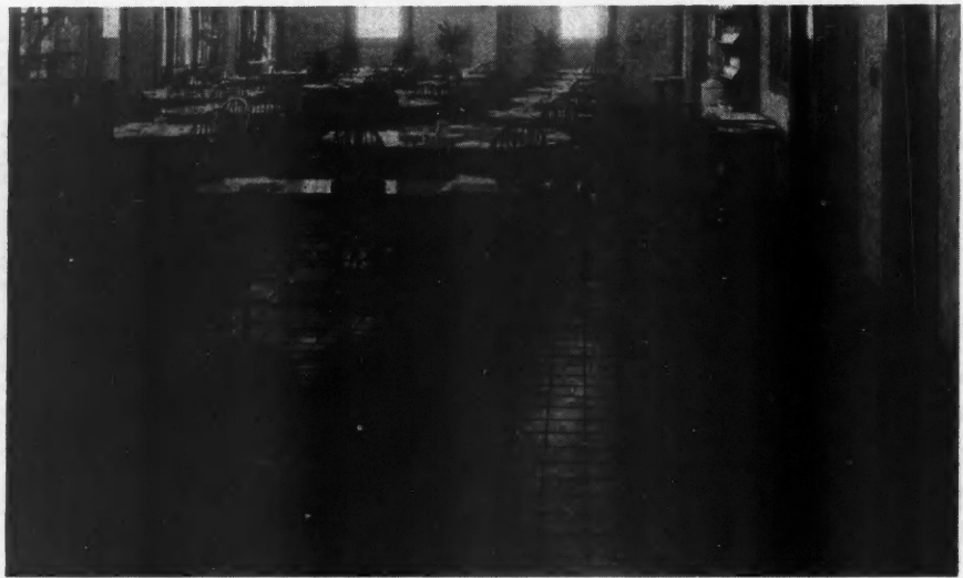
Interior View of Tip Top Cafe, Waukegan, Ill., Showing the Plastic Magnesia Flooring Laid with Tile Effect. It is, of course, important that restaurant floors present a fine appearance and be sanitary and easily cleaned as well.
