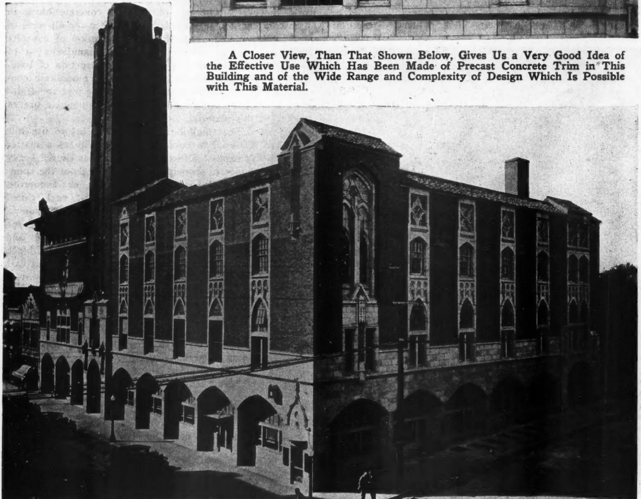
The Scottish Rite Cathedral, Fort Scott, Kan., in Which the Architect, William Schmidt, of Oklahoma City, Okla., Has Developed an Elaborate Decorative Scheme in Precast Concrete Trimstone.
