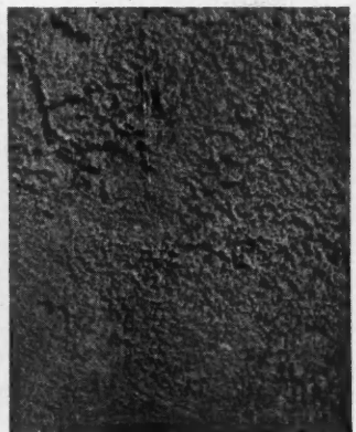
MODERN AMERICAN STIPPLED A smooth surface stippled with a soft, short-bristle brush
