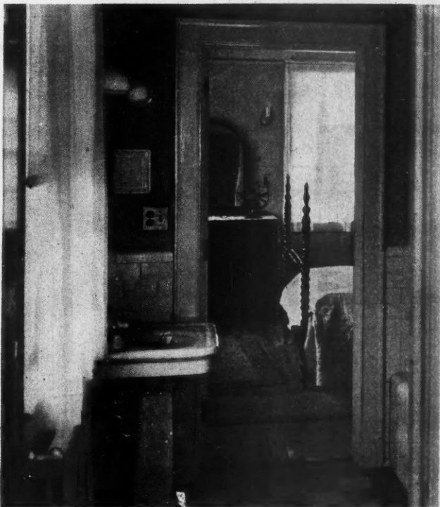
Bathroom Showing Location of Convenience Outlet and Mirror Lights.
