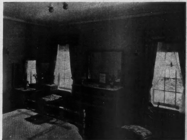
Bedroom Showing Ceiling and Wall Light Outlets and Convenience Outlets. The latter are generally located in the baseboard; however, in many sections the higher location is preferred.
