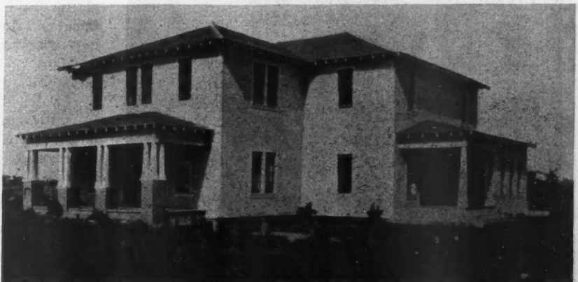
Building at Florala, Alabama, Constructed Entirely of Short Length, End Matched, Yellow Pine.
