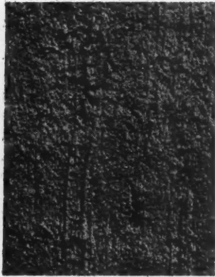
MODERN AMERICAN A texture gained by floating smooth and then roughening with light, vertical strokes of wire brush
