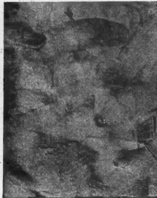
SPANISH A wavy, trowel-marked finish, smoothly irregular
