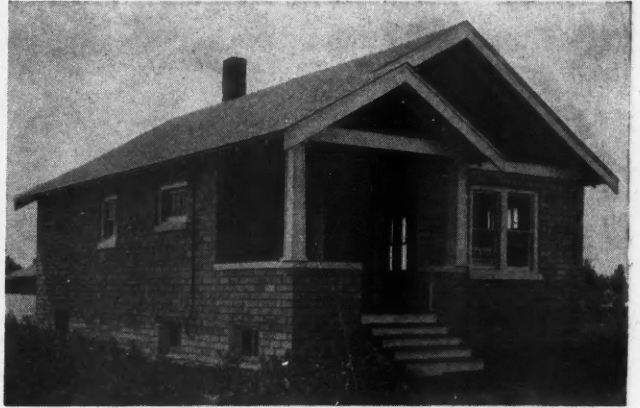
An Inexpensive Garage at Muskegon, Mich., Built of Matt Glazed Tile of an Attractive Tan Color.
