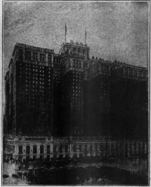
Architects, Holabird & Roche Contractors, Geo. A. Fuller Co. Owner, A. J. Stevens
