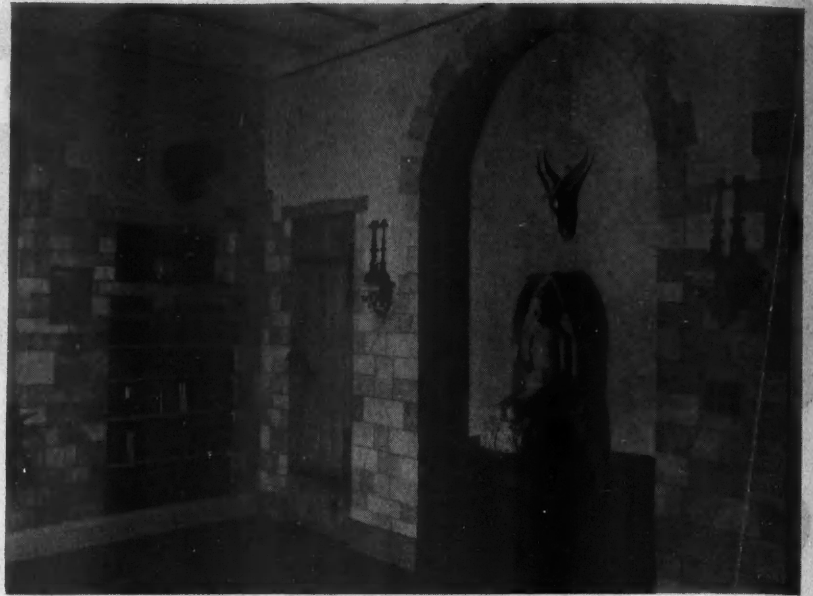
With a Plastic Wall Finish Many Things Are Possible Including an Exceedingly Close Duplication of Certain Kinds of Cut Stone.
