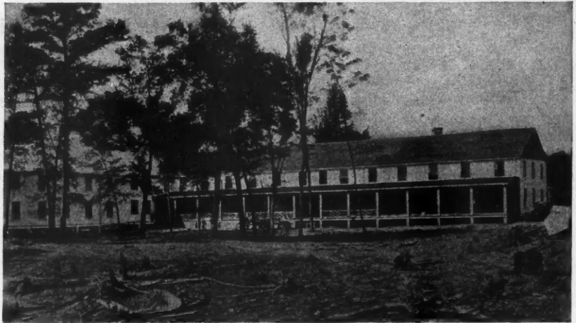
New Employees Hotel at Pine Valley, Oklahoma (a New Saw Mill Town), in Which Every Piece of Ceiling, Siding, Flooring and Partition Is Short Length, End Matched, Yellow Pine.
