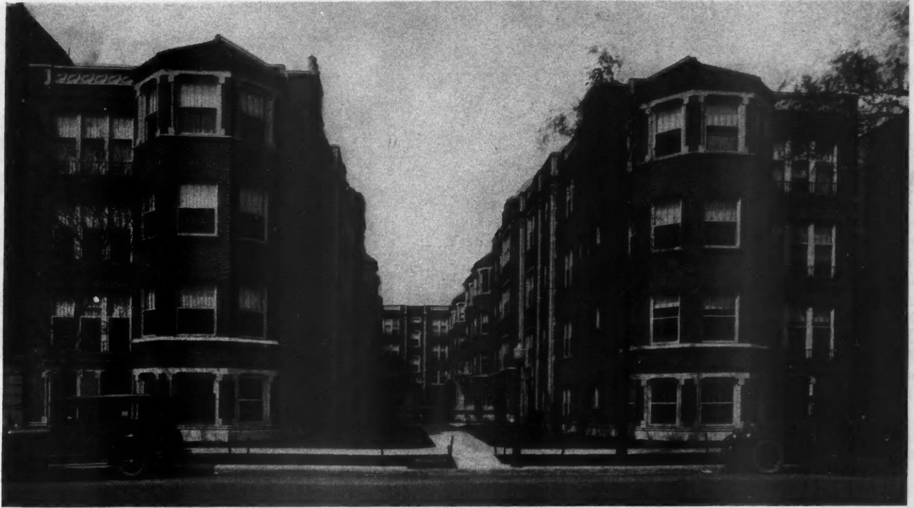
A Chicago Apartment House, Characteristic of the Better Residential Sections of a Larger City, Follows the Now Popular "U" Shaped Plan Giving Good Light and Ventilation for Each Apartment.
