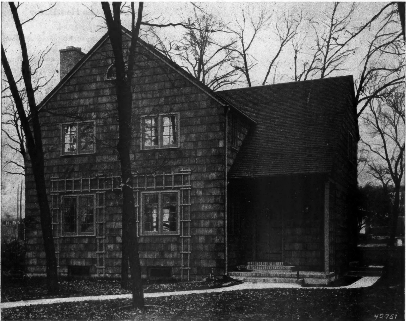
Standardized Knock-Down Window Frames Out of Stock Contribute to the Success of This Well Constructed Minneapolis Residence. Tyrie & Chapman, Architects.
