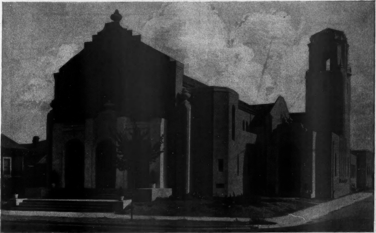
The Presbyterian Church of Fremont, Cal., Is an Interesting Building Especially in the Manner in Which it Varies from the Stereotyped Style of Small Churches and at the Same Time Maintains the Essentials and Spirit of Good Church Architecture.
