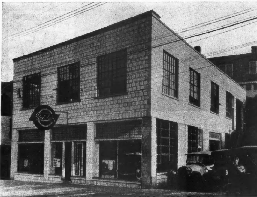
The Studebaker Garage, Morgantown, W. Va., Is a Fine Example of Light Glazed Concrete Building Tile.
