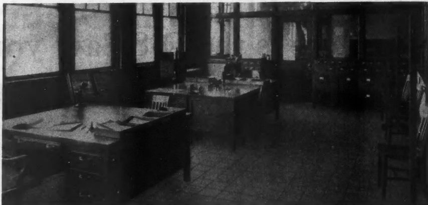
The Attractive Appearance of This Office Is Enhanced by Its Plastic Magnesia Flooring Laid with a Tile Pattern. An increasing number of offices are having this type of flooring installed.
