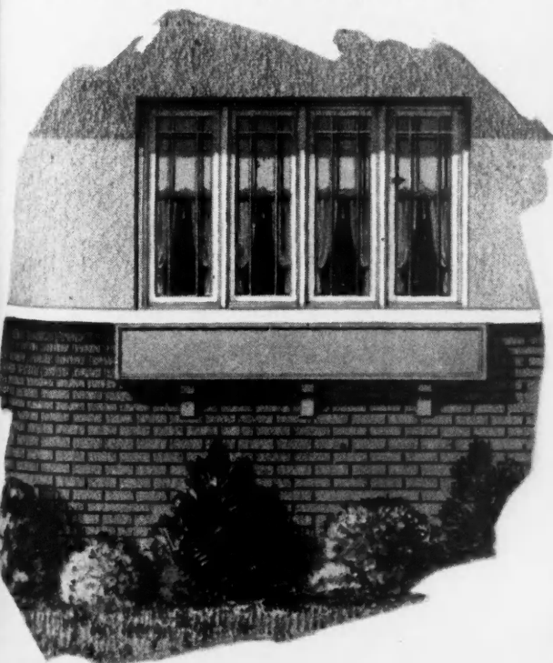
Detail of Front Window Group
