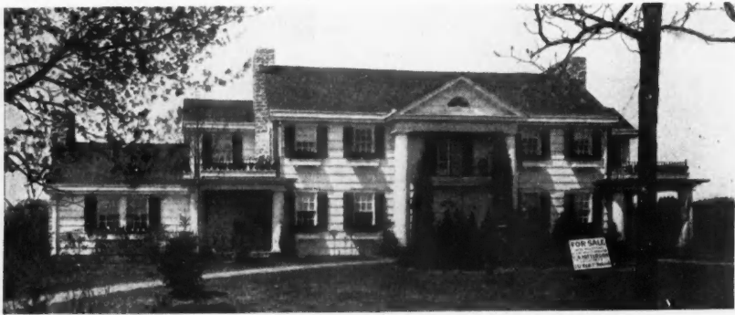
How Long Will This New House Last? The answer depends as much upon the amount of paint that the builder has seen fit to invest in as upon the subsequent paint treatments that the owner subjects it to.
