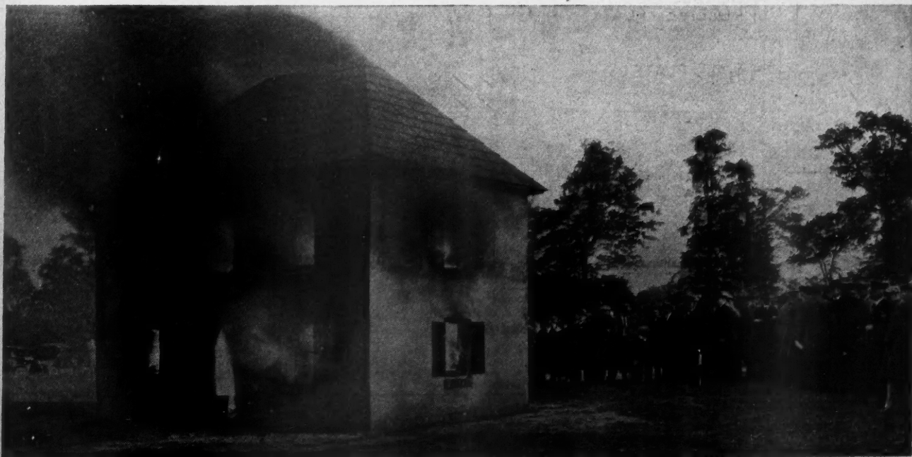
Eight Hundred Interested Spectators, Including Building, Insurance and Fire Officials, Watched This Test of a Small Cinder Block House, Which Was Made as a Feature of Fire Prevention Week, in Indianapolis, Indiana. The blocks were entirely undamaged after a 45-minute test in which the temperature reached more than 1,800 degrees.
