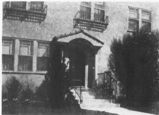
The Use of Wrought Iron Is Not Limited to Spanish Designs as Can Be Seen from This Hand Rail Which Is Equally Suitable for the Colonial Home.
