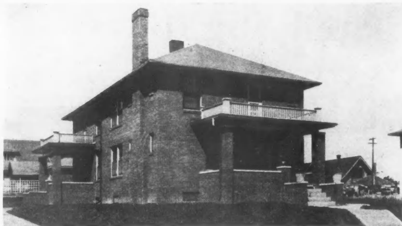
Several Duplex and Four-Family Homes Are Built Each Year by the G. A. Kelly Company at Flint, Mich., and Every House When Finished Is the Product of Experts Throughout.
