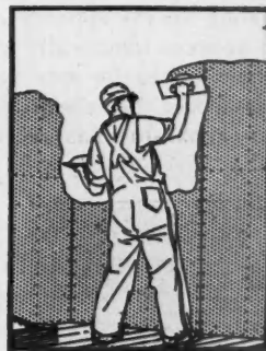
T. A. Curtis, Montclair, N. J., built this house for himself. He used Celotex Insulating Lumber on inside walls in place of lath. Plaster is applied directly to the surface of Celotex, forming a stronger wall than lath and plaster—and a wall that stops heat, deadens sound and is free from lath marks.
