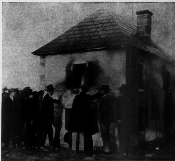
Even When the Blocks Were Red Hot Inside the House, the Outside Surface Was Just Warm to the Hand, an Indication of the High Fire Retardant Qualities of This Building Material.
