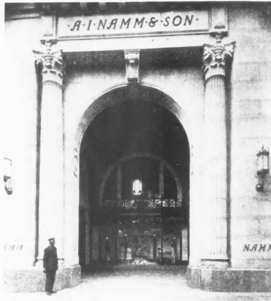
Entrance to the A. I. Namm & Son Store, in Brooklyn, N. Y., Showing the Rear Window in the Vestibule Which Is the Striking Feature of the Layout.
