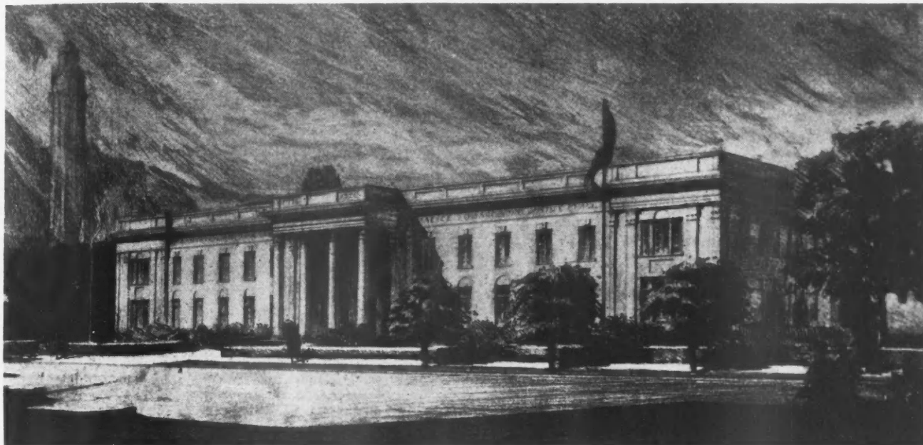
The Administration Building at the Sesqui-centennial Exposition Will Fittingly Follow the American Colonial Style of Architecture.
