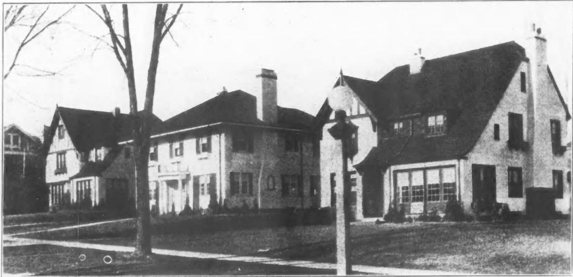
Bishopric Row—Bishopric Stucco over Bishopric Base in this row of Rochester, N. Y., houses.
