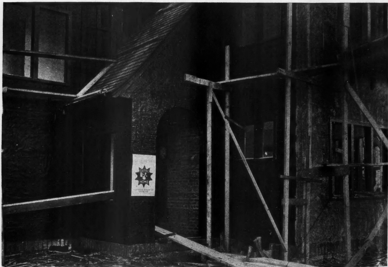
A Red Seal Card on Any House Means That It Has Been Adequately Wired for Electric Comfort and Convenience in Accordance with a Carefully Worked Out Plan and Accurate and Complete Specifications as Provided in the Movement Sponsored by the Society for Electrical Development.
