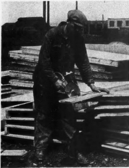
Weighing Only 15 Pounds and Operating from Any Light Socket, This Little Saw Will Cut Thousands of Feet of Lumber in a Day.
