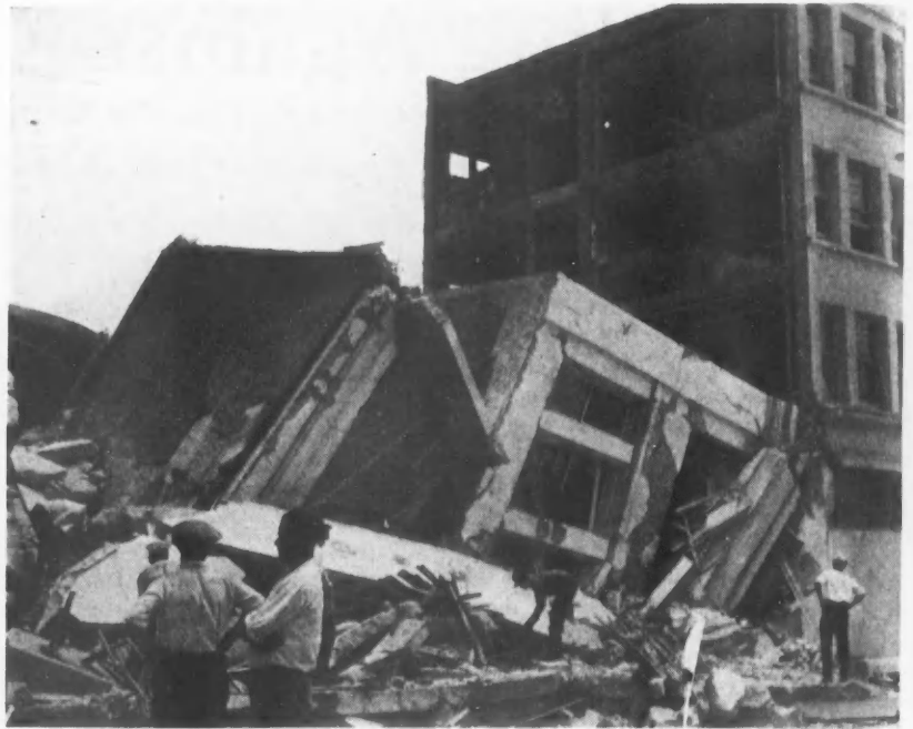
Showing What Happened to an Addition Built Onto One Building Without Any Visible Effort to Tie the Two Units Together. The addition was completely demolished.
