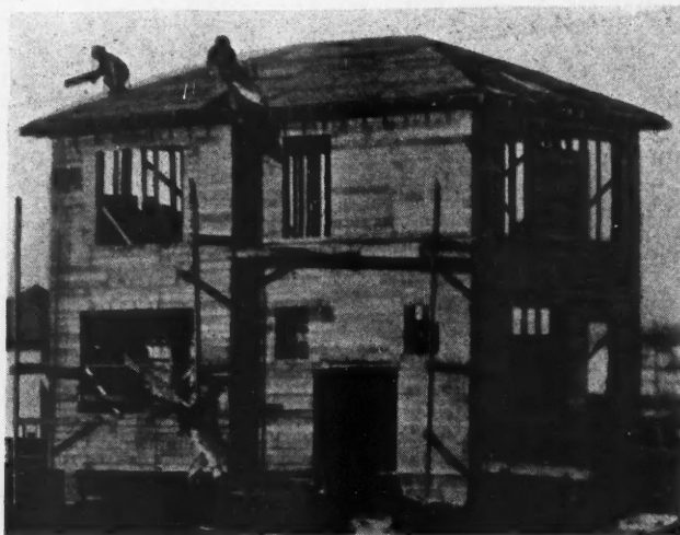
Photo 6—Here Is a House Which Is Sheathed and Roofed with 1-Inch by 6-Inch by 5-Foot 1/2-Inch Car Roofers.
