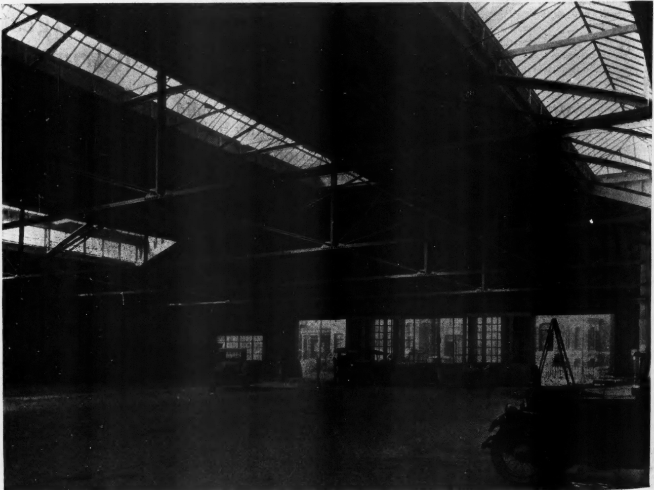
Garage Building at Chicago; 125 Feet Wide; Six Steel Trusses Approximately 20 Feet on Centers. Note the sloping of the joists in the end bay to reduce the height of the end wall.
