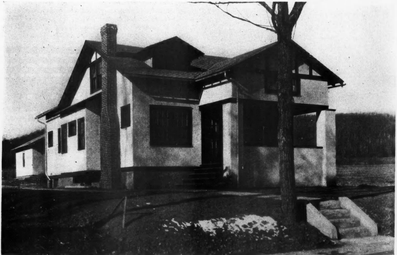
Here Is a Fine Example of the Sort of Houses Which the Hackettstown Investment and Development Company Is Building in Its Belwood Terrace Addition and Selling at Prices Which Place Them Within the Reach of Families of Moderate Means.
