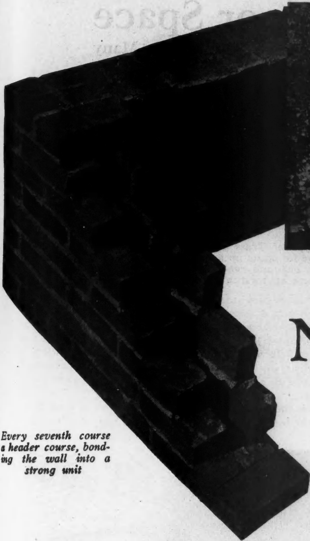
The Ideal Rolok-Bak Wall Has the Same Pleasing Appearance as Any Brick Construction
