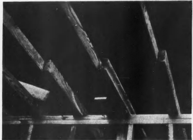
Photo 1—Here Is an Avoidable Lumber Waste in the Overlapping of Joists Which Are Longer Than Required.
