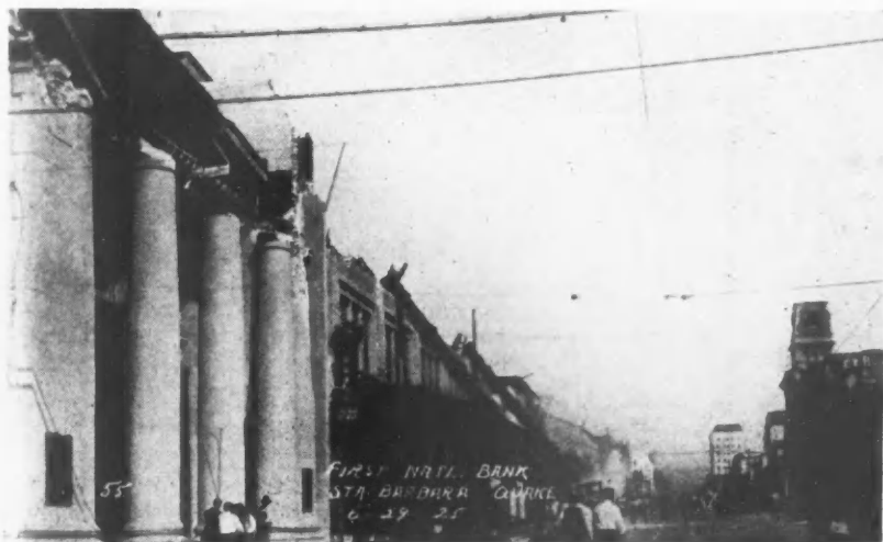
The First National Bank, the Concrete Columns of Which Stood Intact While the I-Beam, Not Properly Tied, Fell Off.
