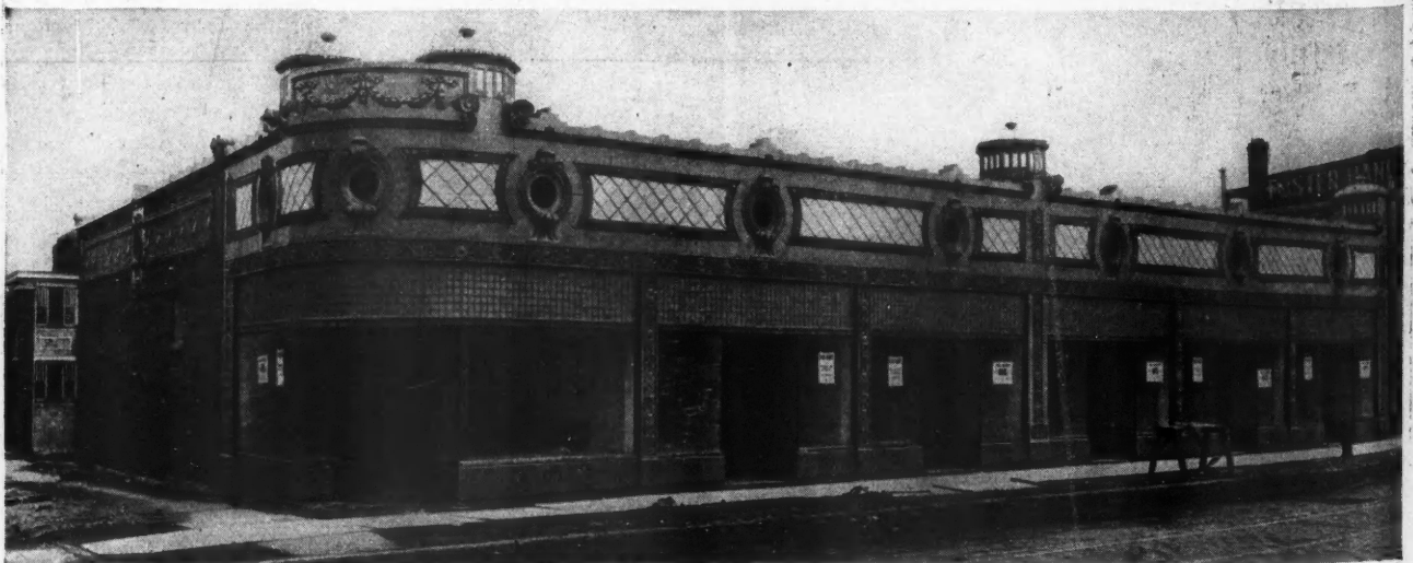
The One-Story Block of Stores in This Picture Was Photographed Just Prior to Completion. Note the unusual attractiveness of the terra cotta ornamentation, metal store fronts and prism transoms.
