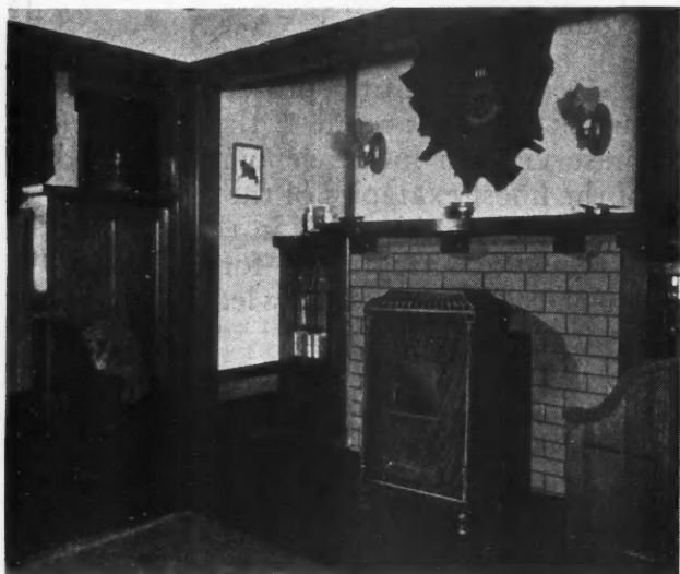
For the Cellar-less House Which is Now Attracting Such Great Attention, This Cabinet Heater Affords an Efficient Heating Plant and Attractively Designed Piece of Furniture.
