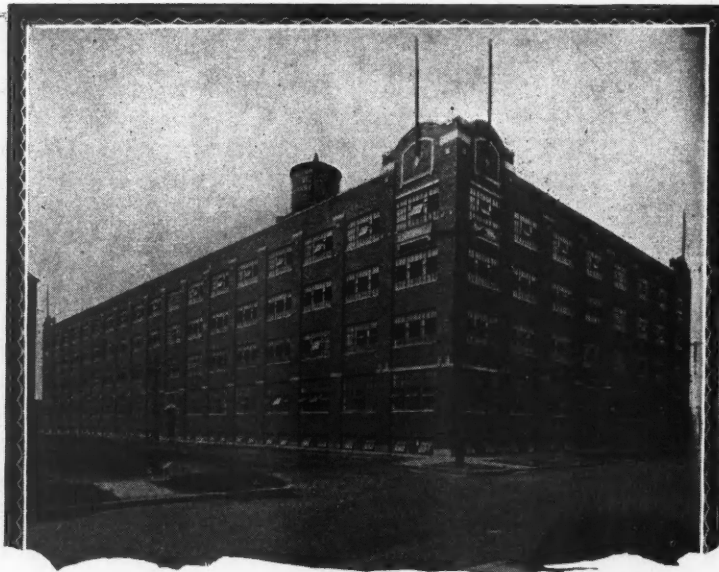
Factory Building of the Appleton Electric Company, Chicago, Ronneberg and Pierce, Architectural Engineers.
