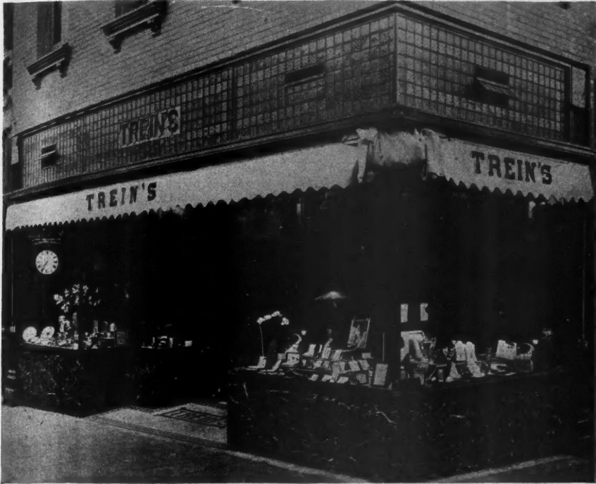
This Jewelry Store in Dixon, Ill., Is a Good Example of What Store Front Remodeling Can Accomplish. Note the marble base, the metal store front, the plate glass, the prism glass transom with merchant's name in colored glass and the mosaic tile entrance.
