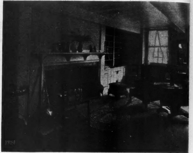
Fig. 1. A Typical Old Colonial House Which Was Recently Restored. It is equipped throughout with hand forged hardware, wherever pieces of the original hardware were missing, new pieces were made to match perfectly.
