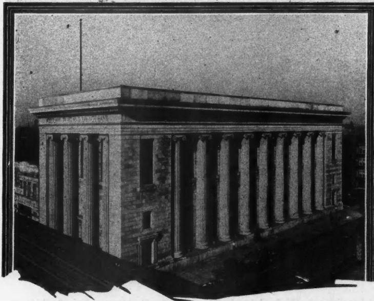
Woodlawn Trust and Savings Bank, Chicago, Weary and Alford, Architects.
