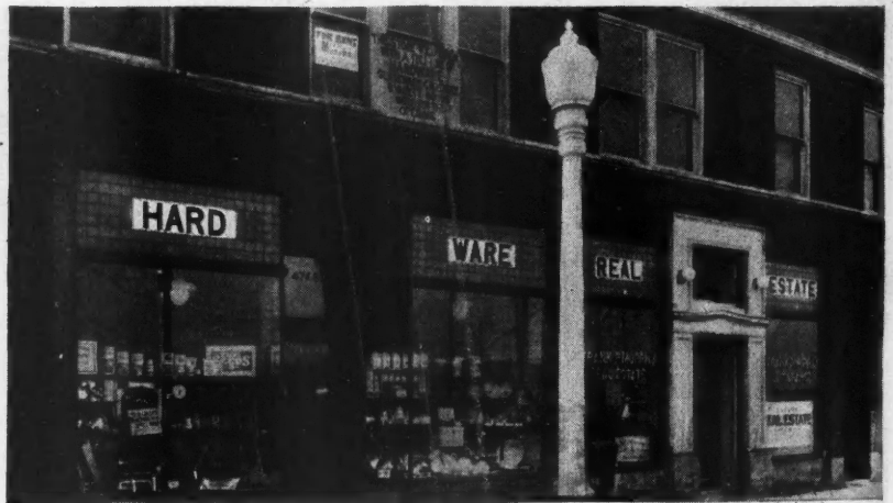
This Picture Shows Two of Sixteen Stores in a Block Built "Out on the Prairie," but Quickly Leased. A clever use was made of transom lights and ornamental glass signs which helped in achieving this result.
