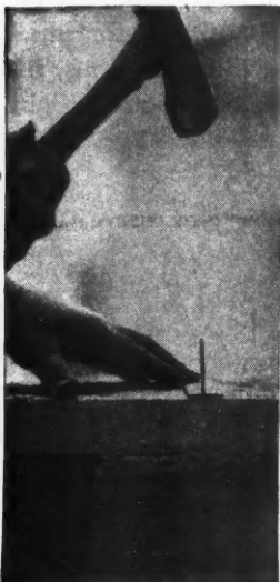
Left: Nailing Anchor on Two by Two Strip. Above: Backmortaring the Wall.
