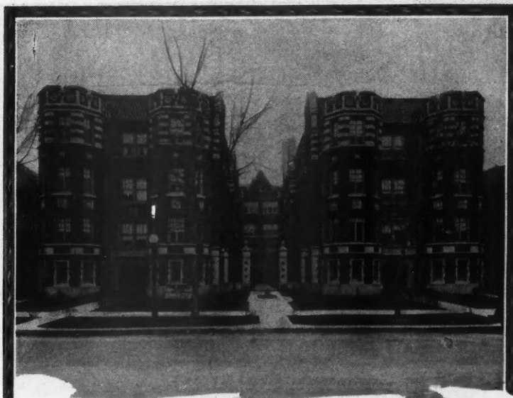
The Birchwood Beach Apartment Building, Chicago.
