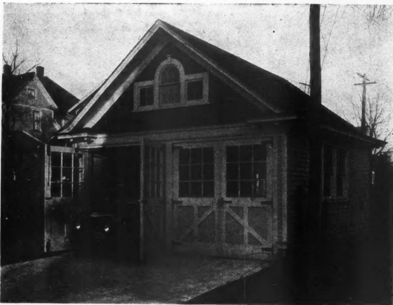
Double Garage with Hinged Doors Properly Equipped with Hold Back Rods.
