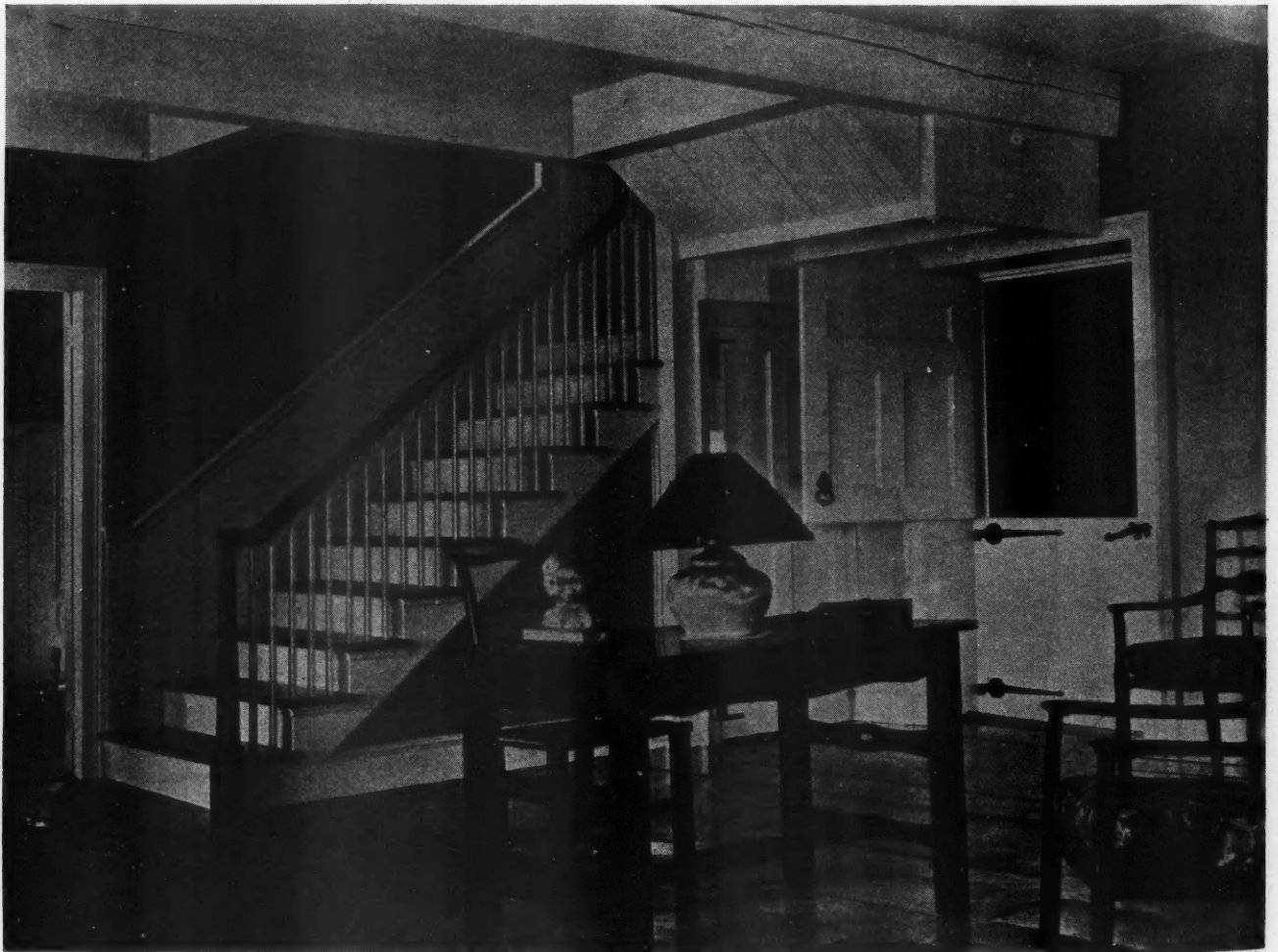
Fig. 2. Hall in an Old, Stone Colonial House in Ulster County, N. Y. Here is a fine example of the Colonial stairway, wide board flooring and heavy beamed ceiling. The top section of the Dutch door is open, showing the drop handle, while the lower half shows the inside latch and strap hinges. The door under the stairs shows the use of H-L hinges.
