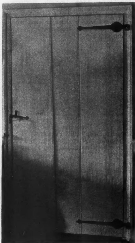
Fig. 4. A Batten Door in the Old Van Buren House, Kingston, N. Y., Showing the Use of Strap Hinges and Latch.
