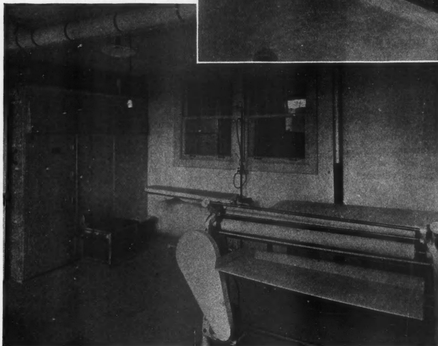
This Well Lighted Basement Has a Very Completely Equipped Laundry. Here are shown the electric ironing machine as well as the ironing board for a hand electric iron. The laundry gas stove is shown, also the gas-fired clothes dryer.
