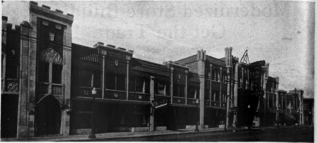
The Lincoln Market Block, Chicago, Shown Above, Is a Fine Example of the Community Store and Office Building. This handsome business block is built of brick with fine terra cotta trim, ornamentation and red Spanish roof tile. Both the Clausen Construction Company and the J. Schworn Company, builders, have offices in this block.
