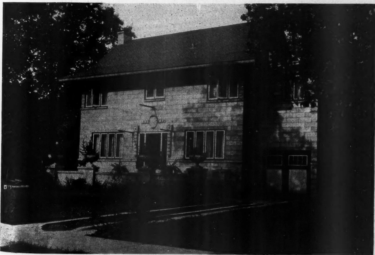
A Fine Type of Concrete Masonry House, with Garage and Sleeping Porch in a Rear Wing. Note the casement windows and fine ornamental effects of the plaisance with concrete flower urns. The portico is not quite complete.
