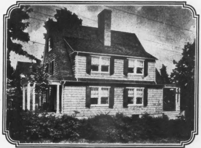
Donn Barber, eminent architect, is quoted in a national woman's magazine as pronouncing this attractive home of John Wise at Relay, Md., "the best small house for its price" among those entered in a recent prize contest. Roof is of WEATHERBEST Green and sidewalls WEATHERBEST Gray Stained Shingles.
