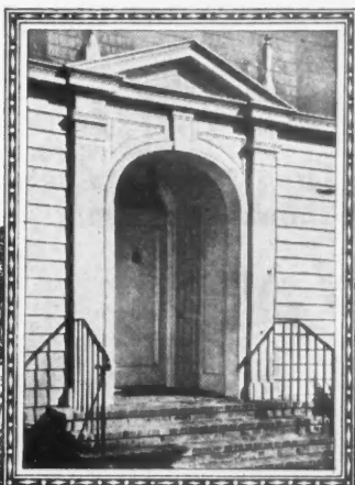
Redwood entrance—124 Santa Clara Ave., San Francisco. Morron and Garren Architects
