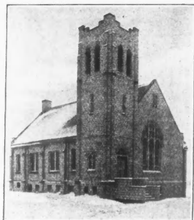
This church completely built of DUNTILE, is typical of the many larger structures for which Albert Dahl & Son are supplying the materials at a cost approximately 30% less than brick.
