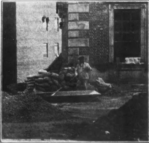
Steel Mortar Box Has Special Advantages.
