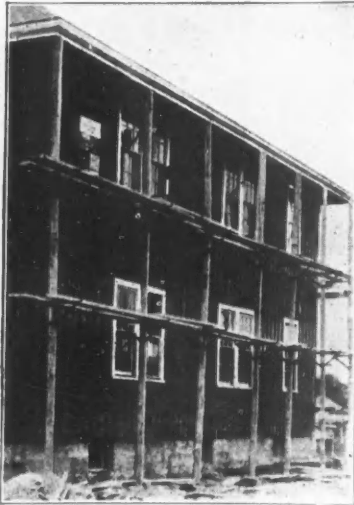
READY FOR STUCCO
