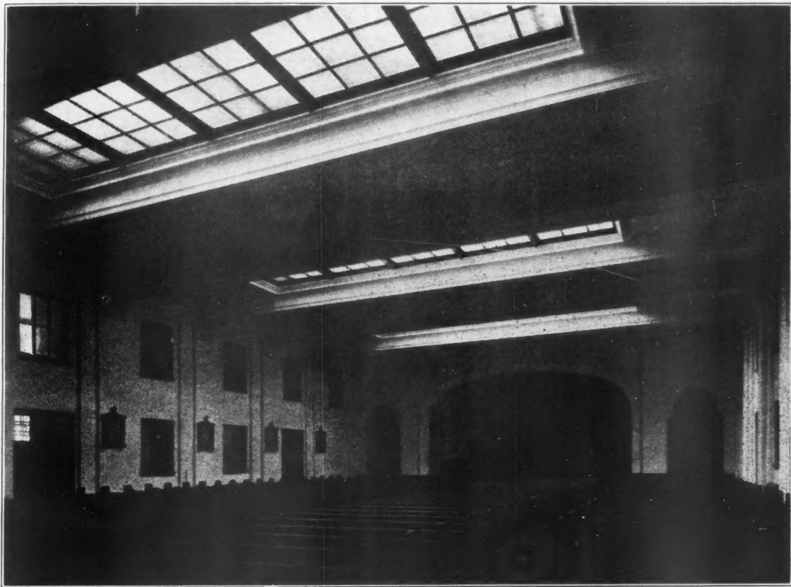
NEW ST. LOUIS UNIVERSITY HIGH SCHOOL, St. Louis, Mo. Barnett, Haynes and Barnett, Architects, St. Louis, Mo. Diffusion of light through Tapestry Glass in chapel. Design appears in lines of clear glass, field sand-blasted.
