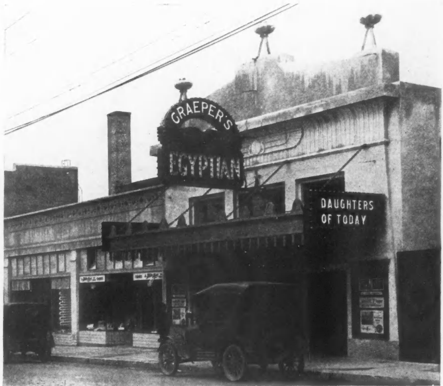
Graeper's Egyptian Theater Shows a Splendid Harmony of Beauty and Utility and Incorporates a Number of Unusual Features. Its speed of construction is a fine example of what can be accomplished by thorough planning of every operation.
