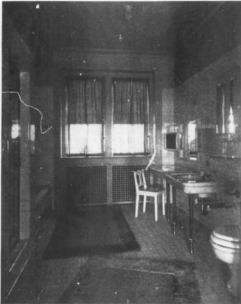
Built-in Bathroom Accessories, Recessed Soap Dishes, Paper Holders and Medicine Cabinets Give an Effect of Substantiality and Luxury and Are Usually Built Into the Walls at the Time the Tile Is Laid.
