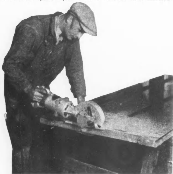
A Portable, Electric, Circular Saw Should Prove to Be a Great Convenience to Building Contractors Because of Its Flexibility.
