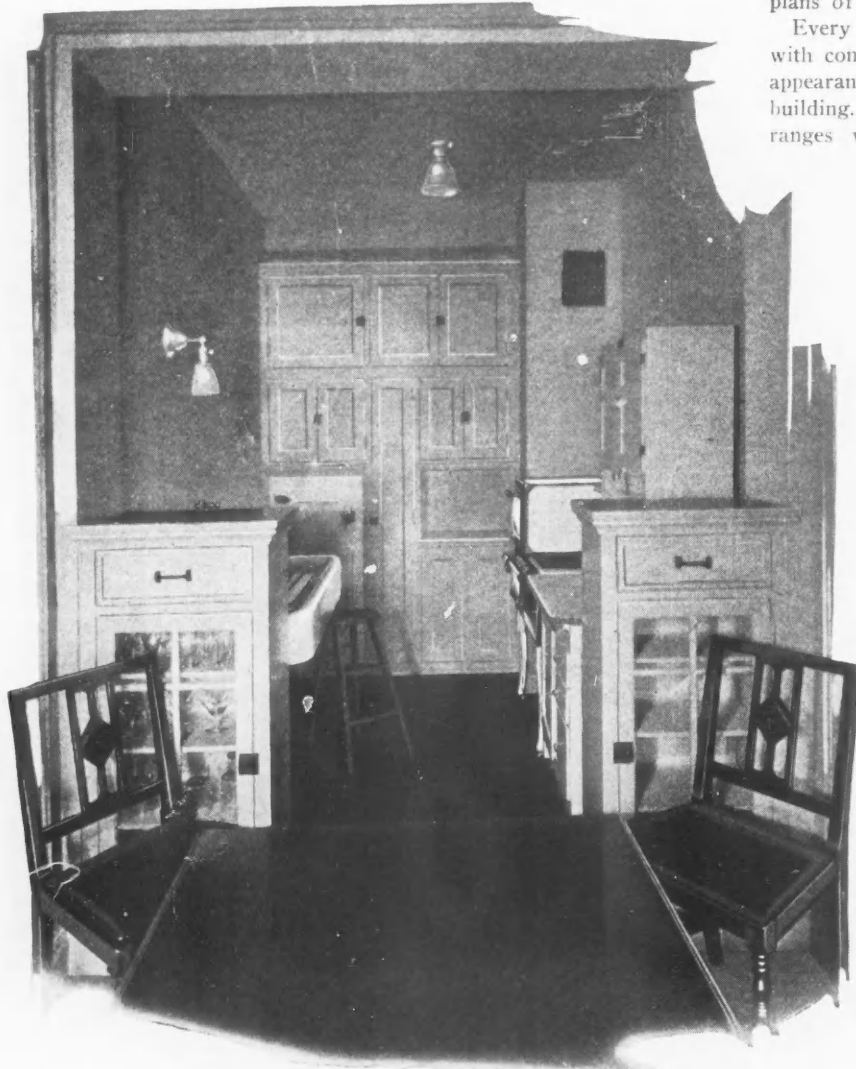
Alden Park Manor Kitchens Are a Fine Example of Compact Equipment Similar to Dining Car Kitchens. Gas range, cabinet, cupboard, ice box and sink are fitted snugly into the least possible space.
