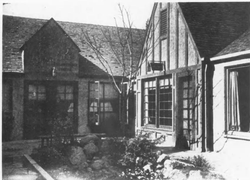
The Restaurant Is Placed in the Rear of the Court, with the Attractive Entrance Shown Here.
