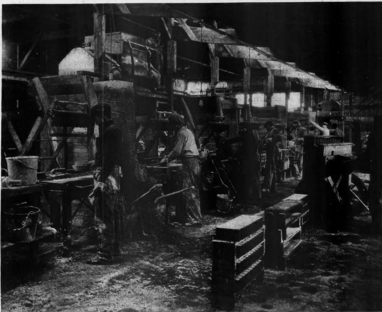
Fig. 5. A Battery of Concrete Brick Machines. At the right is seen a buggy by means of which the brick are conveyed to the curing chambers.
