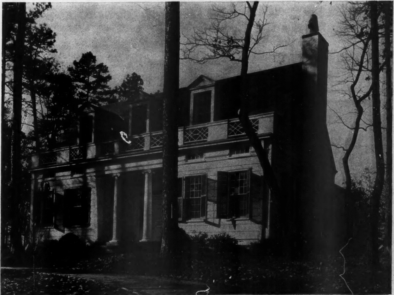
The Colonial Type Home of Mr. Jesse Draper, Atlanta, Ga., Hentz, Reid and Adler, Architects.
