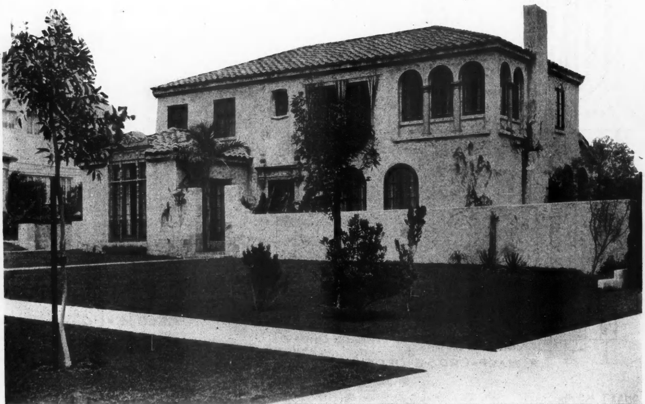
The Attractiveness of Stucco Homes Has Been Enhanced Greatly Through the Increased Attention Paid of Recent Years to the Color Possibilities Attained Through the Use of Mortar Colors and Through the Careful Consideration of the Texture of the Finish of the Stucco. The home shown above has been given a distinct individuality through the use of color complementary to the tile roof and through its rough finished surfaces.
