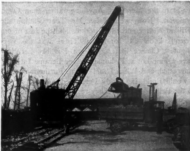
Fig. 8. Loading Concrete Common Brick by Means of Locomotive Crane and Scoop.
