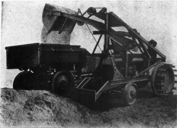
This Equipment, Mounted on a Fordson Tractor, Is Useful to the Contractor for Loading and Digging.
