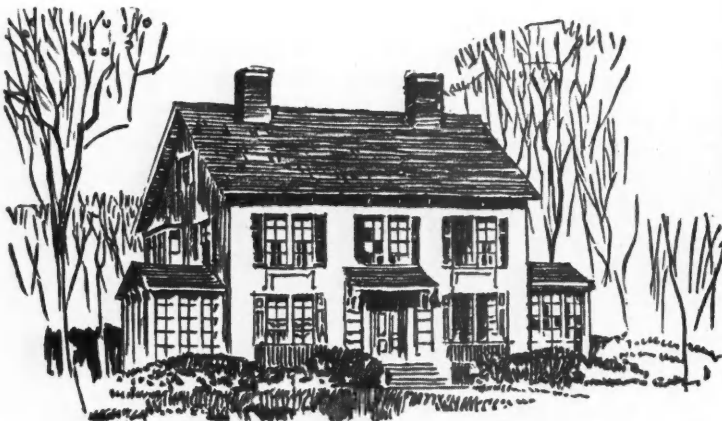
View from Street, Showing Change Effected by Stucco Exterior, New Roof and Sun Porches.
