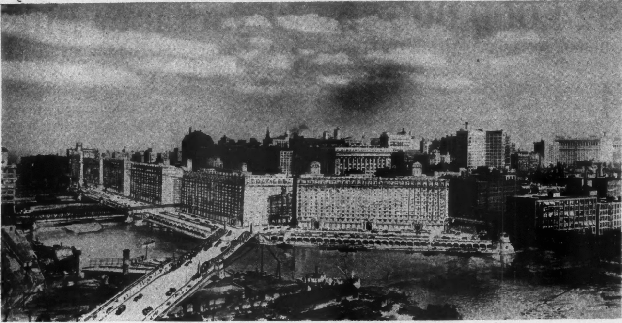
View of South Water Street as It Will Appear When Completed. This perspective is taken from the northwest and shows the street where it turns to the south, following the course of the Chicago River. Notice the facilities given for docking the lake steamers through the double street level.
