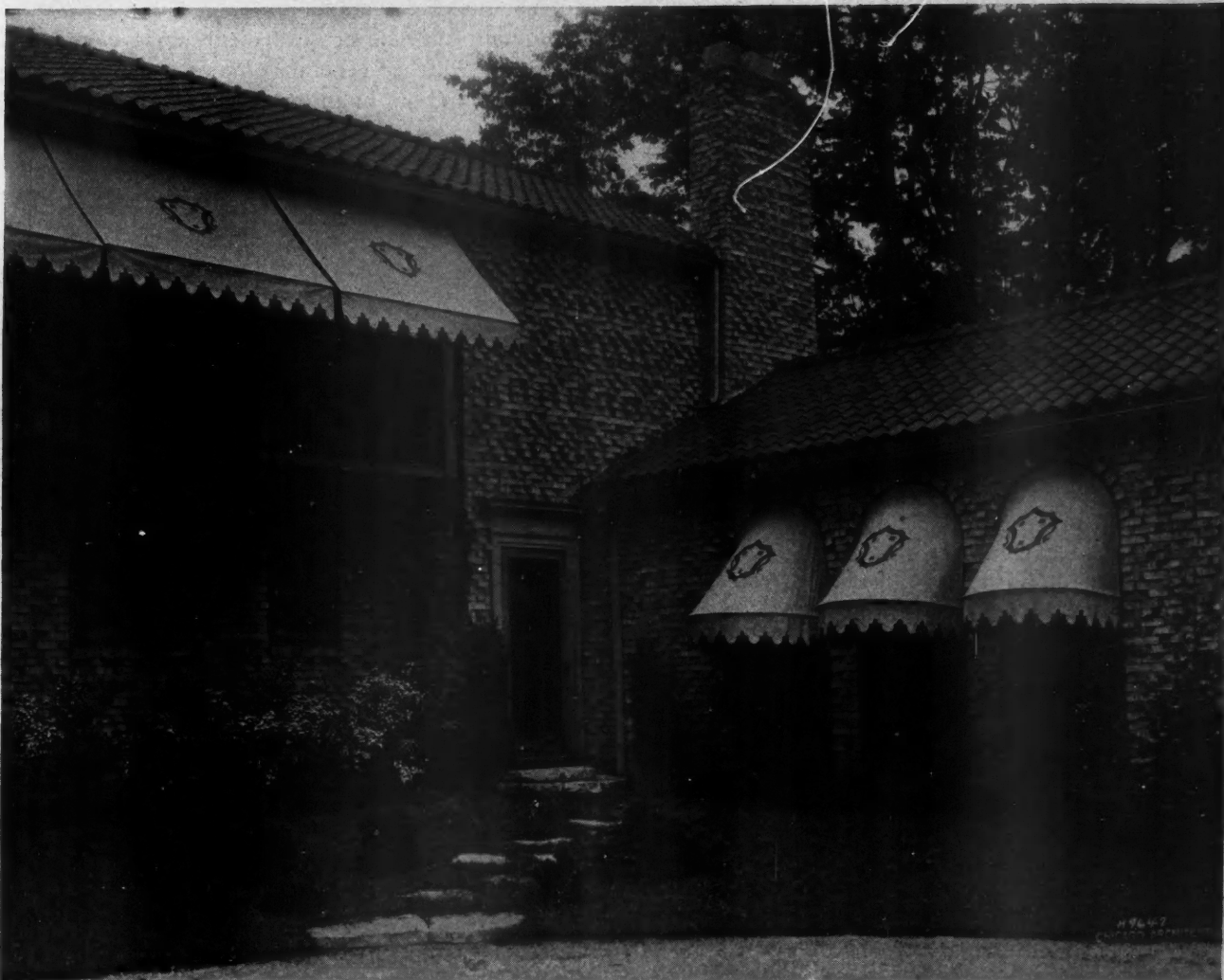
Effect No. 5, Described in this Article, Illustrates the Attractive Residence Walls Which Are Constructed Through the Irregular Placing of Common Brick. The panel above shows the details of the manner in which the brick are laid.
