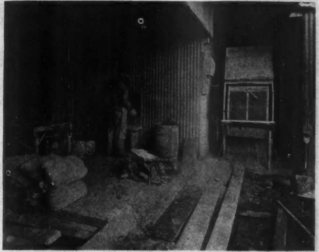
Fig. 2. Unloading Sacked Cement into Cement Bin from Which it Flows Through Measuring Device to the Mixer. The bag cleaner is shown at the right.
