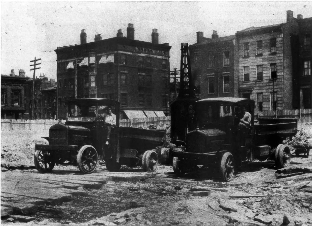
Contractors' Trucks Must Meet Unusual Conditions, Off the Paved Roads, That Entitle Them to Especially Good Care.
