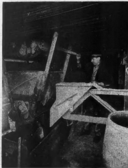
Fig. 3. Large Steel Bucket Over Mixer Measures the Aggregate from the Material Bins Above. Smaller hopper at the right has just tilted down from a position under the supply bin further to the right.
