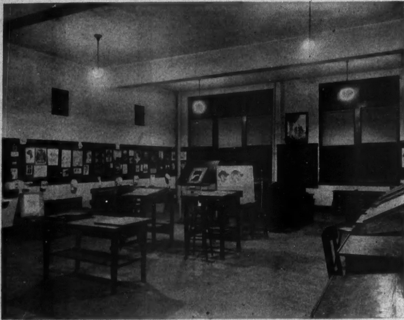
An Average Foot-Candle Intensity of 9.5 Is Provided on the Tables by This Style of Direct Lighting. The lamps are 200 watts each. The Milwaukee Trade School.
