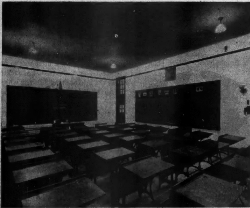
In This Example of Direct Lighting, an Open Reflector Is Used to Good Advantage—Geo. C. Thomas High School, Philadelphia.
