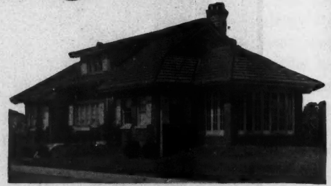
A typical example of single floor home.
