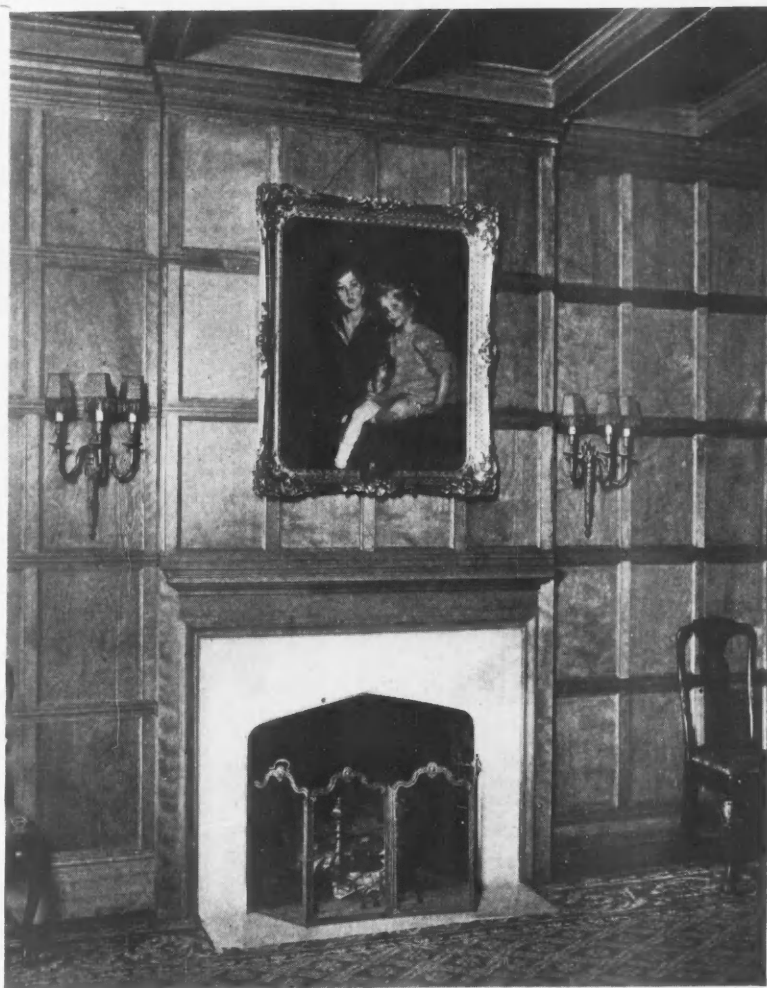
Panelled Walls and Beamed Ceiling of Birch in the Dining Room of Mrs. Minturn Pinchot, New York. Wood has been stained but slightly and waxed, giving a delightful, warm tone. Murphy & Dana, New York, architects.
