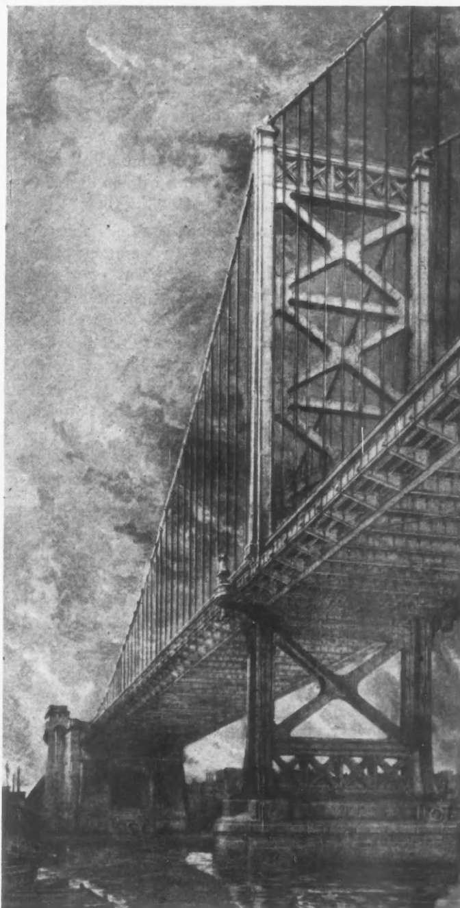
The Bridge is of Simple But Beautiful Design, and a Total of 33,000 Tons of Steel Used. It is expected to have it completed July 4, 1926, for the Sesquicentennial of the Declaration of Independence at Philadelphia "World's Fair."
