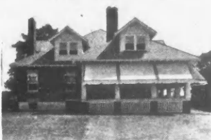
Residence of Abbott Worthley, Bradevelt, N. J., Fred Jennings, Freehold, N. J., contractor.
