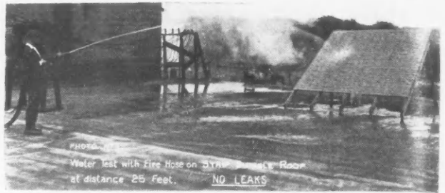
Testing Panel with Fire Hose at 25 Feet—No Leaks.
