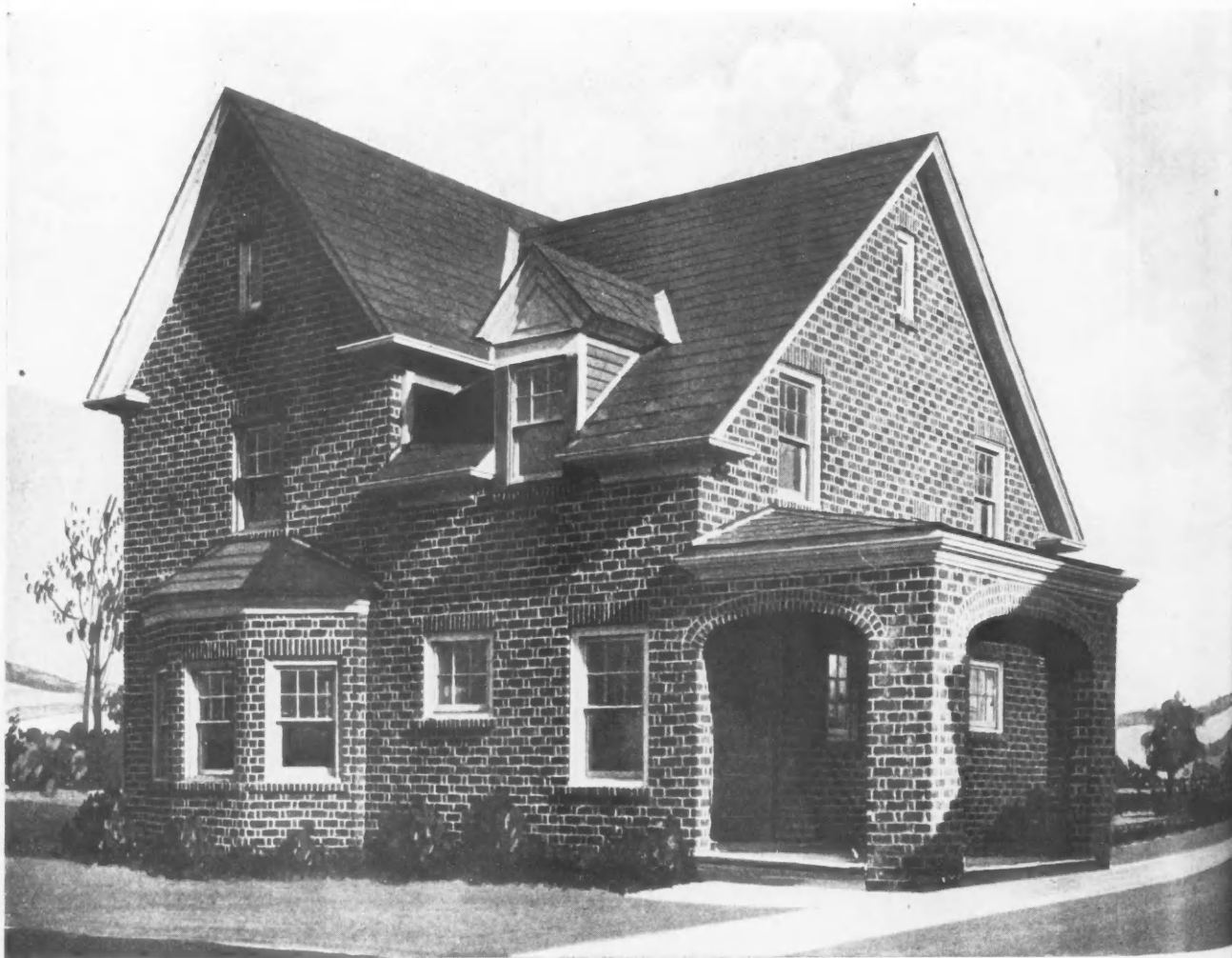
Ideal Wall Home, Built with 8-Inch Walls, at Phillipsburg, N. J., Paul R. Smith, Architect.
