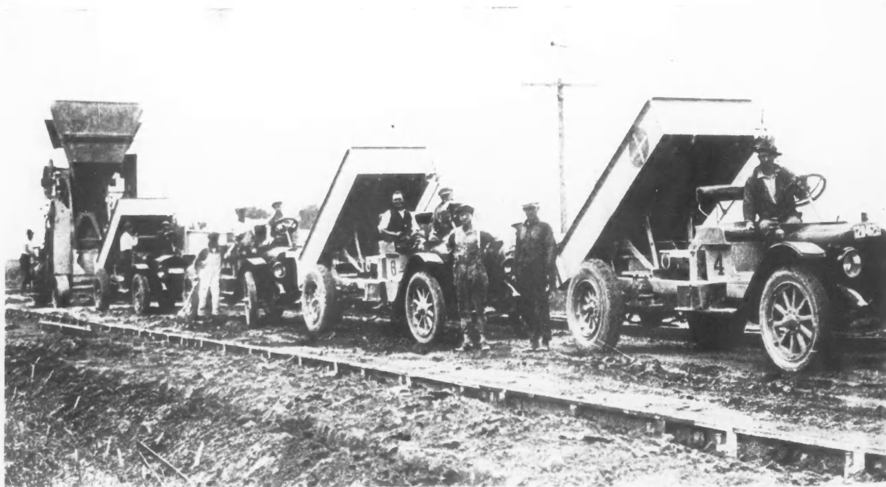
Fleet of Two-Ton "Whites" Used by Johnson, Drake and Piper, Contractors, on a Fifteen-Mile Project Near Minneapolis, Minn. They Averaged 600 Feet a Day for Two Weeks.
