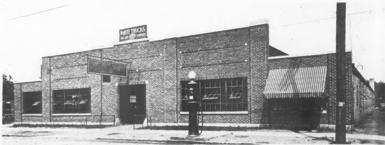
Lorenz Brothers, Lansing, Mich., Appreciate Sturdy Simplicity. Steel Sash and Simple but Attractive Brick Treatment Answered Their Desires.
