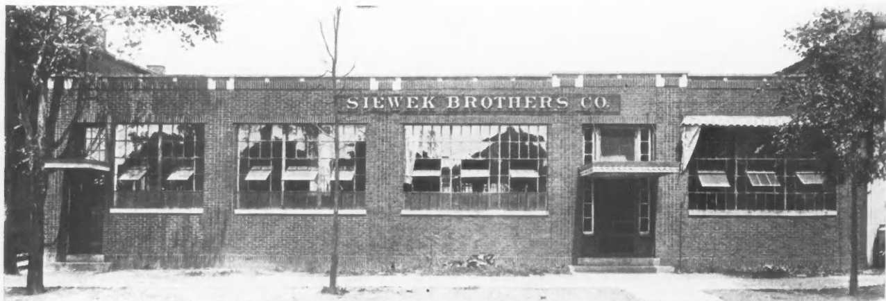
A Commendable Example of a Well Lighted One-Story Factory and Office Building. Steel Sash Was Used Thruout the Building.
