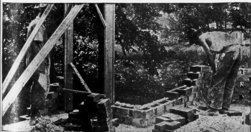
Note the sturdy construction of the Ideal All-Robk Brick Wall, with its 2½ inch webs and ventilated air space
