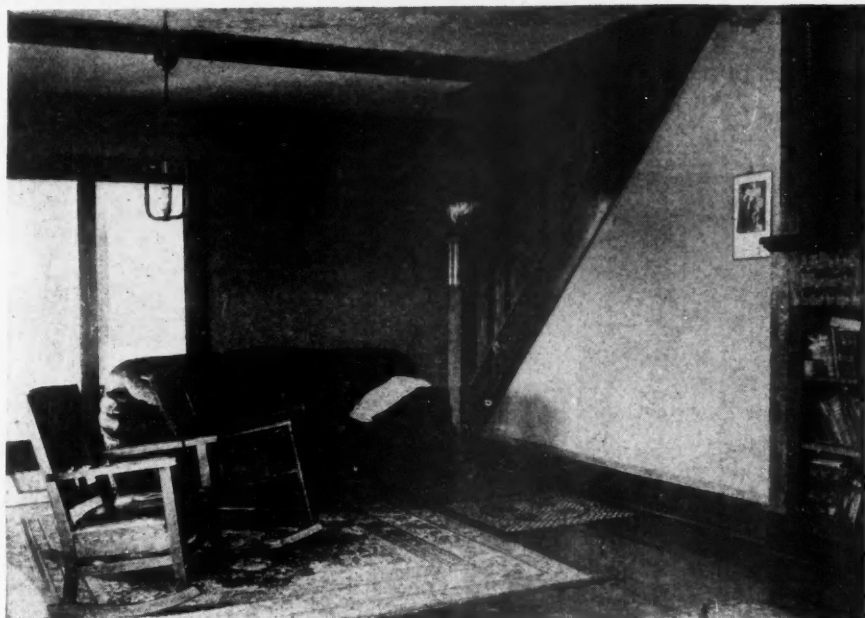
Actual View of Register in Living Room of Shinn Home. The Warm Air Rises and Passes Up the Stairs to the Rooms Above. It Also Circulates Thru the Living Room and Then Into the Other Rooms Connecting.
