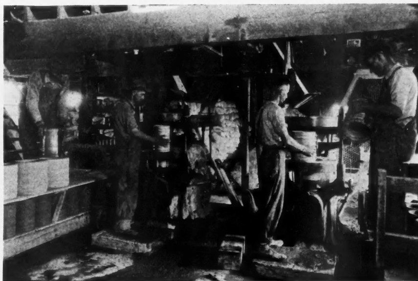
Five Men Operating Tile Plant at Thiensville, Wis. Mr. Melxner, President, Believes in Concentrating on a Quality Product and as a Result Has Built Up a Profitable Business in Very Short Time. Note the Chutes from the Material Bins Feeding the Machines.
