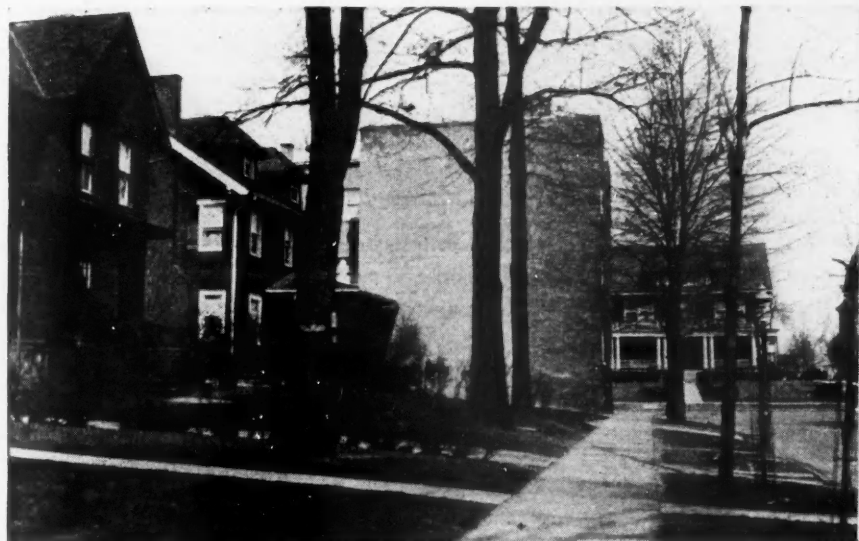
Another Glaring Case of Incongruity in Building. Carefully Planned Zones Will Eliminate Such Undesirable Features.
