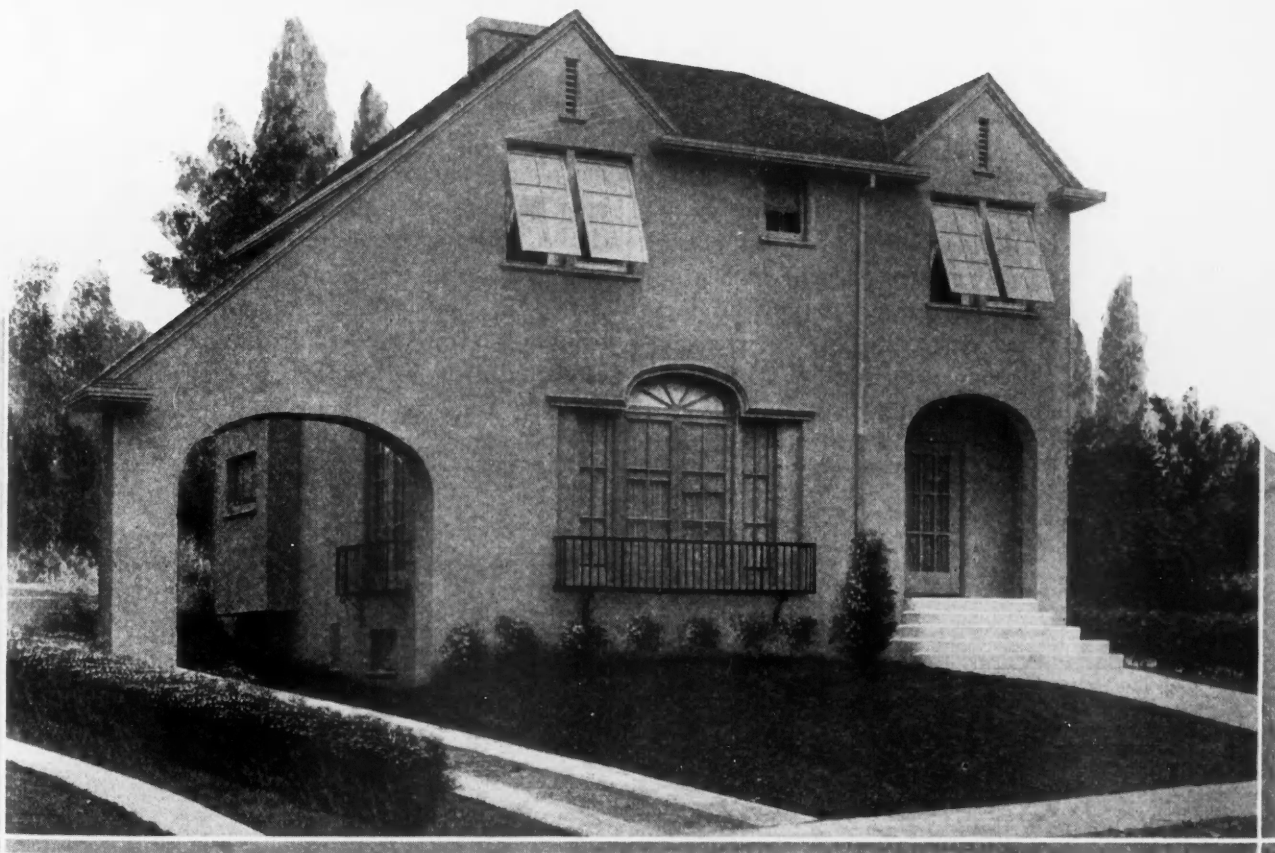
PLEASING HOME OF UNUSUAL AND DISTINCTIVE DESIGN. Architecturally, this house is in a class by itself because of its odd lines and arrangement. It is built of hollow tile with a stucco finish, and at first glance looks to be a double house similar to many found in the east. But it is built to satisfy a home owner who wants something out of the ordinary and at the same time substantial. Particularly striking is the extension of the front wall to form an arch over the side driveway. The plans call for seven rooms, three on the first and four on the second floor. The living room is 18 by 15 feet 6 inches with French doors in front and side opening out into small balconies with artistic iron railings. The entrance to the living room is arched similar to the outside front entrance. A breakfast nook and extra toilet on the first floor should be noted. Four bedrooms are located above. Size of house, 31 feet square.
