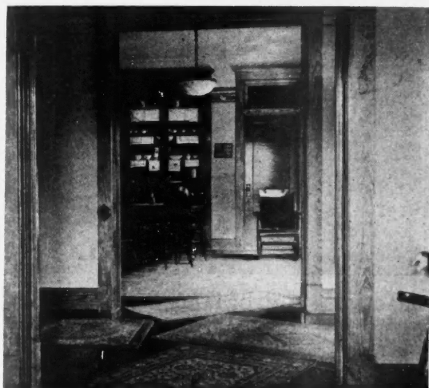
Hall in J. L. Ewing Home, Evansville, Ind., Showing Pipeless Furnace Register Properly Located. This Is One of the Important Parts of the Furnace Job.
