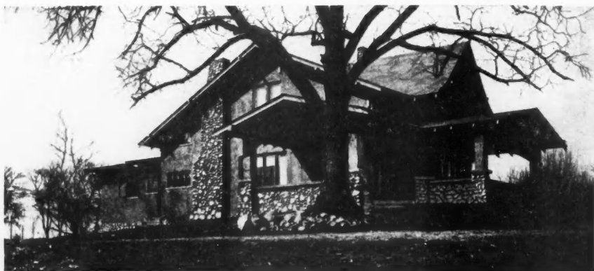
Home of Walter Shinn, Peru, Ind., Which Is Equipped with Modern Pipeless Furnace. Building Contractors Have Installed Many Furnaces of This Type During the Last Five Years.
