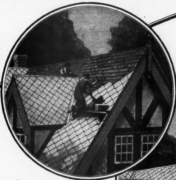
Re-roofing for the last time with Johns-Manville Asbestos Shingles.
