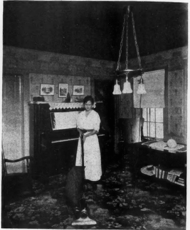
Now It Is Different. Electrical Power, Furnished by Plants or Power Lines, Have Transformed this Home and Made the Wife Younger by Many Years.
