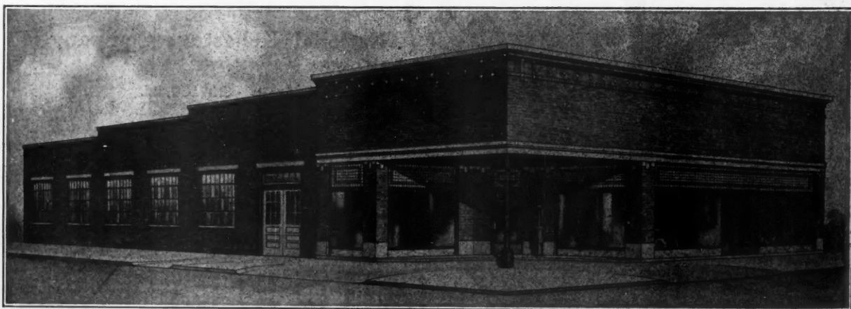
A modern garage featuring a gasoline filling station under the corner of the building. Floor plan of this garage sent upon request
