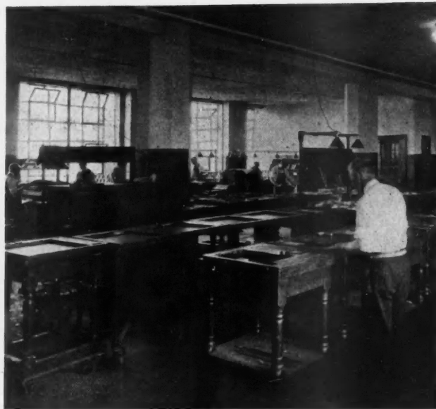
Special Steel Sash in the Work Rooms Insure Plenty of Natural Daylight which is Essential to the Printers. This Floor is Composition.
