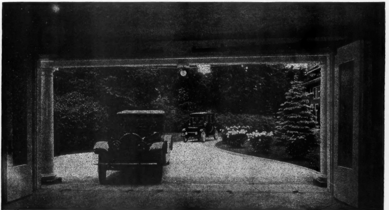
Entering the Garage After the Daily Spin. The Doors Painted White with Narrow Glass Panels Are Swung Back Against the Wall. Note How They Slide Along an Overhead Track Above the Door.
