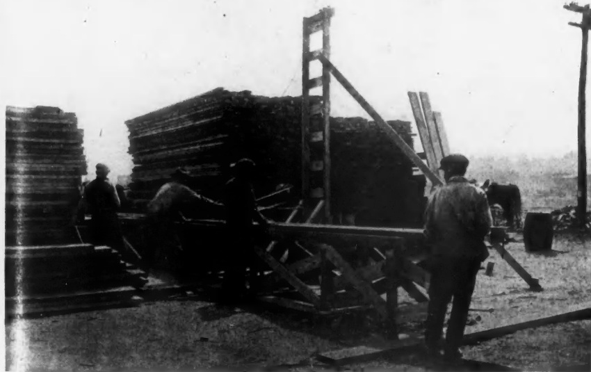
Power Saw Rig Is Called Into Action to Speed Up Building of Monster Stadium for World's Championship Fight at Jersey City, July 2. This Structure Is to Be Built in Eight Weeks.
