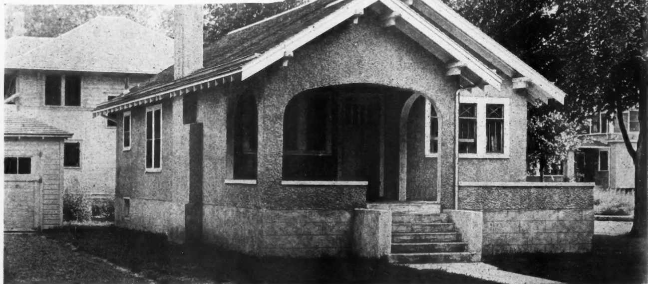
Home No. 5. Stucco and Concrete Block Help to Make This Five-Room Bungalow Attractive. It Is Substantially Built and Very Comfortable. Floor Plan Above.
