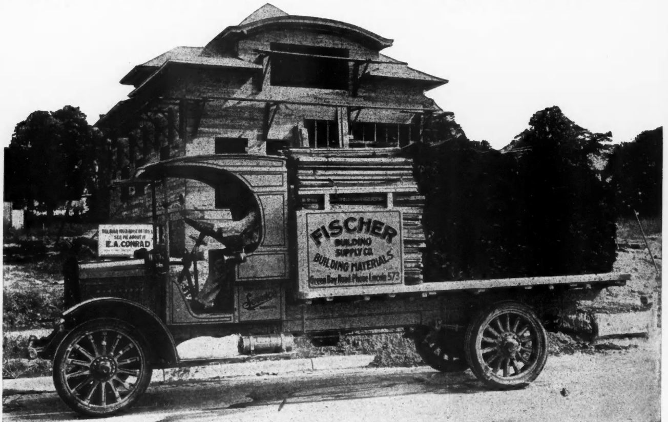
Getting Supplies to the Job in Time Is the Big Function of This "Service" Truck. The Fischer Building Supply Co. Find It Keeps Their Customers Satisfied Because They Are Not Held Up Waiting for Material.
