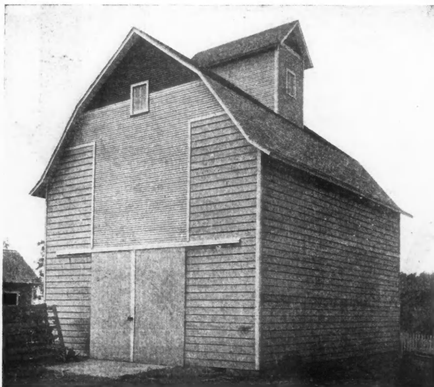
Substantial Frame Corn Crib and Granary of Type Popular in Corn Belt. It Is Equipped with Inside Cup Elevator and Rat-Proof Concrete Floor. Bins for Grain in Addition to the Corn Cribs Are Provided.
