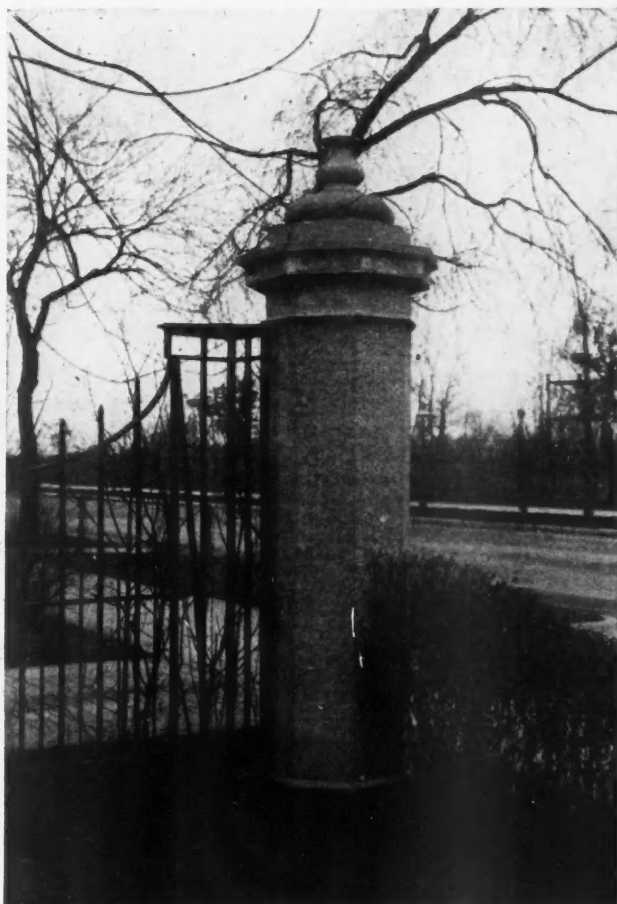
Figure 4. City and Suburban Homes Are Made More Attractive by Simple Gate Posts of Dignified Design and Elegant Surface Texture. The Shaft Shown in this Illustration Has a Coarse Colored Aggregate Surface, Acid Washed.
