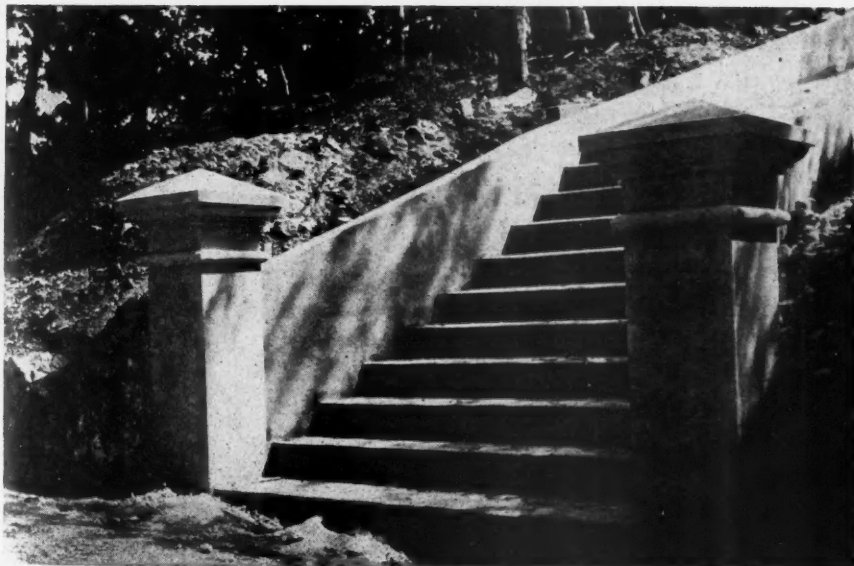
Figure 1. Plain Square Posts with Surfaces Mortar-Filled and Painted with Creamy Mixture of Ordinary Cement and Water.
