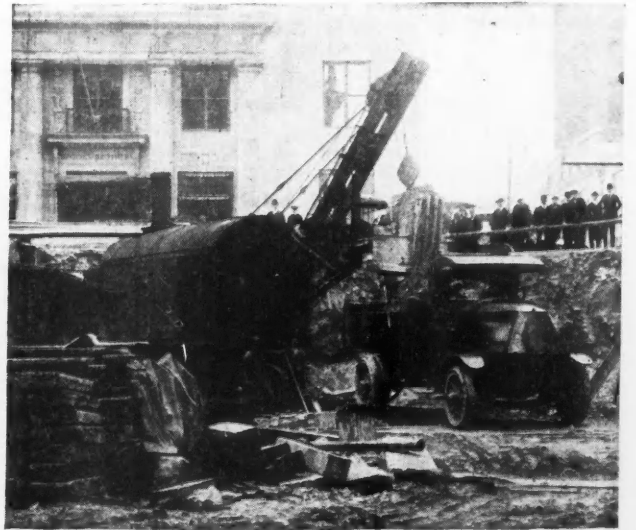
Excavation Work Is One of the Test Jobs for a Motor Truck. This Giant "Mack" Is Taking on a Load. Mr. Ferger Keeps His Trucks Going Day and Night on Work of This Kind.
