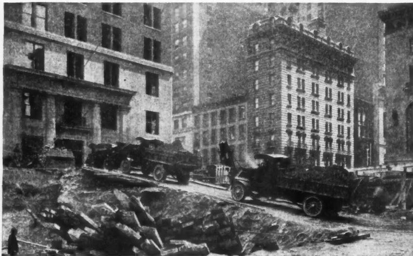
Keeping the Trucks Busy the Year 'Round Is the Secret of the Contracting Business According to L. Ferger, a New York Contractor. When the Building Business Is Slack He Does a General Hauling Business and Thus Keeps a Fleet Going at Top Speed.
