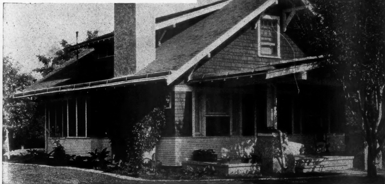
Home No. 3. Pleasing Cottage Bungalow Built on Economical Lines. Several Space-Saving Features Have Been Used to Cut Cost. Floor Plan in Upper Left Hand Corner.
