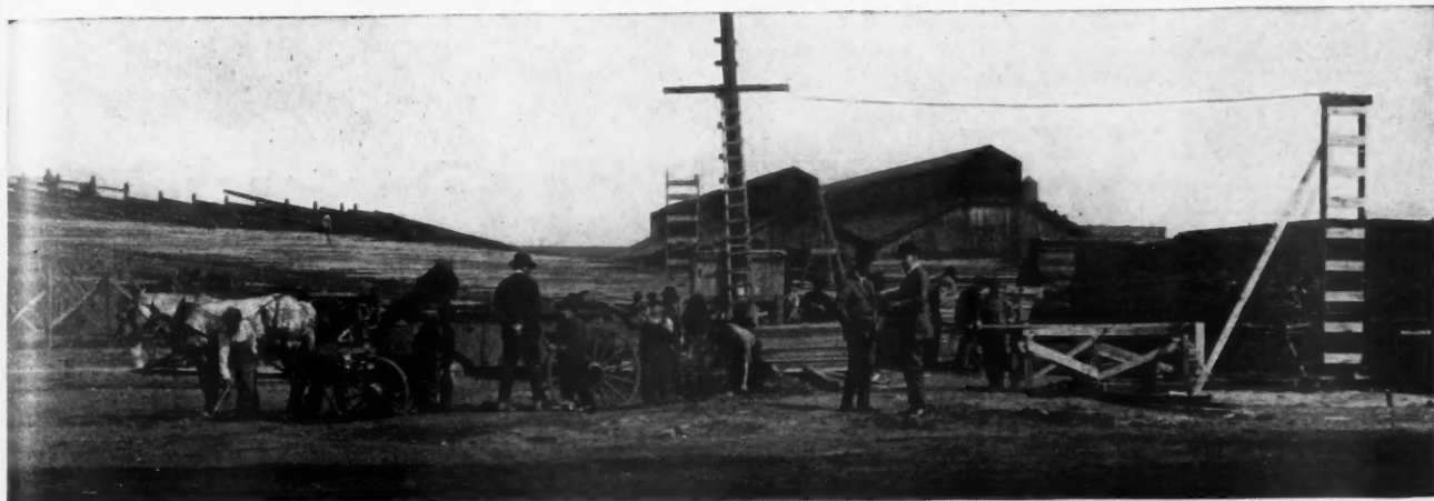
Gradually Taking Form. This Stadium Will Hold 60,000 People When Completed. It Requires 2,000,000 Feet of Lumber and 13 Tons of Nails.
