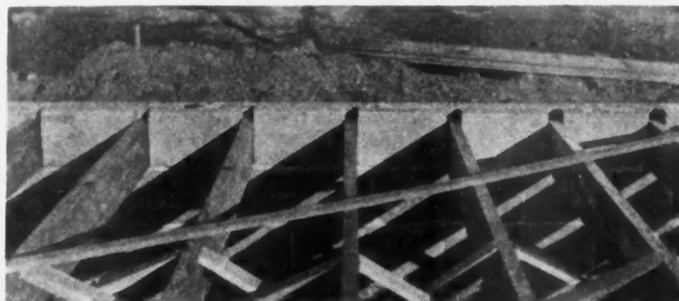
Figure 3. Method of Seating Floor Joists. The Joist Block Filling the Space Between Joists on the Inside of the Wall, Are Clearly Shown.
