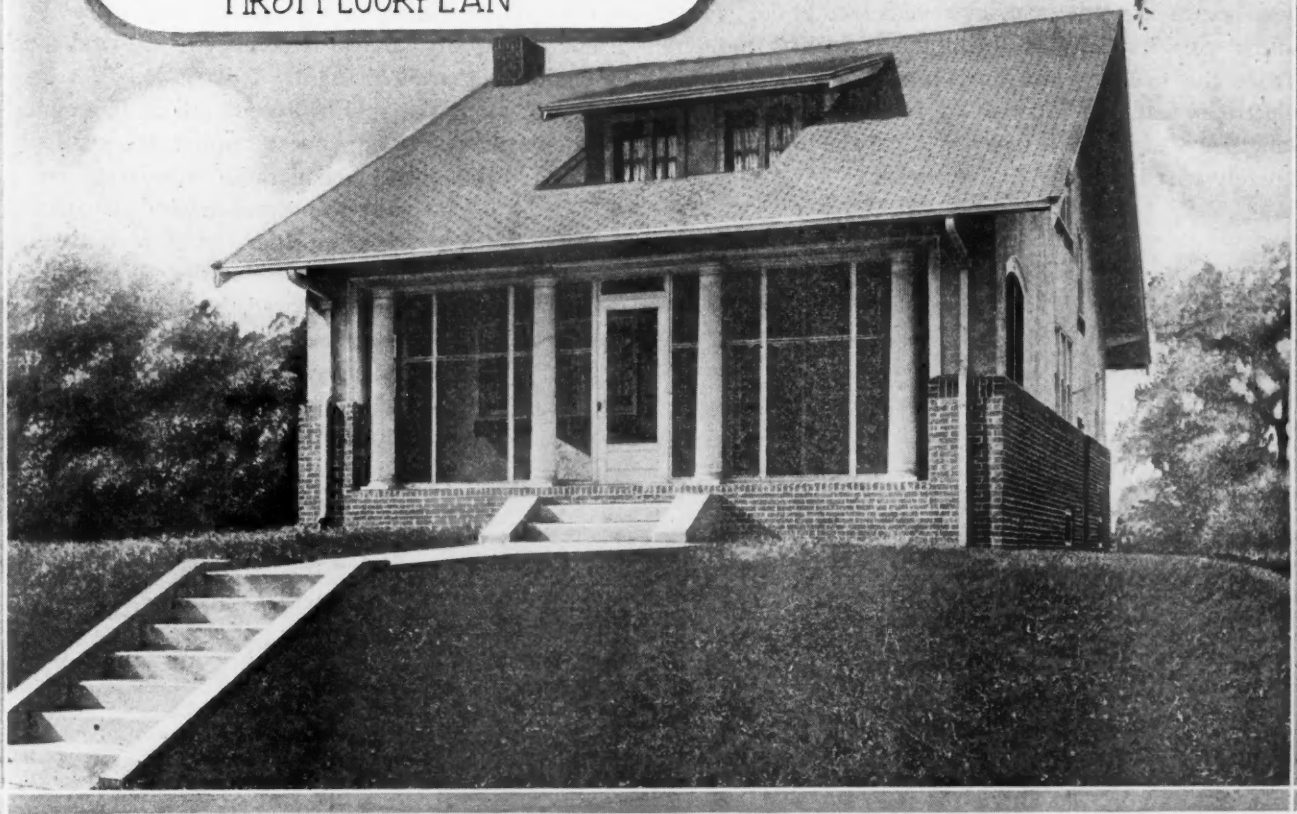
COZY STORY-AND-A-HALF HOUSE OF SIMPLE BUT PLEASING DESIGN. This appealing little home is built of brick and stucco, the brick extending about half way above the first floor line. The house is set back on a terrace and reached by concrete steps. The front porch extends the full width of the house and is screened in for the warm months. On the first floor are living room, dining room, kitchen and a large combination pantry and work room. The living room is 15 by 12 feet 6 inches, with brick fireplace and wall bookcase on the outer walls. The kitchen and pantry have been equipped with many modern labor-saving conveniences, such as hinged ironing board and refrigerator for outdoor icing. On the second floor are two bedrooms of good size, well lighted by windows in the roof dormers in front and rear, modern bathroom and a small alcove. The balcony floor has been covered with canvas flooring. Size of house, 36 feet 10 inches by 26 feet 10 inches.
