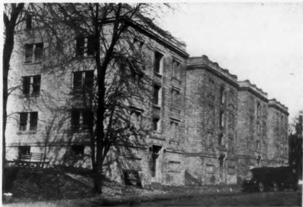
Figure 7. The Aberdeen Apartments, Nearing Completion, Have All Exterior Walls of Concrete Block and Concrete Architectural Trim, Using the Bedford Finish. The Rear and Side Elevations Are Practically as Attractive as the Front.
