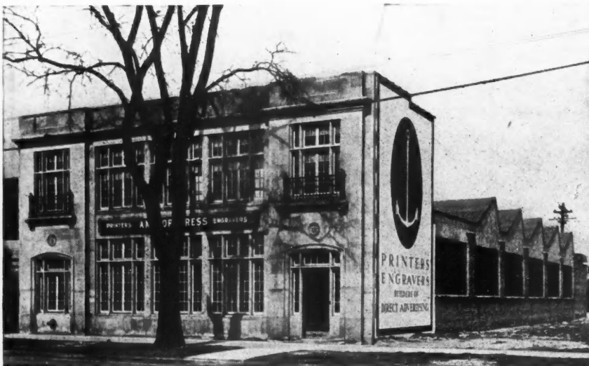
New Plant of Anchor Press, Detroit, Mich., Built Along Latest Lines in Factory and Shop Construction. Note the Splendid Natural Lighting Facilities Provided by Walls of Windows. Frederick J. Winter Was the Architect.
