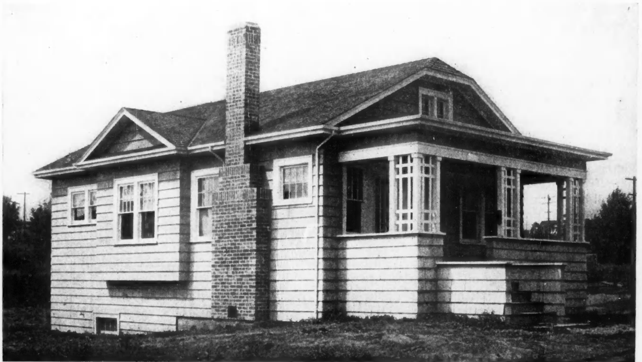
This Is the House as Built at a Saving of $720. Space Saving Closets and Kitchen Units Eliminated Much Waste Space and Saved 202 sq. ft. as Shown in the Comparative Floor Plans on the Next Page.
