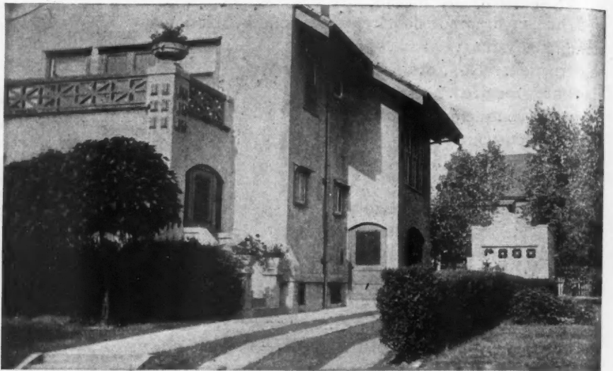
View of Ahnfelt Home, Chicago, with Combination Block and Stucco Garage in Rear. The Garage Was Designed to Harmonize with the Residence. Judge the Results for Yourself.
