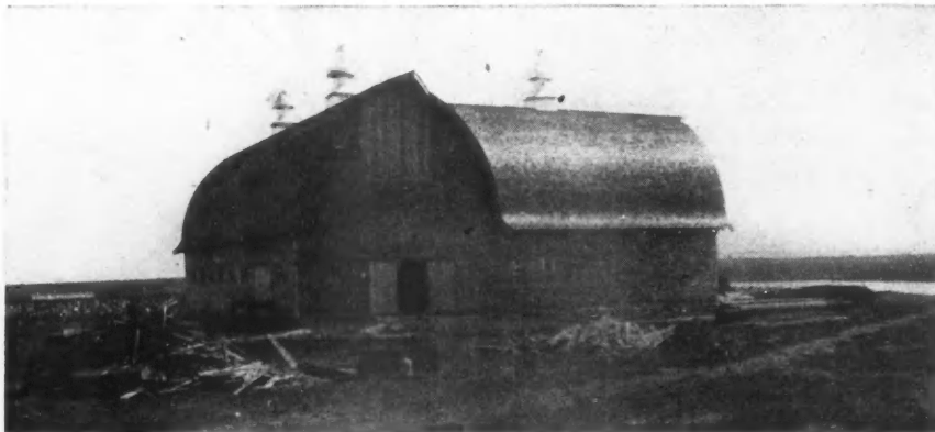
Large Barn Built by Geo. M. Gunderson, Havana, N. Dak. Note the modern Ventilators on the Roof and Gothic Type Roof.
