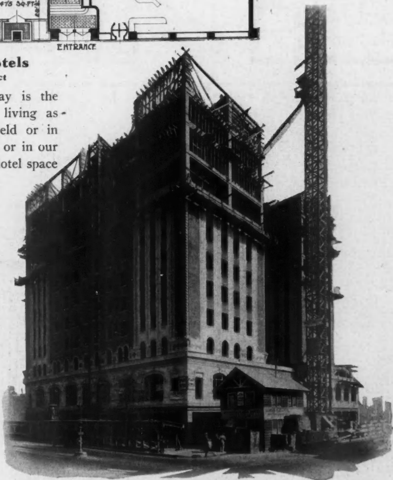
The Sheridan-Plaza During Construction. The Concrete Is Being Poured for the Reinforced Framework of the Upper Floors, While the Masons Are Following Close Behind With the Brick and Terra Cotta Walls. Executive Management of a High Order Is Required for the Co-ordinating and Speeding Up of a Construction Enterprise of This Character.
