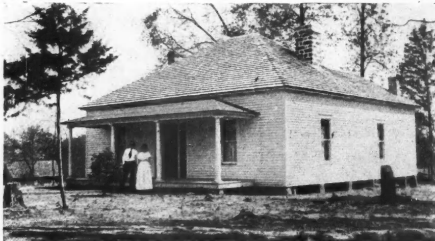
Joe Masters, Builder at Hilham, Tenn., Built This Home and Several Others Down in That Vicinity. He Reports Unusual Activity. The Cost of This Building Was $2,000.
