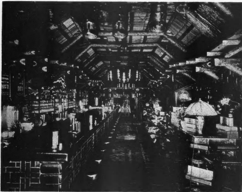
Fountain and Counter of Establishment. The Walls Are Covered with Bark Set in Upright Sections While the Ceiling Is of Modified Chapel Design and Well Suited for Heavy Beams and Braces.
