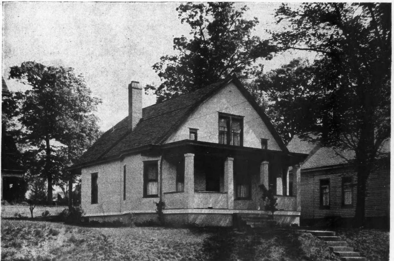
After. The Same Home After It Had Donned Its New Suit of Special Stucco. It Is Used Over Wood or Metal Lath. The Value of This Home Has Increased Considerably Thru This Operation Which Is Carried Out at a Low Cost.
