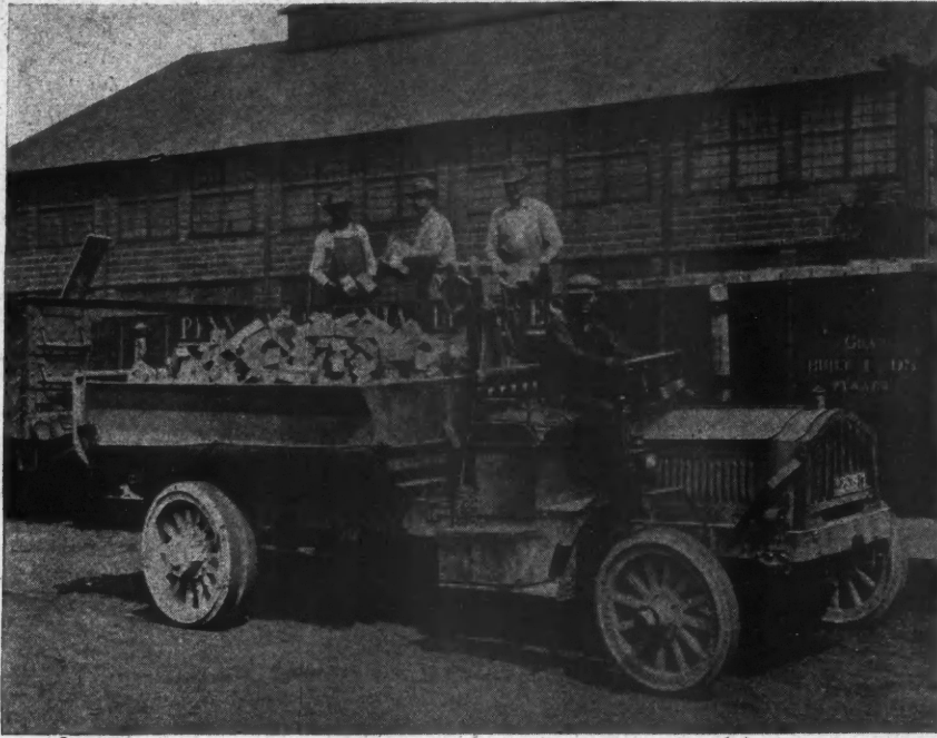
Five-Ton "Packard" Doing Its Bit in the Big Building Campaign. The Dump Body Has Eliminated Much of the Delay Connected with the Unloading of Brick. The Large Hauling Capacity of This Truck Cuts Down the Number of Loads for a Job.
