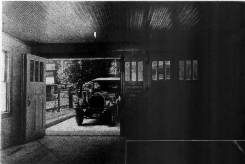
Combination Folding and Sliding Door Set Made Up of Six Doors. The Two Middle Doors Swing on Hinges to Make an Entrance. Each Set of Three Fold Up Accordion Fashion and Slide to the Side of the Doorway.
