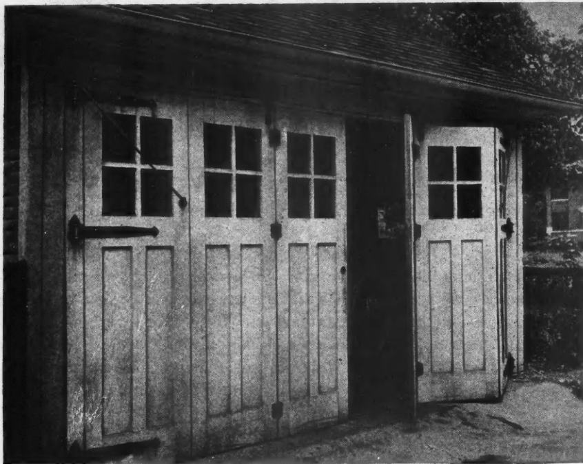
Combination Folding and Sliding Doors Opening Out Instead of Inside. These Doors Are Made in Sets of Three to Ten Doors and Are Designed to Fit Garage Doorways Ranging from Eight to Thirty Feet. This Picture Gives a Good View of the Hanger Equipment.
