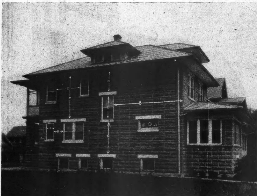
Fig. 2. Elevation of Concrete Block House Showing Dimensions "B" Conveniently Computed by Means of Curves Shown in Fig. 3, Dimensions "C" Computed Similarly by Means of Curves Shown in Fig. 4.
