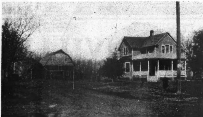
"Chips of the Old Block." Mrs. Wm. Neumeister's Three Sons Have Taken Up the Building Profession, Following the Footsteps of Their Father. This Picture Shows a Group of Farm Buildings Which They Built at Scotland, S. D.
