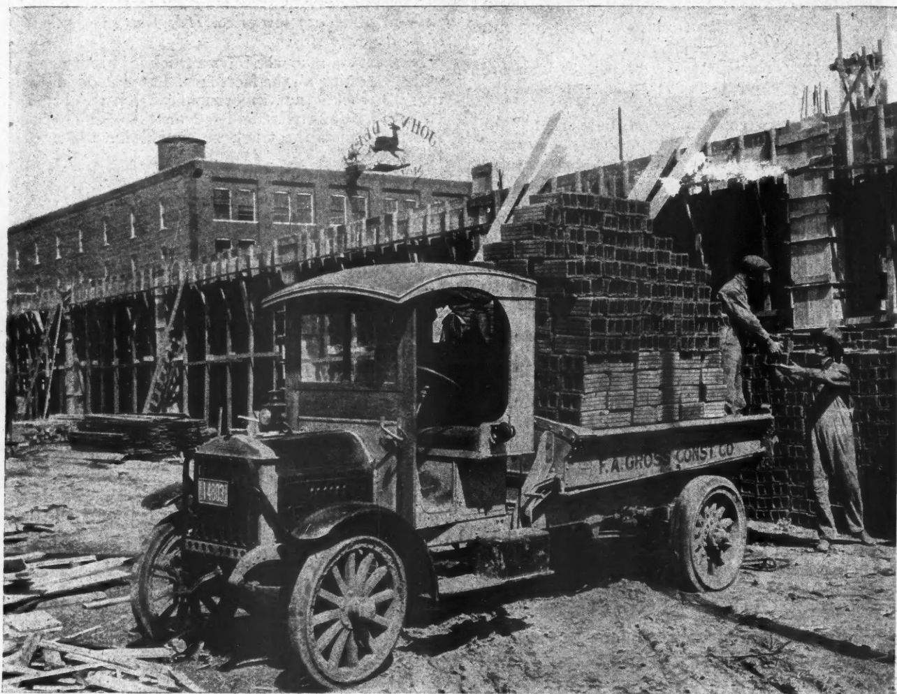
Carrying a Little More Than Its Share. This "Federal" Truck Does Not Believe in Rest as the Size of the Load Shows. In Fact It Is Ready to Work Just a Little Harder Than Usual to Make Up for Lost Time. The F. A. Gross Construction Co. Keep Their Men Supplied with Material All the Time.
