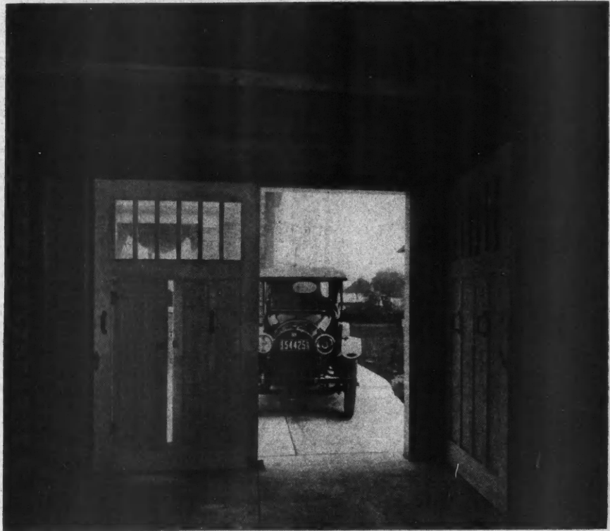
Right Angle Doors as They Appear from the Interior of the Garage. This Picture Shows the Track Arrangement, also the Wicket Door, Which Is Very Convenient in Getting in and out of the Garage. The Space Saving Accomplished by This Type Is Apparent.
