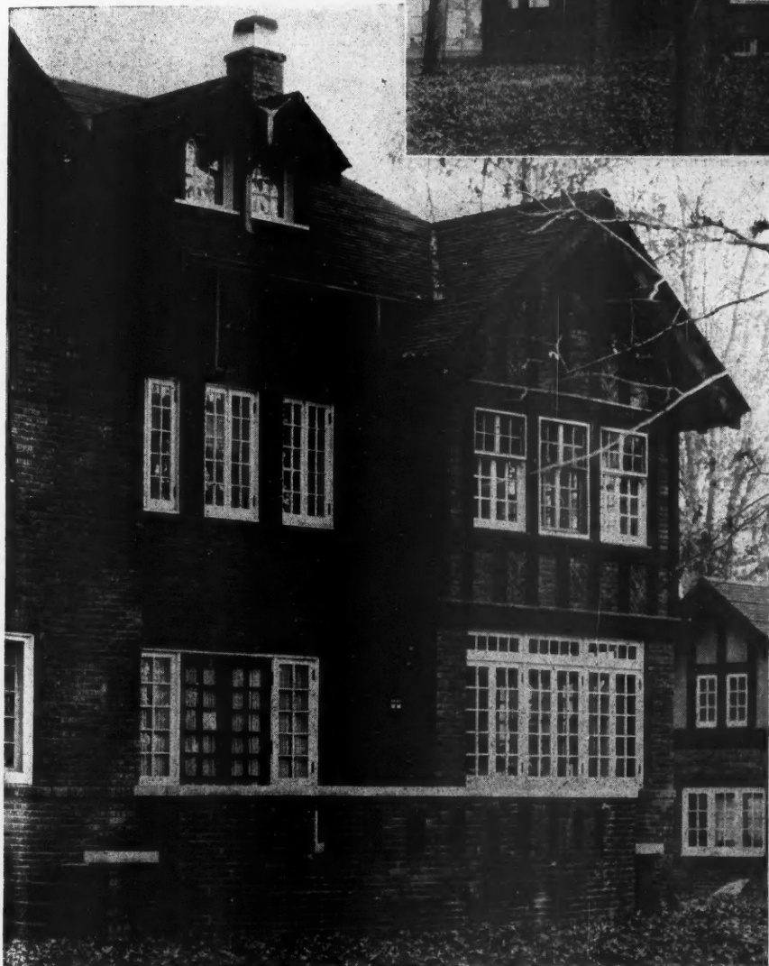
Close-Up View of Brick House, Showing Face Brick Construction. The Variations in Panel Patterns Can Be Seen Clearly Between the First and Second Floor Windows of the Sun Porch.
