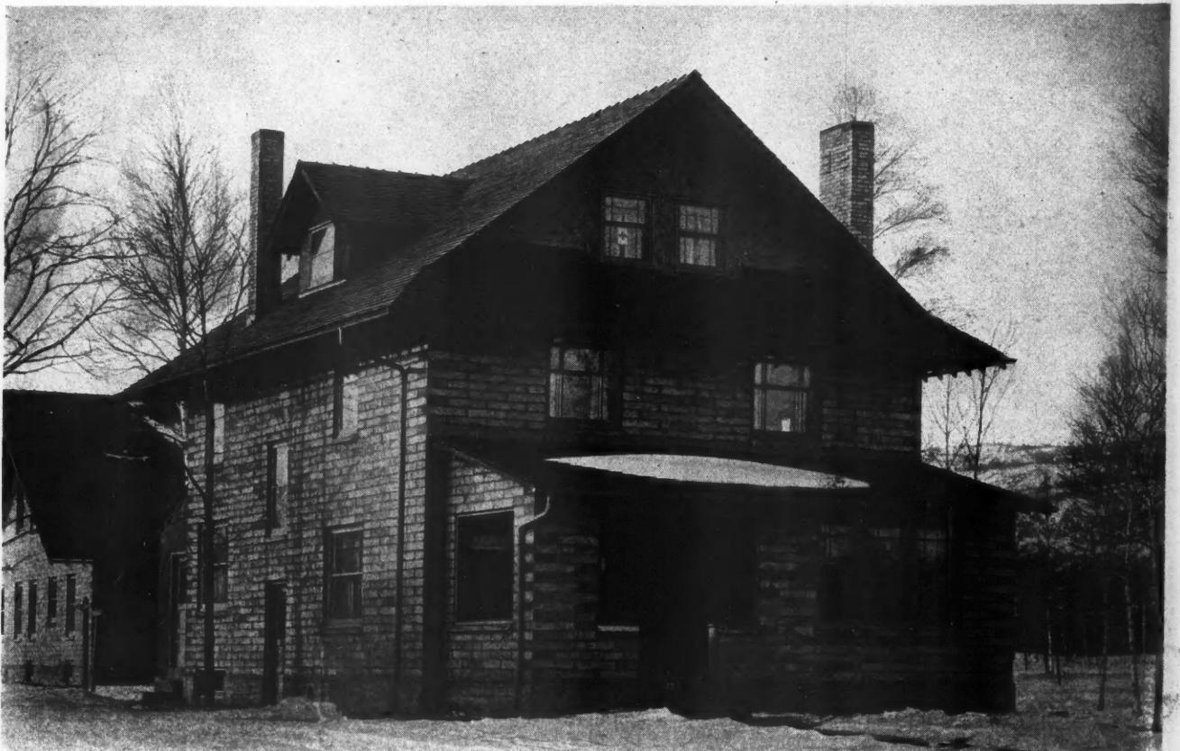
Front View of Concrete Block House Described in the Accompanying Article. The Plain but Good-Looking Practical Home for the Family Requiring Ample Bedroom Space.
