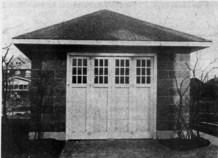
Concrete Block for a Structure Like This Can Be Made Up in the Dormant Winter Season and Hauled by Motor Truck to the Job. The Hip-Roof Effect Is Very Popular in Garage Construction.
