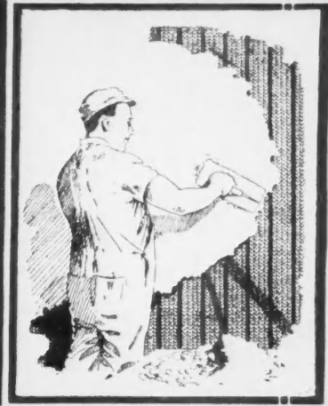
METAL LATH USED FOR SUSPENDED CEILING
