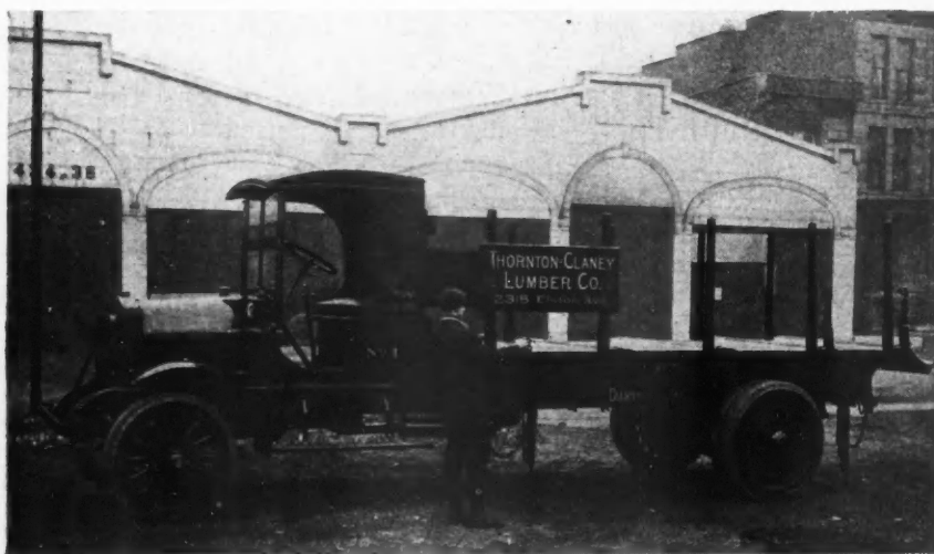
One of the "Diamond T" Fleet Operated by the Thornton-Claney Lumber Co., Chicago, Ill. Note the Special Equipment for Unloading and Body for Carrying Long Timbers. Two Trucks Like This One Hauled Lumber at an Average Cost of $1.53 Per Thousand.
