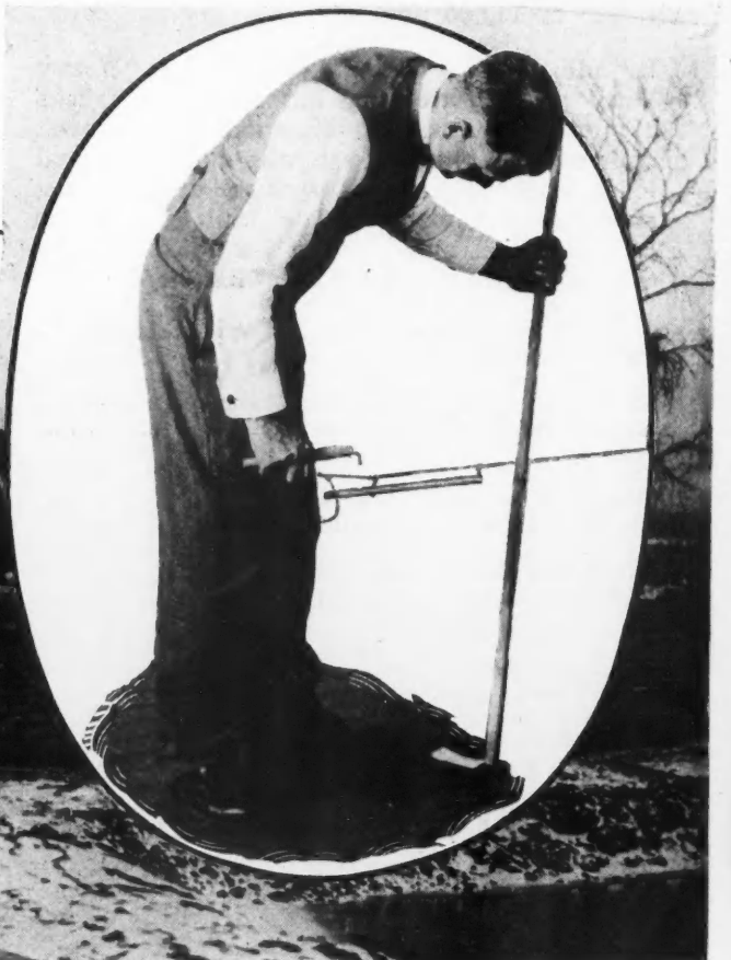
A Level Is an Essential Instrument on the Job. It Gives the Proper Lines and Enables the Workmen to Keep the Walls True. Insert Shows How Levels Are Secured by the Use of a Line Level.
