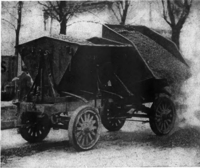
Side Dumps on Trailer Speeds Up Building Work by Eliminating Unloading Delays. These Side-Dumps Are Very Delicately Balanced and Can Be Tilted by Hand. This Truck Can Carry Two Kinds of Material.
