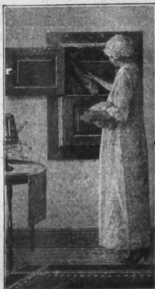
This Housekeeper Is Not Disturbed by the Delivery of Parcels. This Package Receiver Has Been Built in the Wall Between the Kitchenette and Service Hall.
