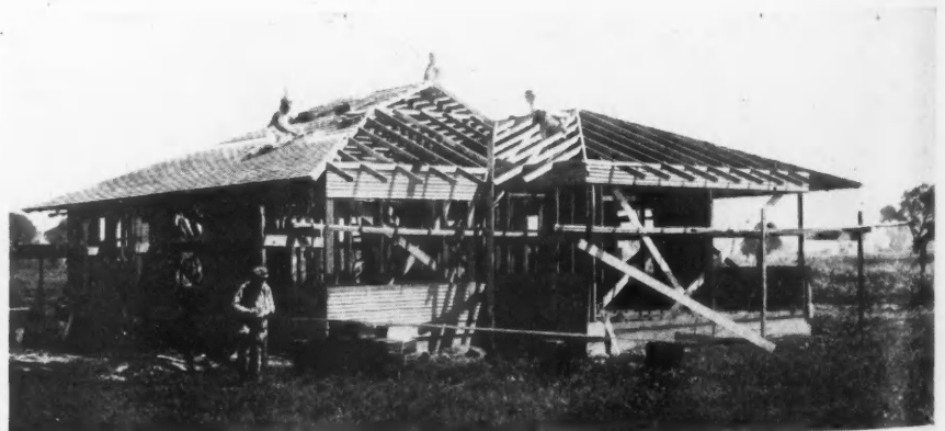
Bungalow Farm Home Under Construction in the Durham Colony, California.
