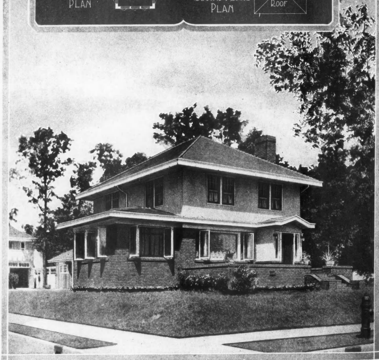
S IX-ROOM STUCCO HOUSE. Stucco homes are popular. Here is a design for a stucco house with a face brick porch that is a beauty. The dimensions of the house are 36 by 28 feet, exclusive of the porch projection. The living room, 13 feet, 6 inches by 26 feet, is extraordinarily large, and so is the dining room, 20 by 13 feet. The good-sized sun parlor, the sleeping porch on the second floor and the arrangement of the rooms take this design out of the "ordinary" class. An additional feature is the garage adjoining.
