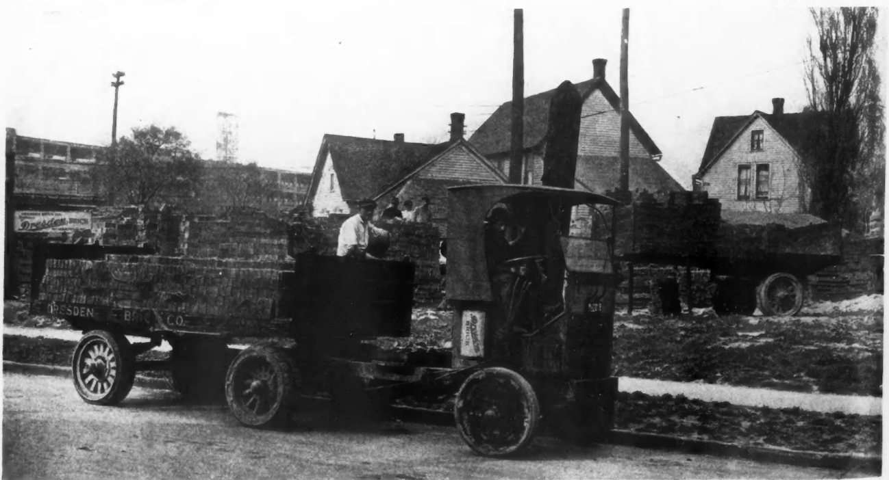
An Extra Semi-trailer Keeps the Motor Truck in Operation Continuously. The Dresden Brick Co. Has Two Trailers. While the Truck Is Taking One to the Building Job, the Other Is Being Loaded. Attaching and Detaching the Trailer Requires Only a Few Minutes. This "Packard" Truck and Semi-Trailer Is Carrying Eight Tons of Brick.
