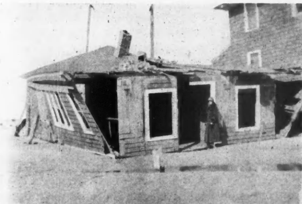
Photo 2. What Remained of a Bungalow that Was Set on Wood Piers.
