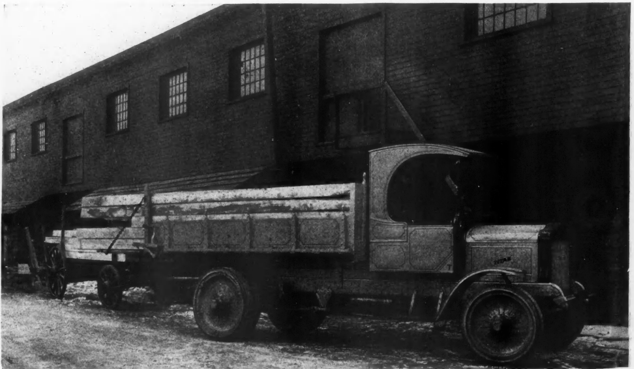
Heavy Foundation Timbers are Awkward to Transport, But the Modern Heavy Duty Motor Truck Has Successfully Solved the Problem. Here is a "Titan" Carrying a Big Load of Timbers Out of the Yard to the Job.
