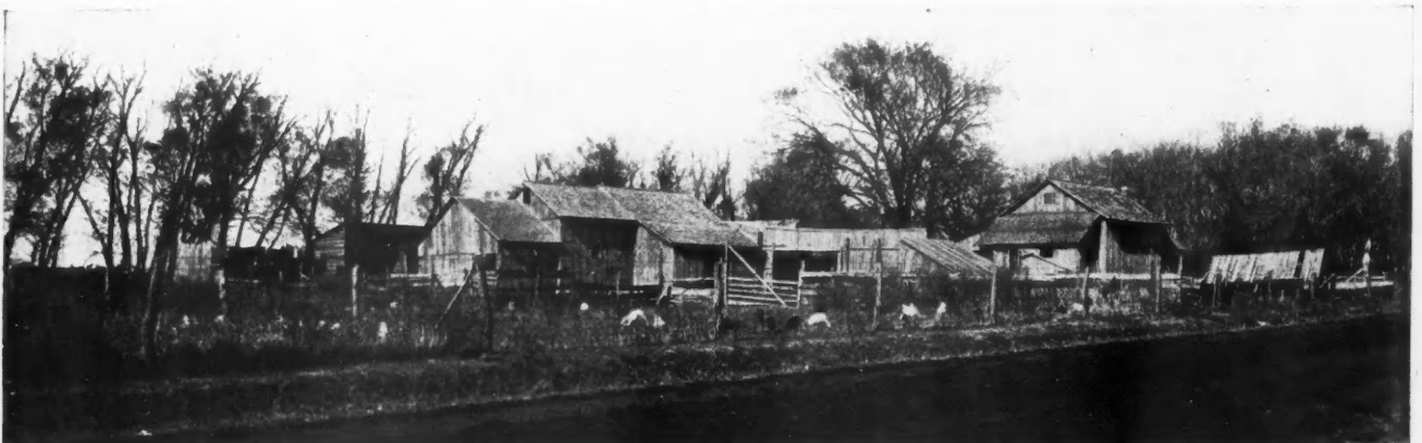
Buildings Like This Have No Place on the Modern Farm. They Are Too Expensive When One Considers What They Allow the Elements to Do to Crops, and Livestock.
