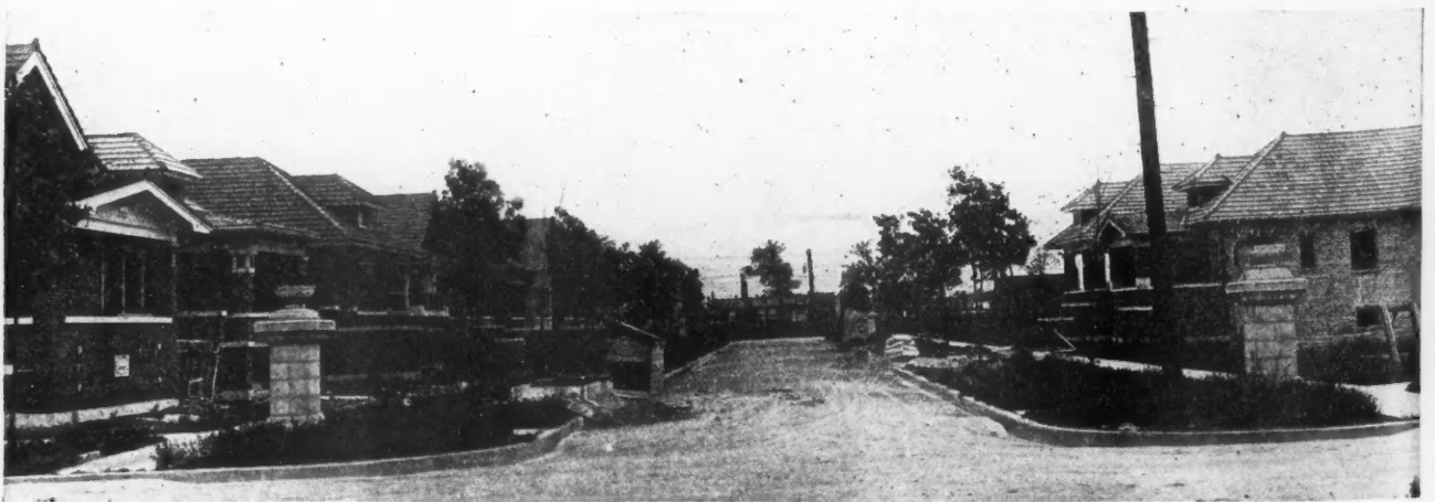
Building Projects Such as This Are Numerous Now that Construction Work Is On In Earnest.
