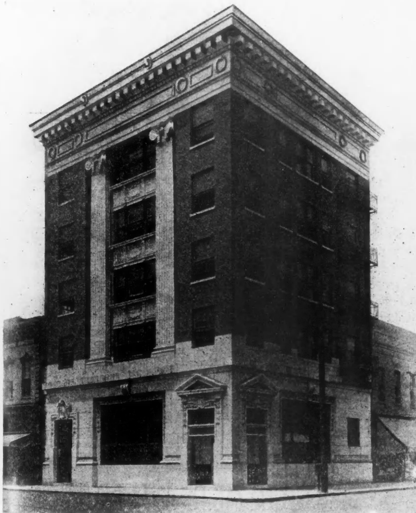
The New Home of the Bank of Edwardsville, Edwardsville, Ill. The Extensive Use of Terra Cotta, Coupled With Face Brick, Make This a Most Attractive and Impressive Building. Two Features a Bank Demands. The Building Is Five Stories High, the First Floor Being Occupied by the Bank and the Upper Floors Divided Into Offices. The Dimensions Are 52 Feet, 2 Inches, by 49 Feet, 3 Inches. Structural Steel Construction Was Used.
