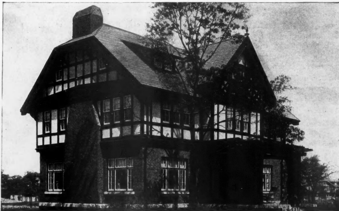
Roof covered with Ambler Asbestos Shingles (Century Brand)—American method. Upper sidewalls covered with Ambler Asbestos Building Lumber—Half-timber effect.
