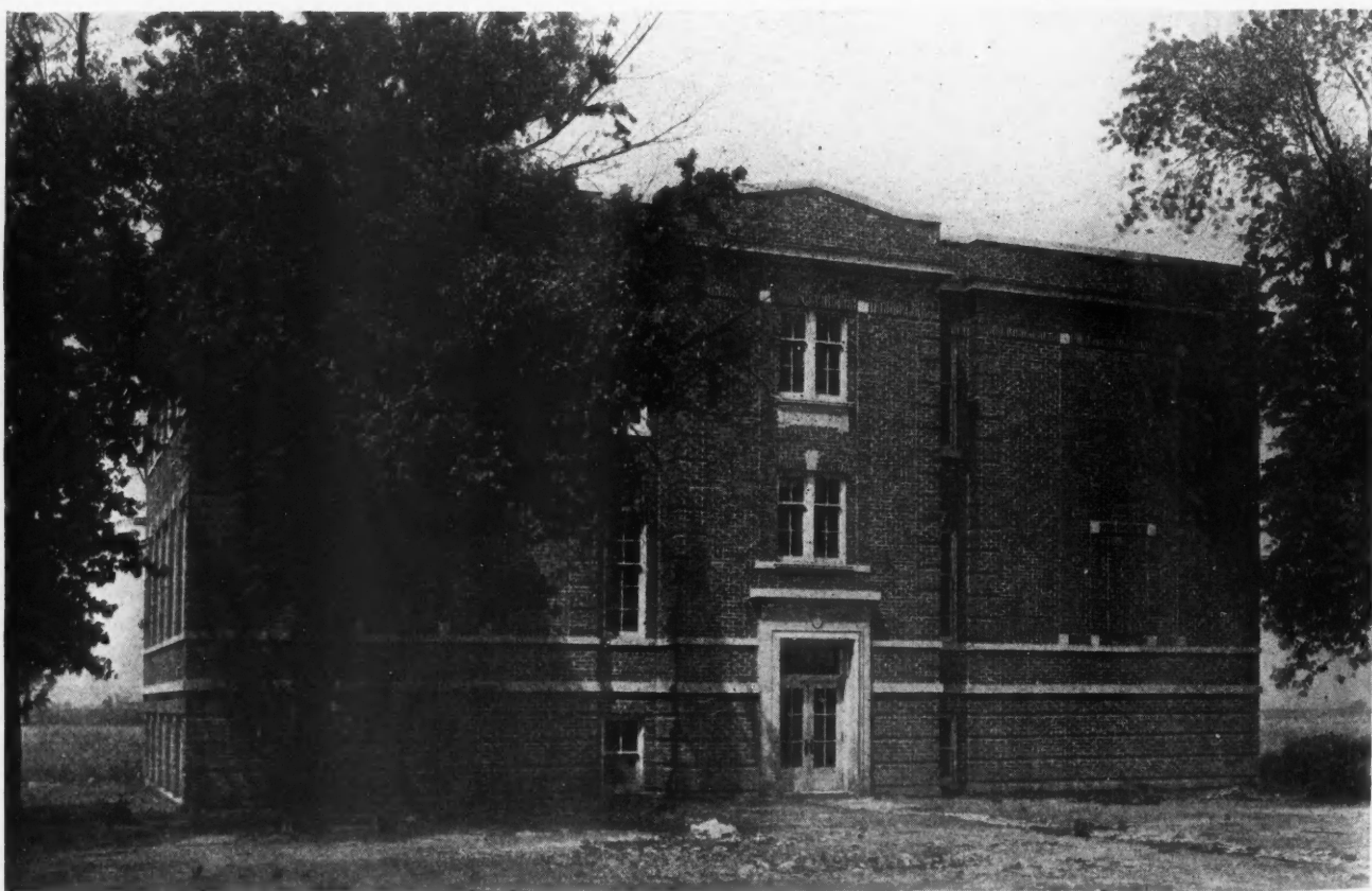
MODERN TWO-STORY, FOUR-ROOM GRADE SCHOOL BUILDING. The dimensions of the building are 79 by 34 feet. The floor plans show how well the rooms are laid out to provide proper light and ventilation. This is an excellent design for school buildings in rural districts and the smaller towns and cities. G. W. Ashby, Chicago, Architect.
