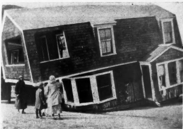
Photo 1. Shows Washed Away Pier Foundation and the House Was Left in this Position.
