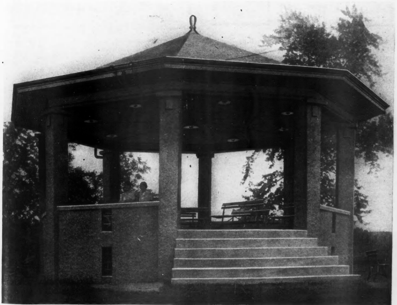
Design for a Rough Finished Concrete Band Stand, Such as Are in Demand for the Parks in All Cities, Large and Small. The Floor Plan and Cross-Section Show the Construction Methods Used.
