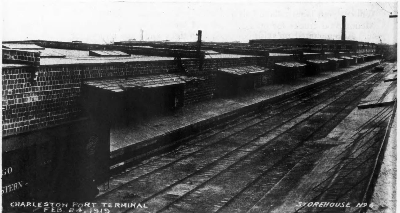
Fig. 8. Another View of the Charleston Port Terminal, Showing the Freight Receiving Platform. Note how the building is divided at intervals by fire walls which extend above the roof.
