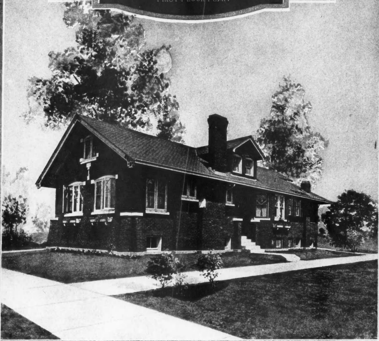
B EAUTIFUL BRICK BUNGALOW. Here is a brick bungalow of five rooms, with a large sun parlor and well-lighted attic space. This house is designed for a narrow lot, or for the owner who wants a wide expanse of side yard. Its dimensions are 25 feet, 10 inches by 56 feet, 10 inches. The large living room, 13 by 24 feet, with the sun parlor, 22 feet, 6 inches by 9 feet, 6 inches, opening off it and connected by glazed doors, is a feature. Here is a home that the owner can be proud of and will be a credit to the builder, as it is not only attractive, but contains every convenience.
