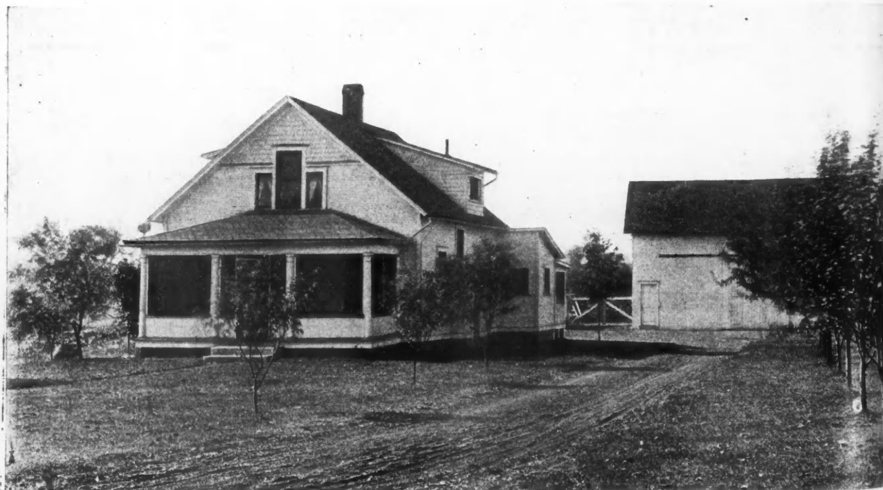
Farm Home of E. S. Wells, Near Salem, Ohio. Mr. Wells Has His Home Equipped with Electric Light and Running Water. The Electric Light System Furnishes the Power to Run the Small Water Plant Shown Above.
