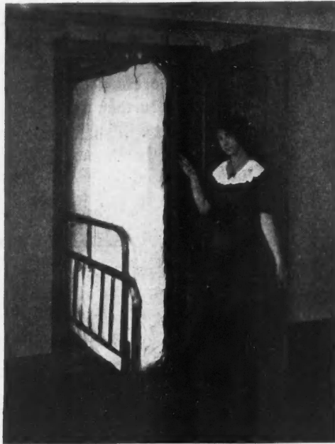
The Space-Saving Bed that Is Hinged to the Door Casing and Swings Into the Closet.
