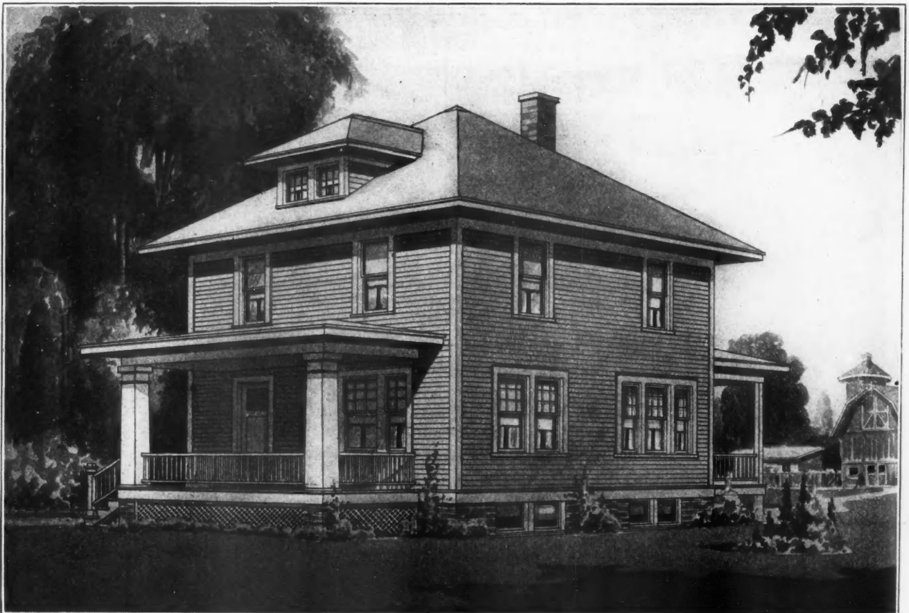
Perspective of a Six-Room Farm Home of Standard Frame Construction. The Size, 30 by 34 feet, and the Room Arrangement Make It a Good Design for the Average Farm. It is Modern in Every Respect and Will Make an Attractive Home.
