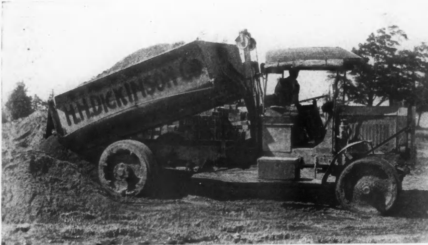
The H. H. Dickinson Builders' Supply Co. Use Seven Big "Packard" Trucks to Transport Materials from Its Five Yards in Detroit.
