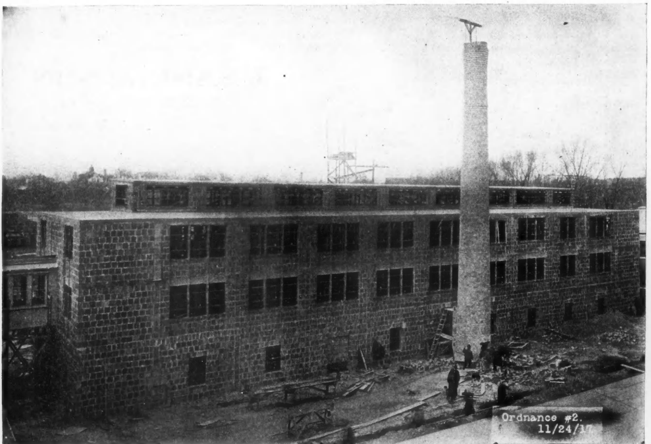
Fig. 1. Ordnance Department Building, Washington, D. C. An excellent model for the small all-fireproof factory building.
