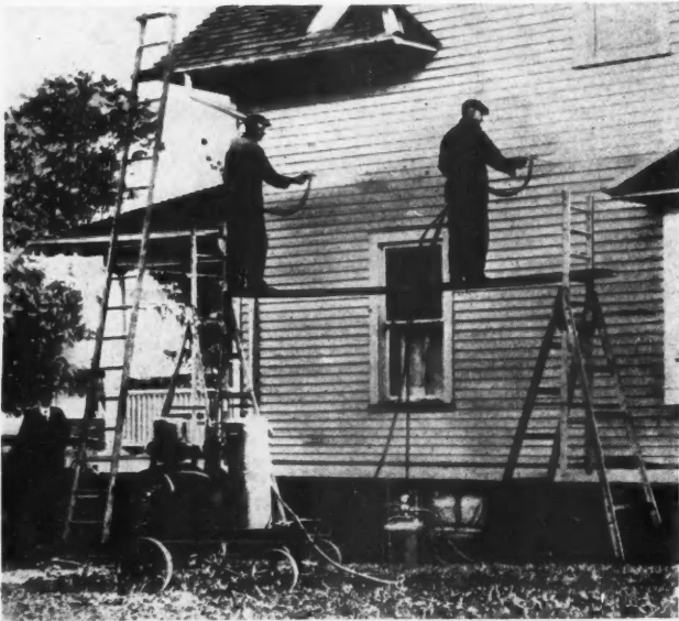
It Takes Only a Few Hours to Paint a House by the Air-Brush Method.
