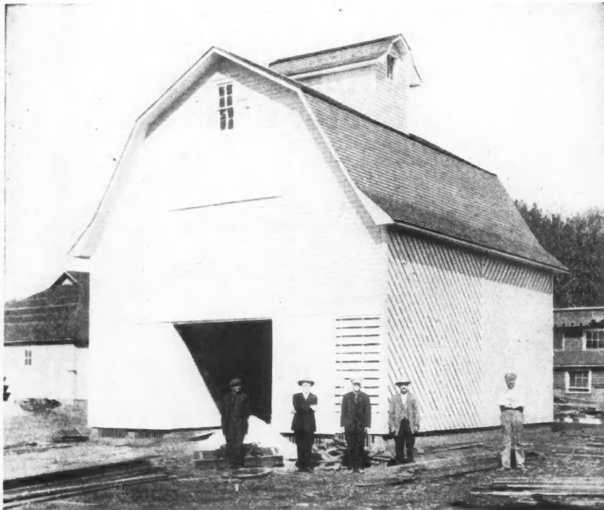
Here is a Fine Corn Crib and Granary Erected by Albert Werner at Dewese, Neb. Mr. Werner and His Crew Are Shown in the Foreground.
