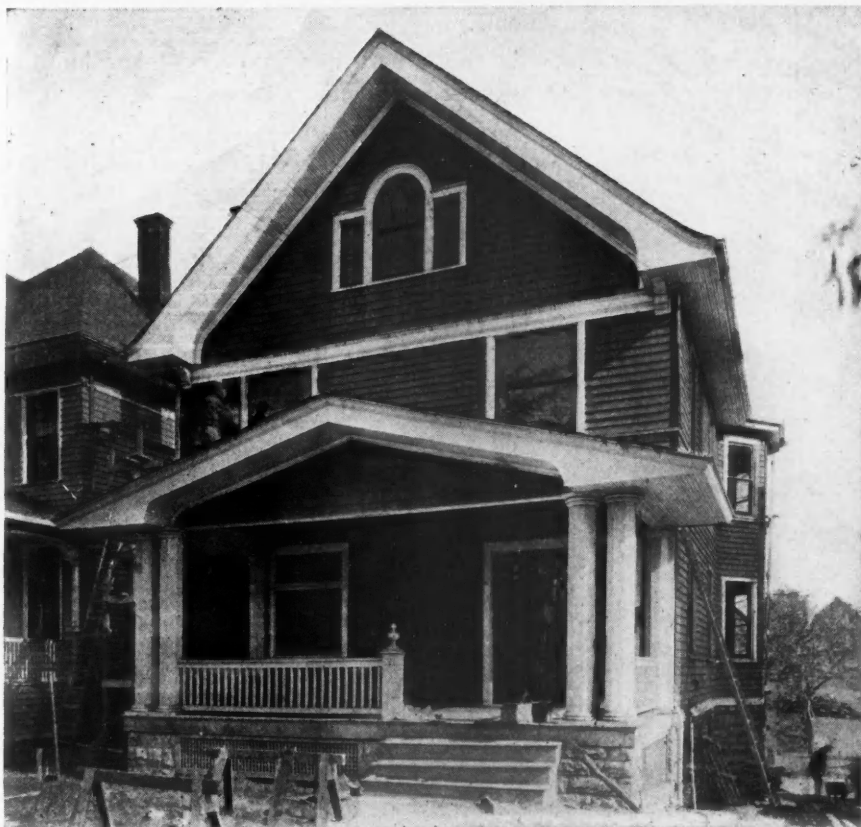
The Home of J. D. Hodson, Cincinnati, Before It Was Overcoated with Stucco Over Metal Lath. The Siding Was Not Removed, the Lath Being Nailed to It and the Stucco Applied by Means of a Special Machine.
