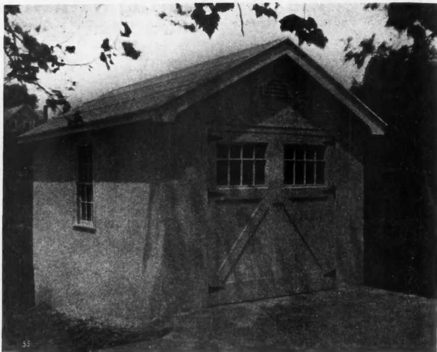
The Stucco Garage that Was Built in Connection with the Hodson Home. Metal Lath Was Nailed to the Sheathing and the Stucco Applied.
