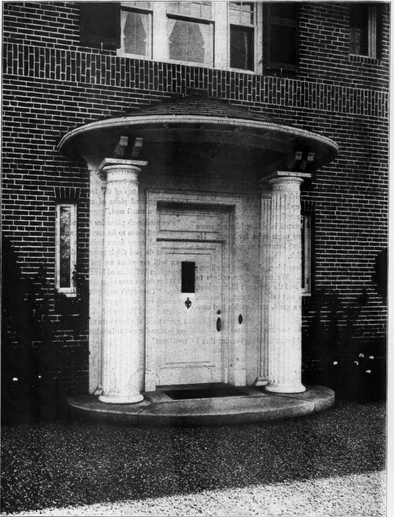
Detail of the Entrance and Porch of the George E. Smith Home, Philips Beach, Mass. This is a Fine Example of Colonial Style Brick Work. The Soldier Course Marking the Second Story is an Unusual Feature of the Brick Work.
