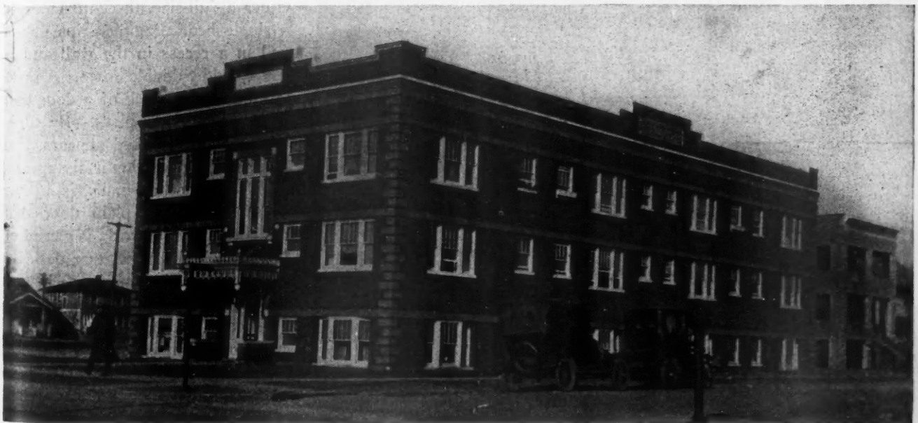
Perspective of the Modern Type of Apartment Building. This Building Contains Twenty-two Two-Room Apartments, Eight on Each of the Upper Floors and Six in the Half Basement. Thru the Use of Space-Saving Beds and by Eliminating the Dining Room Each of These Apartments Has the Efficiency Found in a Four-Room Apartment.
