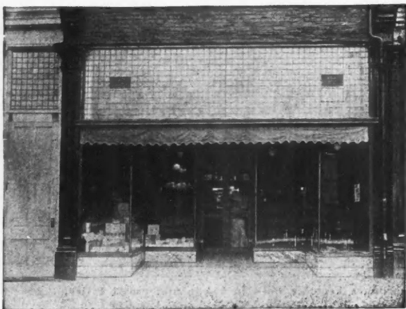
The Store Pictured Below After a New Front Was Installed. Converting Saloons, with Their Closed Fronts, Into Such Business Places as this Will Furnish Profitable Work for Contractors.
