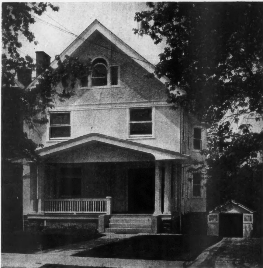
The Hodson Home After It Had Been Overcoated with Stucco. What an Improvement in Appearance the Stucco Made Is Shown by Comparing this and the Other Illustration on this Page.
