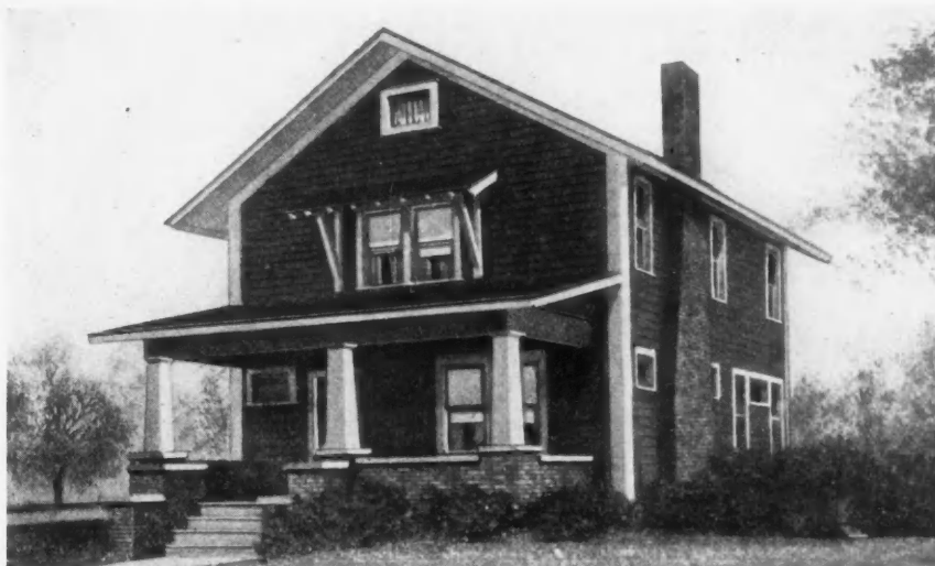
Two-Story Cottage with Good Lines. Size 22 by 26 feet. This is the type of home for department managers and foremen. It is modern in every particular
