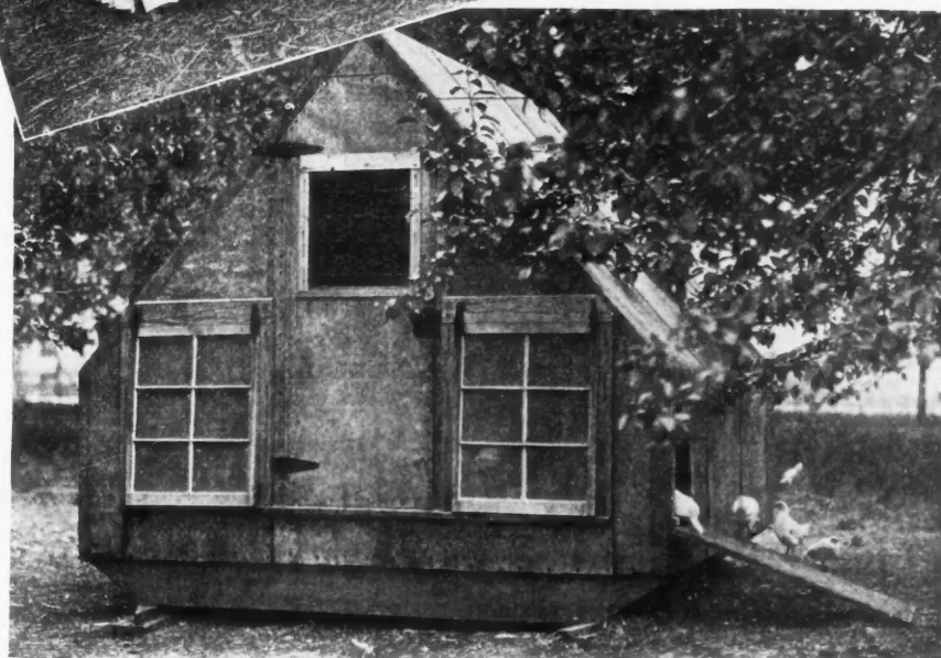
An Inexpensive Brooder House Made of Rough Lumber and Covered with Tar Paper or Ready Roofing. This Little Poultry House is Well Lighted and Ventilated. The Heater is Gasoline Heated as Illustrated in the Two Upper Photos.
