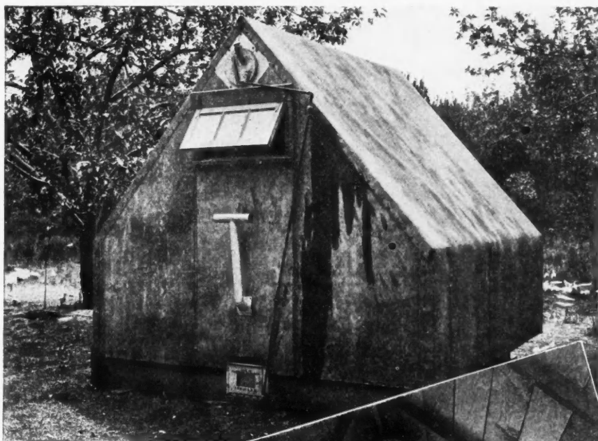
Brooder House Viewed From the Rear, Showing Fuel Storage Tank Piping and Vent for Gas Heater.
