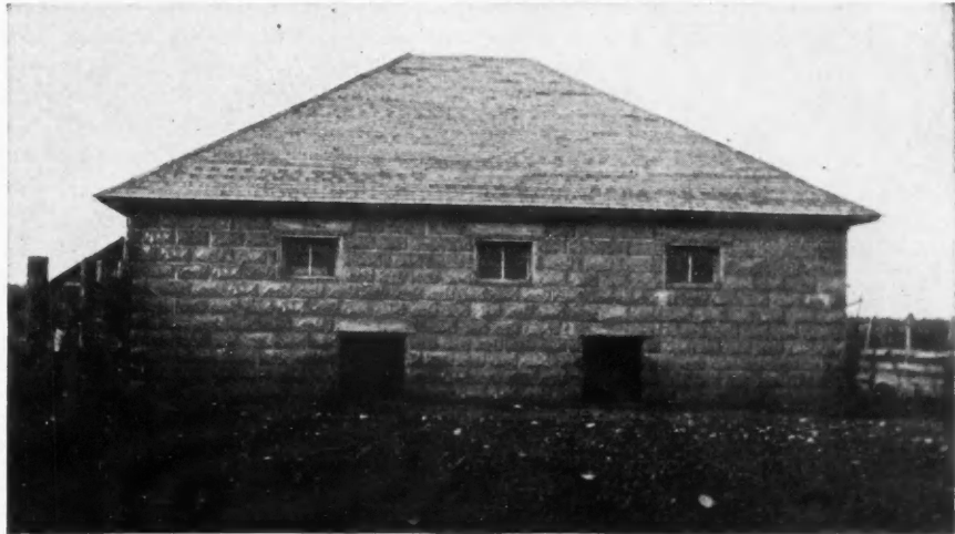
Hog House—Medusa Waterproofing used for facing Concrete Blocks
