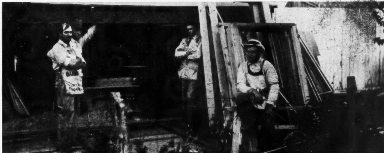
Wass & Budge, of Malad, Idaho, and Their Power Woodworking Establishment.
