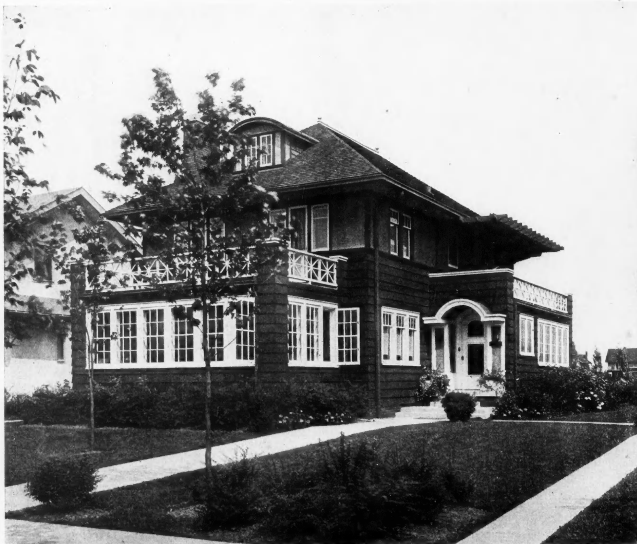
Modern Square-Type Sun-Parlor Dwelling Containing Eight Rooms. Complete Working Plans for This Dwelling are Presented on the Four Blueprint Pages Following.
