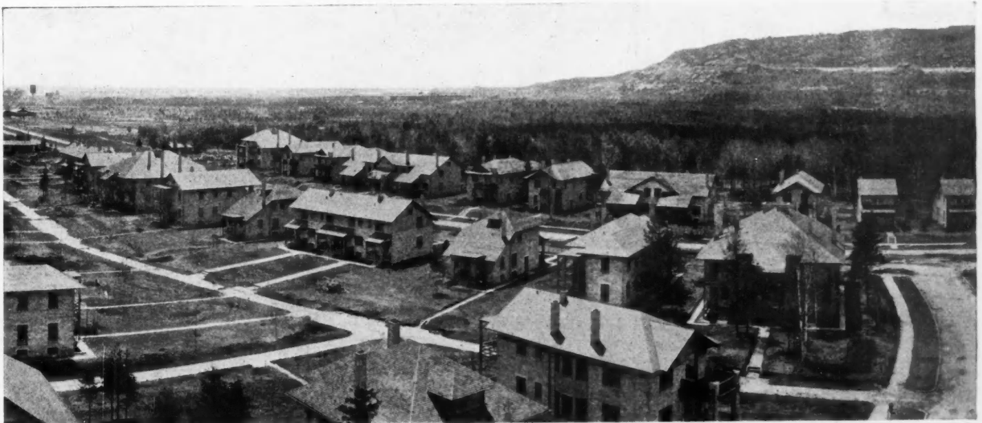
Carried Out by the Universal Portland Cement Company. All of These Buildings are of Concrete Block Construction.
