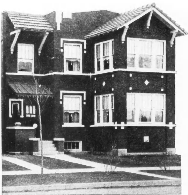
Newest Type Two-Flat Building with Large Sun Parlors. Building of Face Brick and White Terra Cotta Trim.
