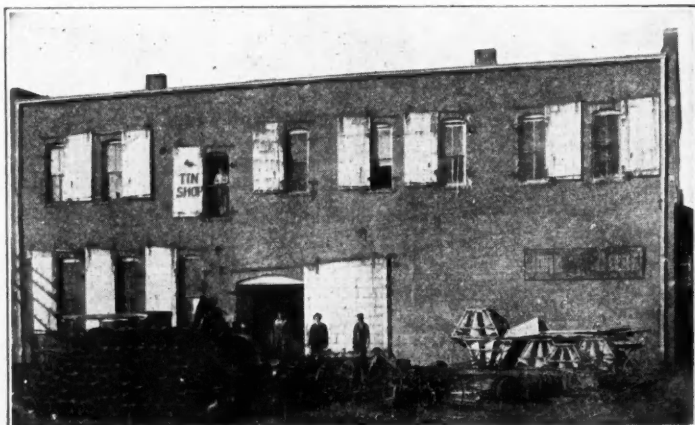
The Fire Door and Window Shutters Still in Good Shape and Giving Service Six Years After the Fire.
