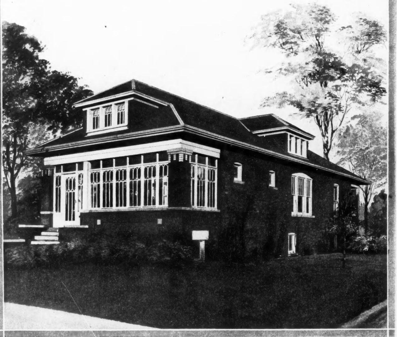
B BRICK COTTAGE WITH GLAZED-IN PORCH. Here is the popular city cottage. It is 24 feet wide to go on a 30-foot lot. The front porch is glazed in for the sun parlor. The connecting living room and dining room are pleasant apartments. The kitchen is conveniently located and the suite of two bedrooms and bath is well arranged for privacy.
