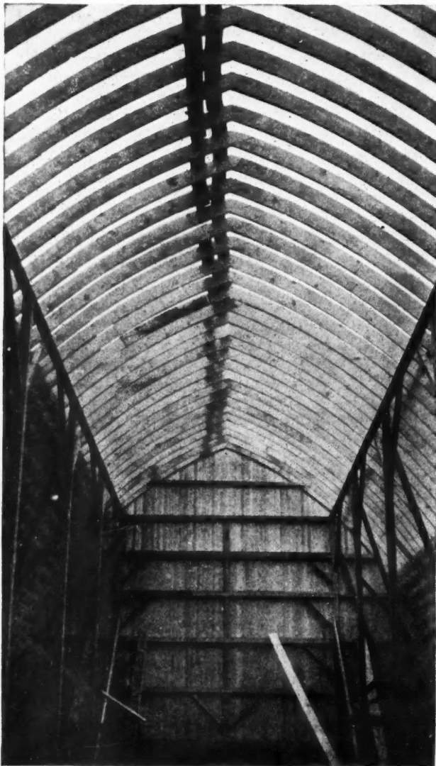
Interior of McPherson Gothic Roof Barn.
