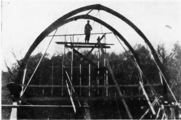
Raising the Roof Trusses.
