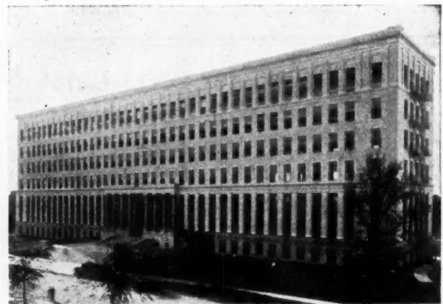
An Exceedingly Fine Example of Modern Office Building Construction Built for Permanence—The New Administration Building of the Willy's-Overland Company at Toledo, Ohio.
