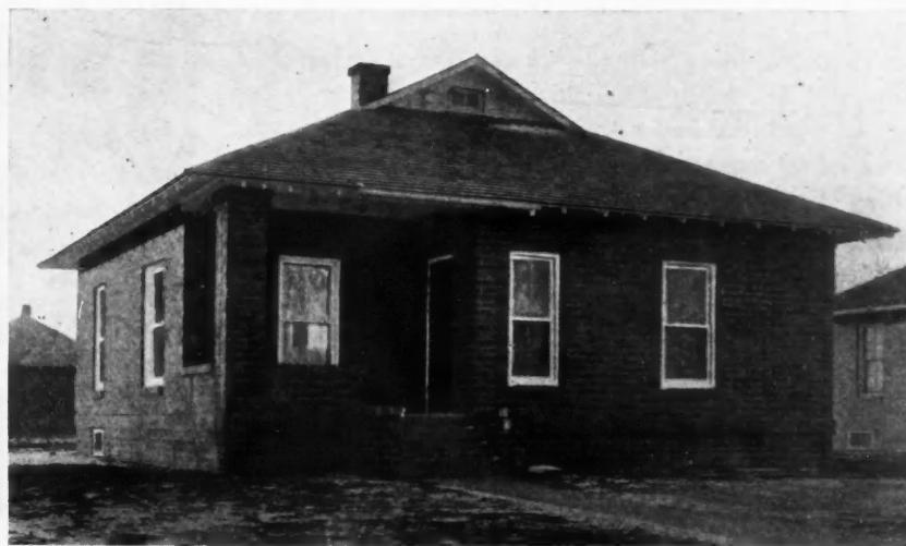
Small House of Structural Tile Which is Neat in Appearance and Especially Well Arranged. Cost, $1,350.00.
