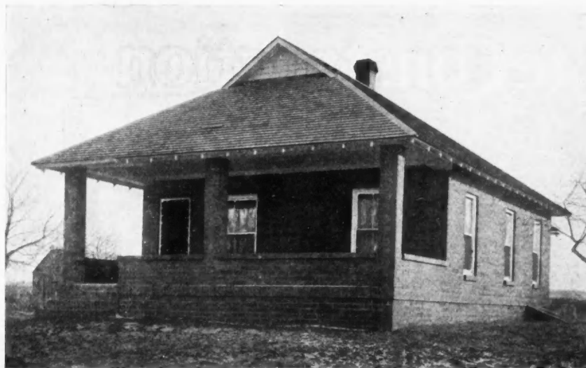
Five-Room Cottage Built of Self-Facing Structural Tile. Cost, $1,000.00
