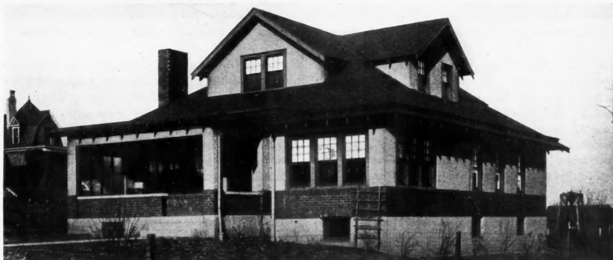
Attractive Bungalow with Poured Concrete Walls, Stuccoed Over for Finishing Coat. The Face Brick Veneer Course is an Interesting Detail.
