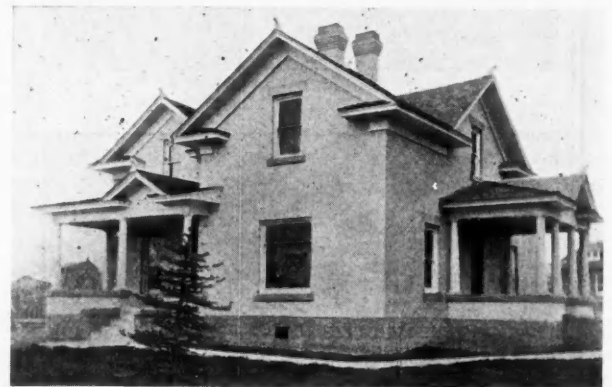
House of Light Buff Pressed Brick, Built at Fountain Green, Utah, for Thomas H. Cook, by J. E. Sorensen.
