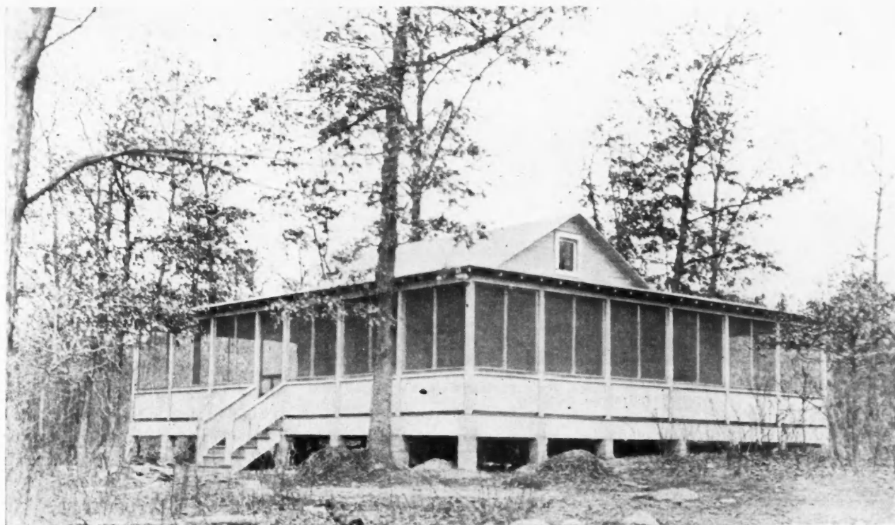
Cottage Built by Edwin L. Bradley Along Fox River Above St. Charles, Illinois. Notice the Large Porch Enclosed with Fine-Mesh Wire Cloth Screens. House Sits on Concrete Piers Placed 8 Feet Apart.
