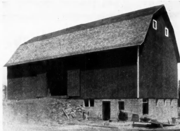
The Finished Barn, Which is the First, But Probably Not the Last Plank Frame Barn in the Vicinity of Fairmont, Minn.
