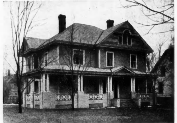
Residence of J. F. Ryan, Truro, N. S., Canada, Plans and Specifications of Which Were Prepared by George J. Mosher.
