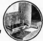
This shows sliding pivot hinge in position on top edge of sash.
