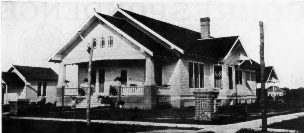
The Beautiful Residence of S. W. Huddleston, Auditor for the Alamo Lumber Company, at Cuero, Texas. This House is a Good Example of a Well Balanced One-Story Gable Roof Residence.
