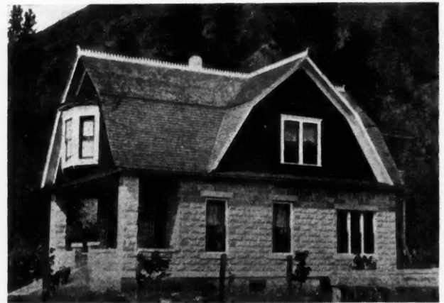
O. P. Decker, Kooskia, Idaho, writes regarding this concrete house: "We consider it ideal for all kinds of weather. It is very easy to heat and is very cool in the hottest weather. It is a veneered house."
