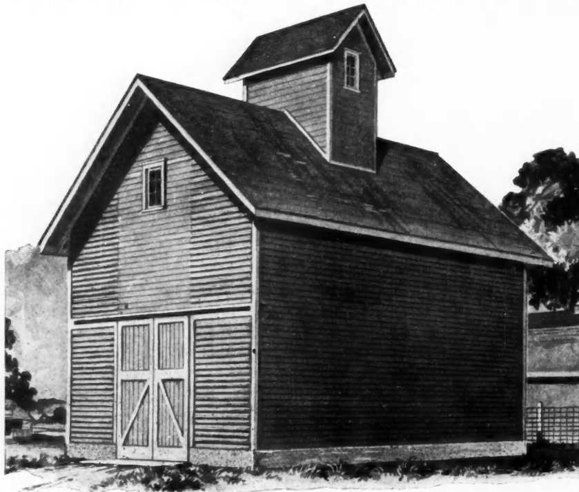
Fig. 1A. A Modern Two-Story Corn Crib and Granary.
