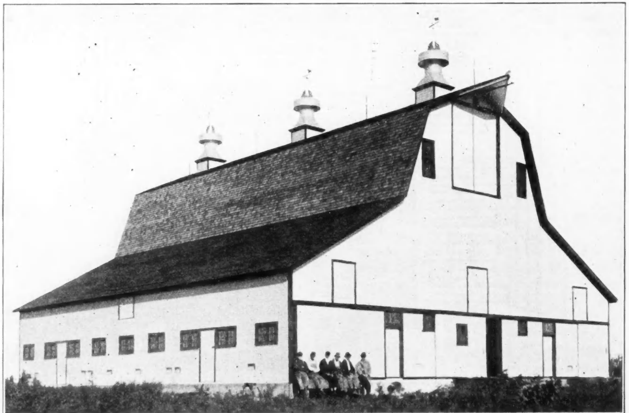
General Purpose Barn Costing About $4,000 Built by Stolp and Trainor, Ellendale, N. D., for H. E. Heine. This Building Represents a Type of Barn Which These Contractors and Builders Have Found Very Popular in Their Vicinity.
