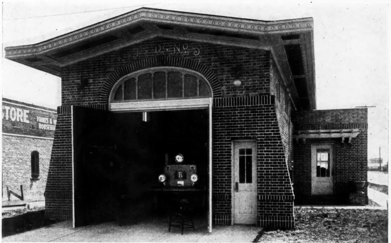
BEAUTIFUL BRICK FIRE ENGINE HOUSE. This fire engine house is distinctive, both because of its architectural design and because of the novel method of building up its face brick walls. It is situated at Richmond, California. Two kinds of face brick are used, the darker in color being laid in the lower walls with the lighter colored wall above. The color contrast between the header and stretcher brick in the upper wall is very effective.
