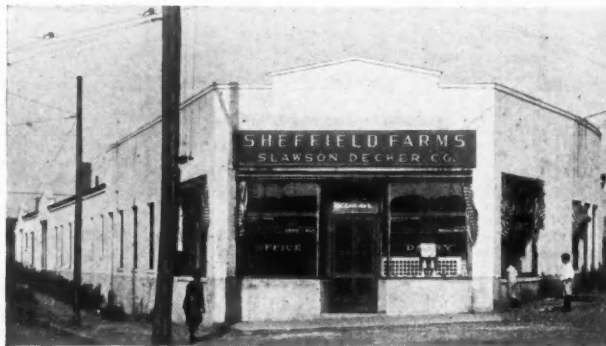
Milk Depot at Greenville, N. J., Constructed of Hollow Tile.
