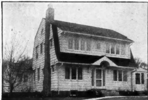
Architects, Whitmyer & Chaffee, Peoria, Ill., for Dr. T. C. Coggeshall, Henry, Ill. 24-inch "Dixie White" "CREO-DIPT" Stained Shingles on side walls. 16-inch moss green "CREO-DIPT" Stained Shingles on roof.
