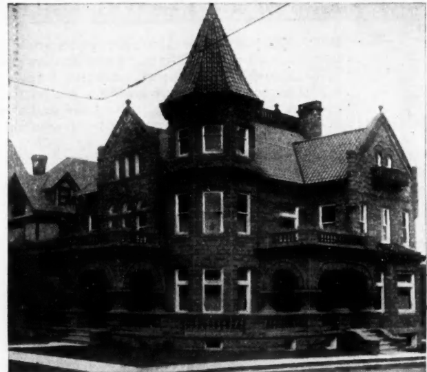
The Above Residence Completed. The Use of Stone, Tile and Concrete Makes It Practically Fireproof.
