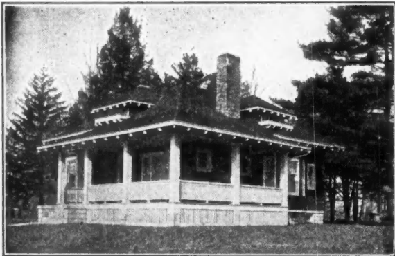
A Bungalow for Permanent Occupancy. Charles E. Anderson, designer, White Plains, N. Y. "The roof is covered with shingles dipped 10" in Cabot's Creosote Shingle Stains; the body is stained a rich brown with Cabot's Creosote Stain."
