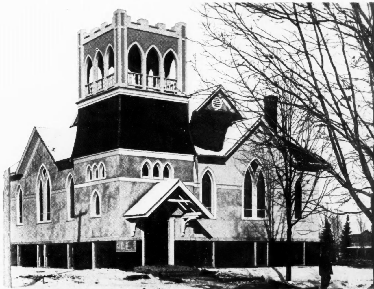
Methodist Church, First Prize Class C. Designed by D. A. Haines and Erected Under His Supervision at Mable, Minn.
