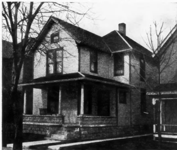
This Goes Perhaps a Trifle Too Far, tho the Owner is Satisfied. Three Rooms Upstairs are Warmed thru Ceiling Registers.
