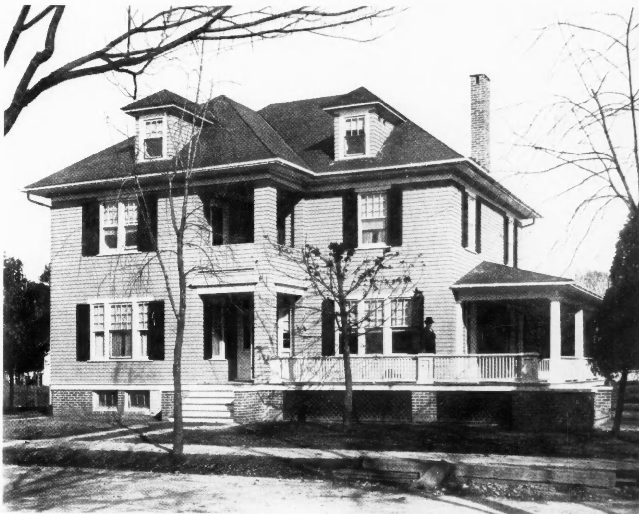
Eight-Room House Awarded First Prize for Residences, Class A. It Was Designed and Built by W. Twilley Malone, Contractor and Builder, of Allen, Md., for Mr. Frank Lano, at Princess-Anne, Md.
