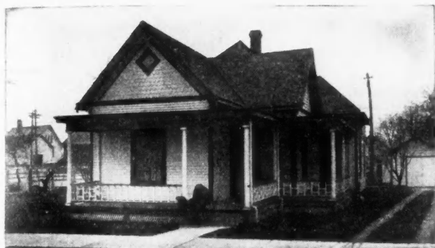
Six-Room Cottage Perfectly Heated by One Central Register. Range Sufficiently Heats Kitchen and Bath.
