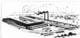
The most completely equipped Wall Board Plant in America
