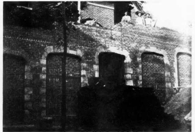
Brick Retaining Wall Decorated with Recessed Panels.
